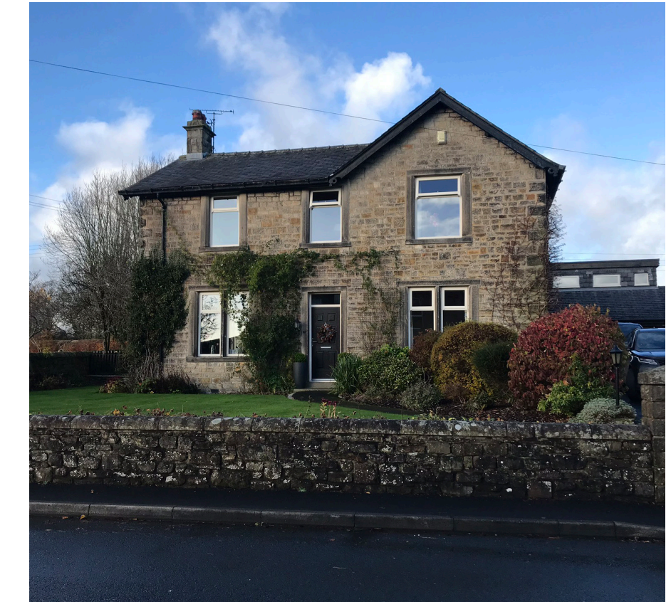
View of the front elevation from West Bradford Road.
