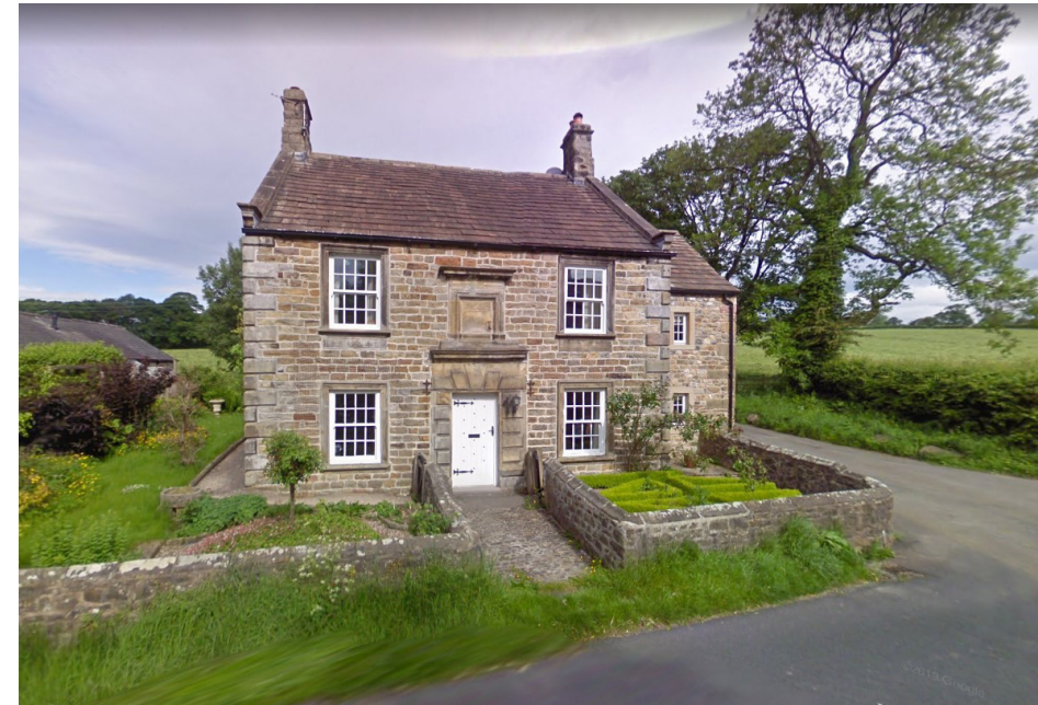
Locally listed property on West Bradford Road, Laneside, Grade II listed.
