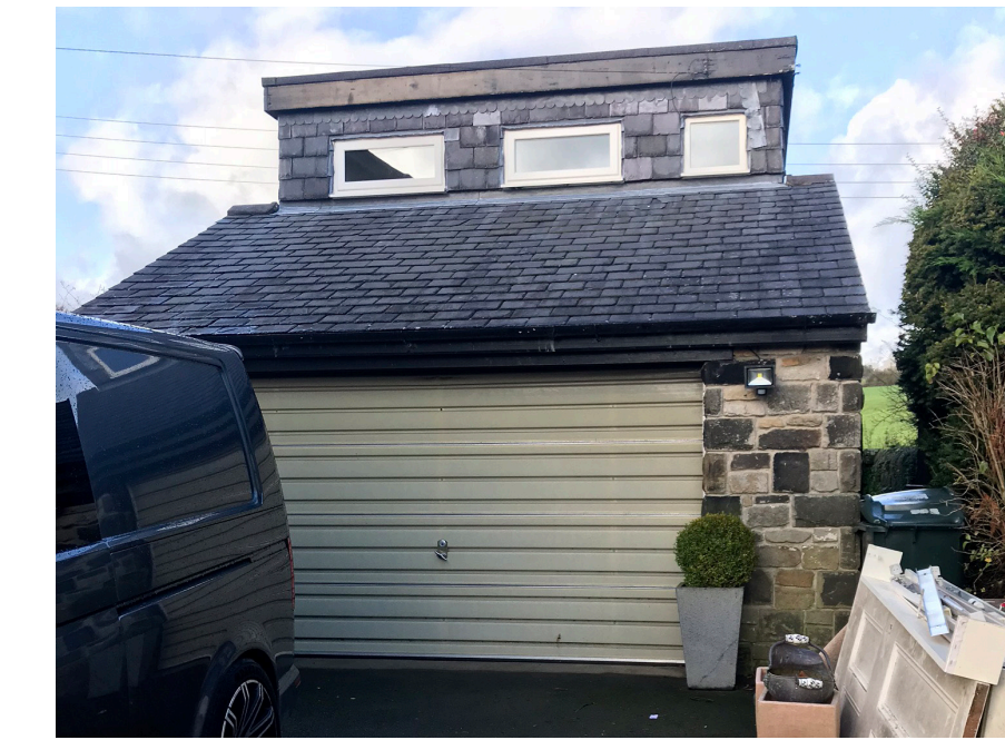
View of the 2-storey garage and home office.
