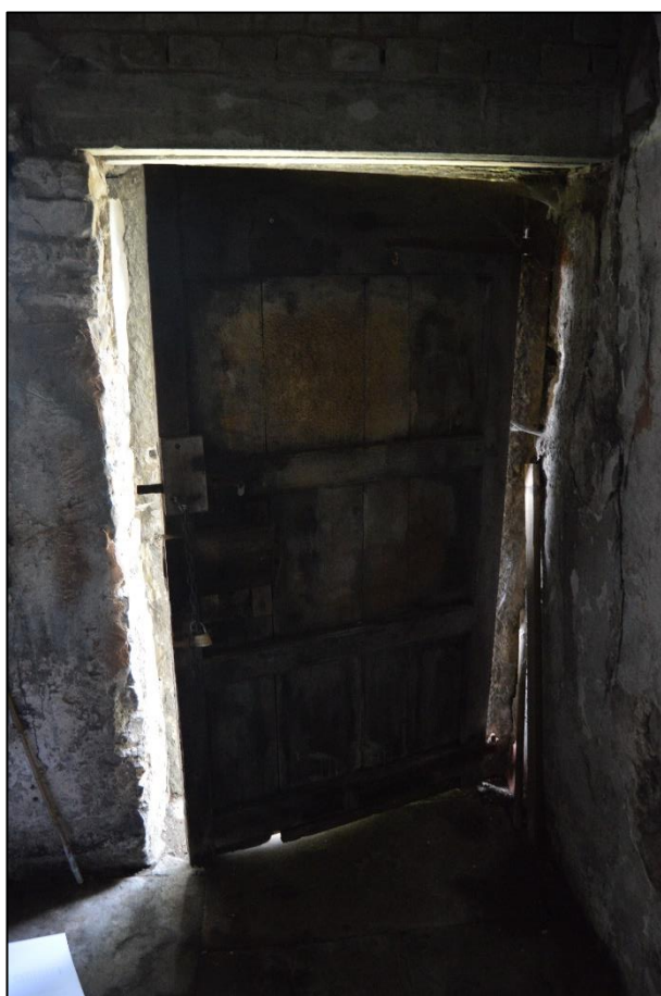
PL21: View of external plank and batten door to the ground floor living room.
