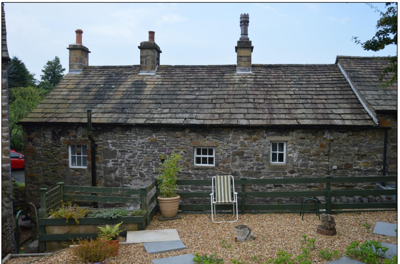
PL09: View of the rear North East facing elevation of No's 24 and 25 Brookside.
