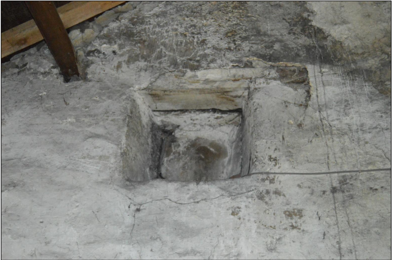
PL32: View of closed off former attic window present to the south west wall at first floor level.
