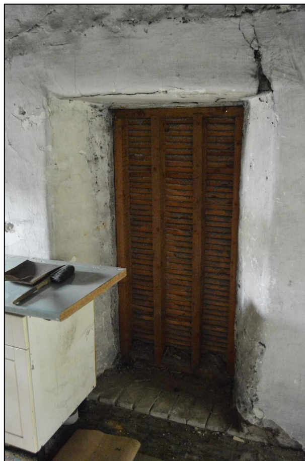
PL31: View of closed off opening present to the south east wall at first floor level.
