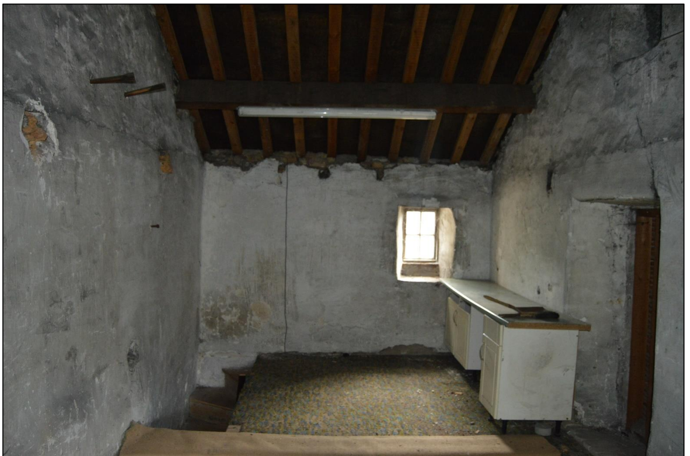
PL27: View north east at first floor level.
