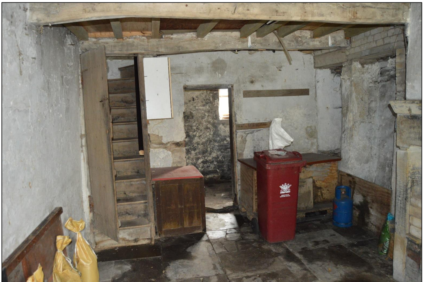
PL13: View north east within the ground floor living room.
