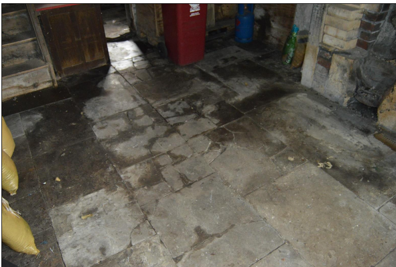
PL23: View of stone flag flooring to the ground floor living room.
