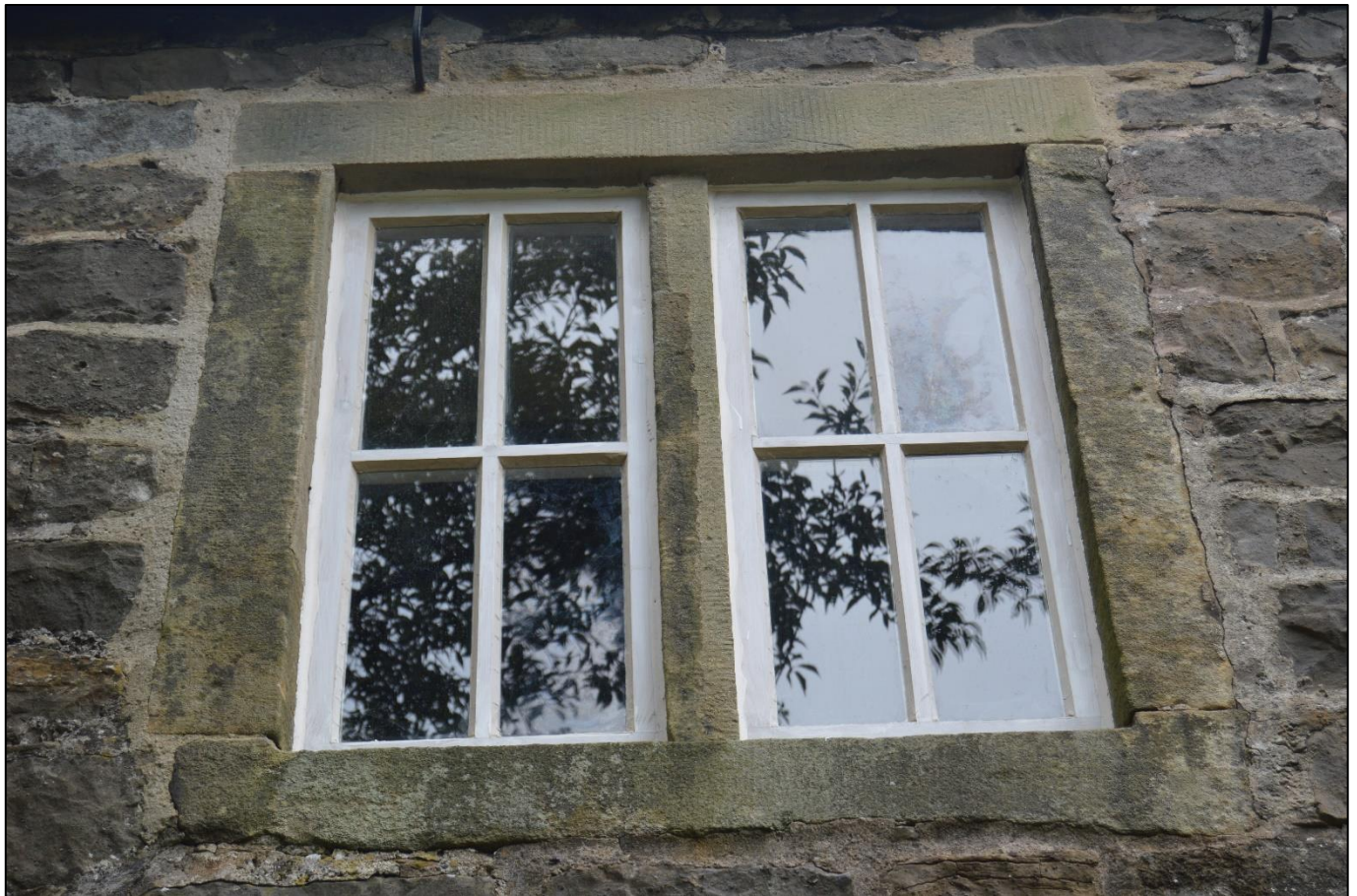
PL08: View of the first-floor window to the front elevation of No. 24 Brookside.
