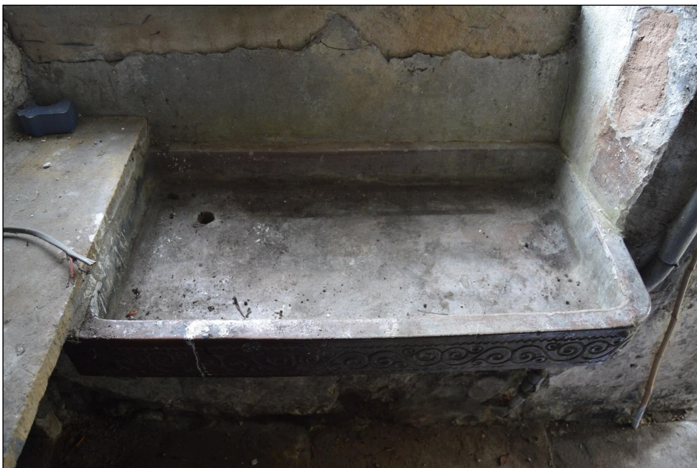
PL19: View of slop stone sink present to the ground floor lounge.
