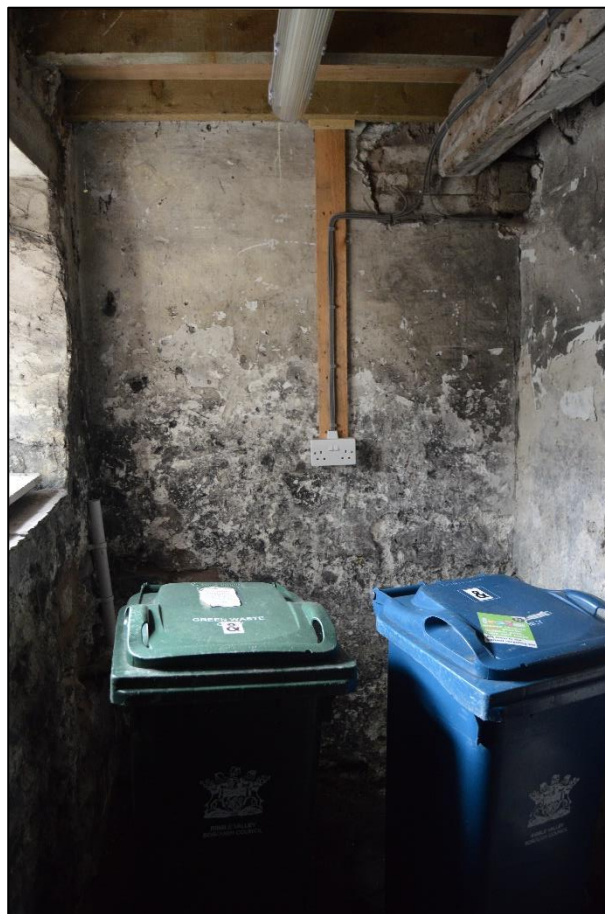
PL25: View south east within the rear ground floor unit.
