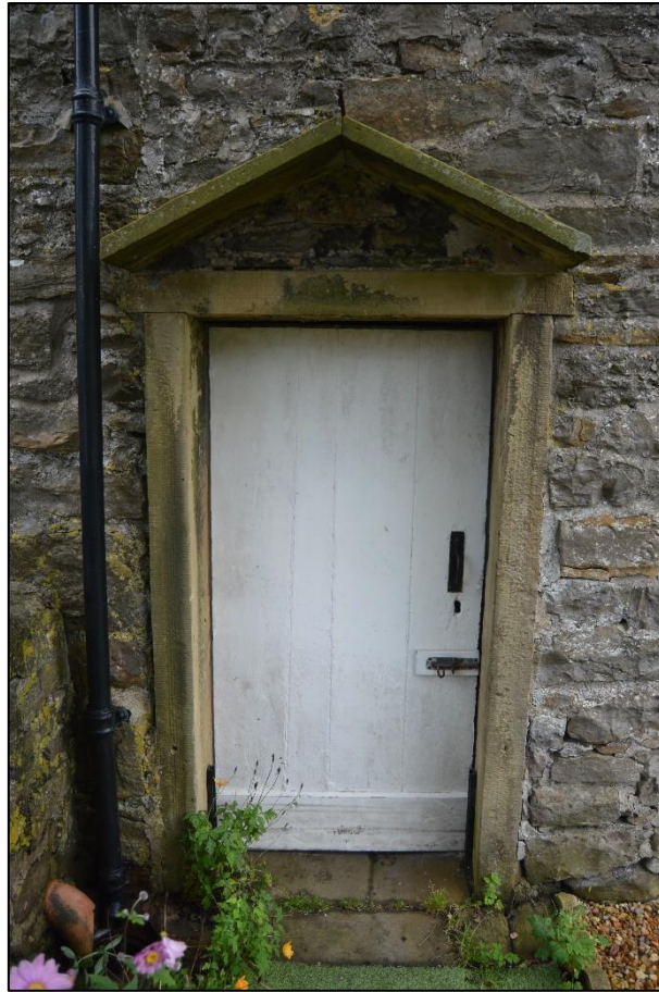
PL04: View of the front doorway to No. 24 Brookside.
