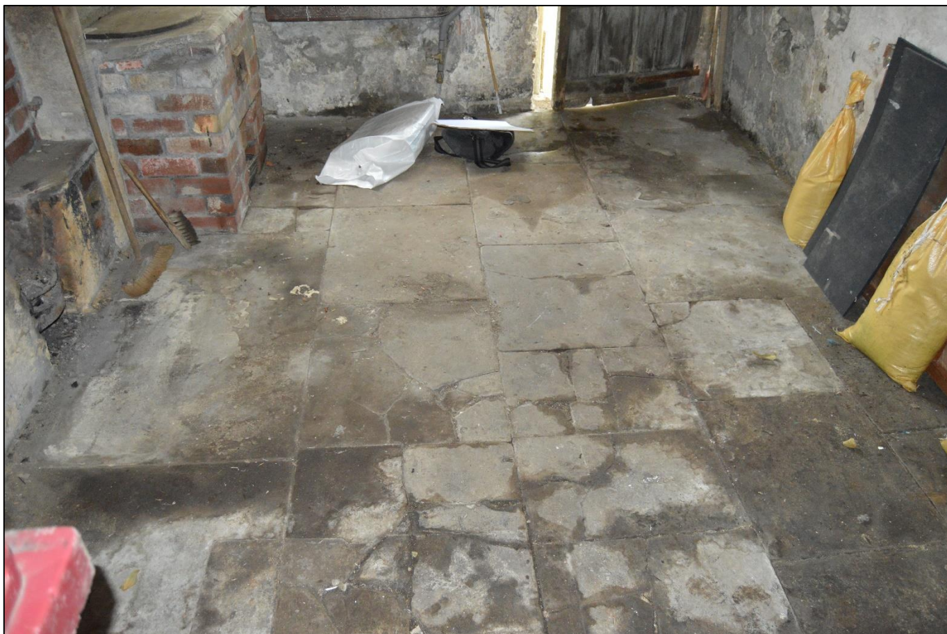
PL22: View of stone flag flooring to the ground floor living room.
