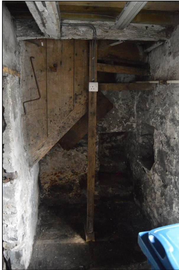
PL26: View south east within the rear ground floor unit.
