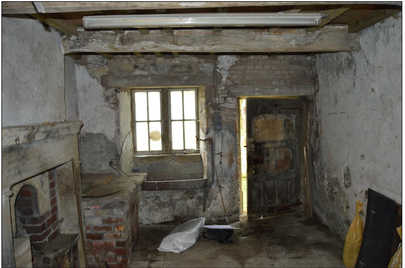
PL24: View south west within the ground floor living room.
