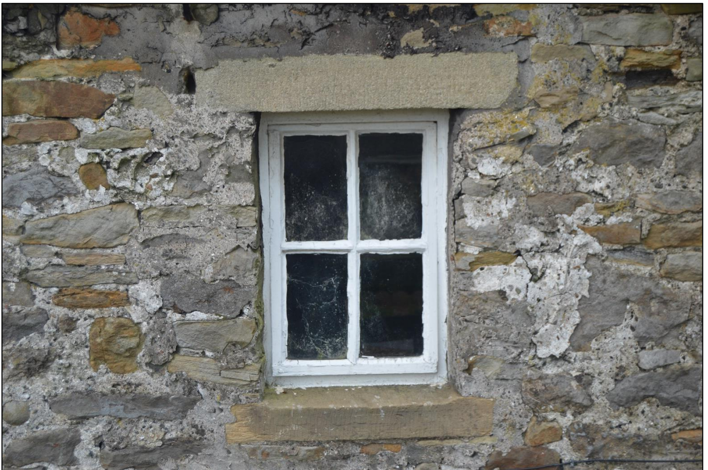
PL11: View of the rear first floor window to No.24 Brookside/
