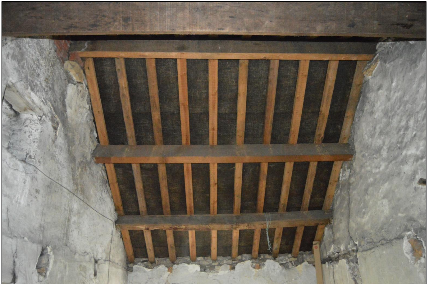
PL30: View of the roof structure to the south west roof slope.
