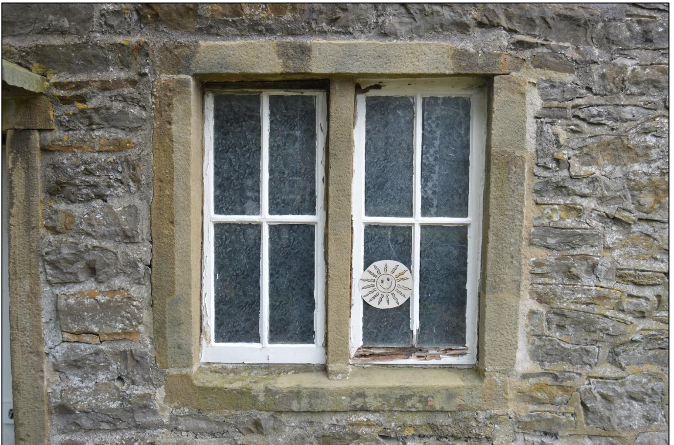
PL05: View of the ground floor window to the front elevation of No. 24 Brookside.
