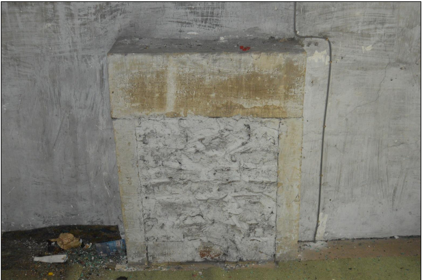
PL33: View of blocked up fireplace at first floor level.
