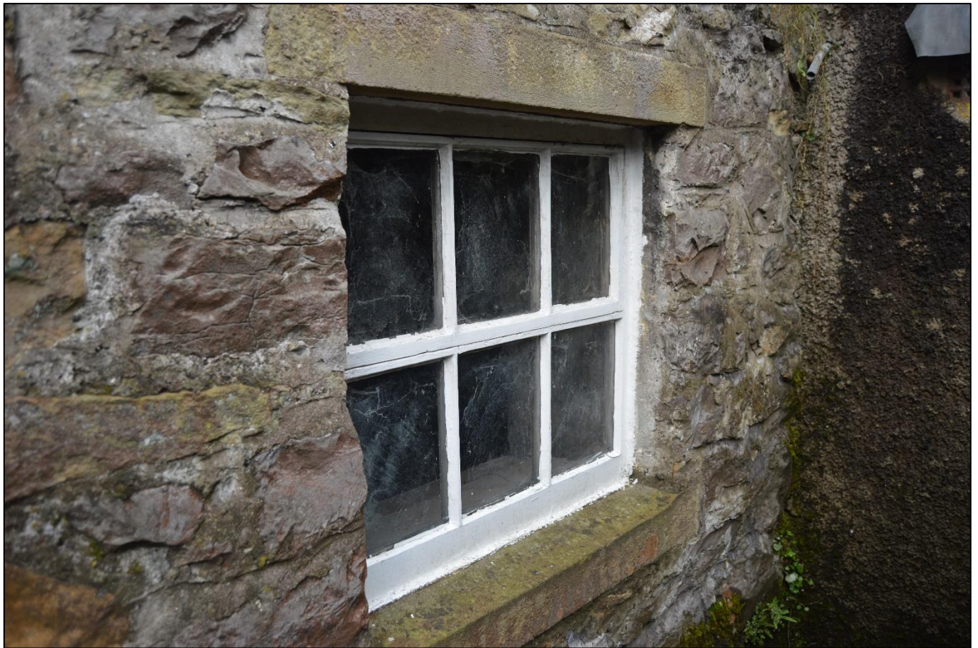
PL12: View of the rear ground floor window to No. 24 Brookside.
