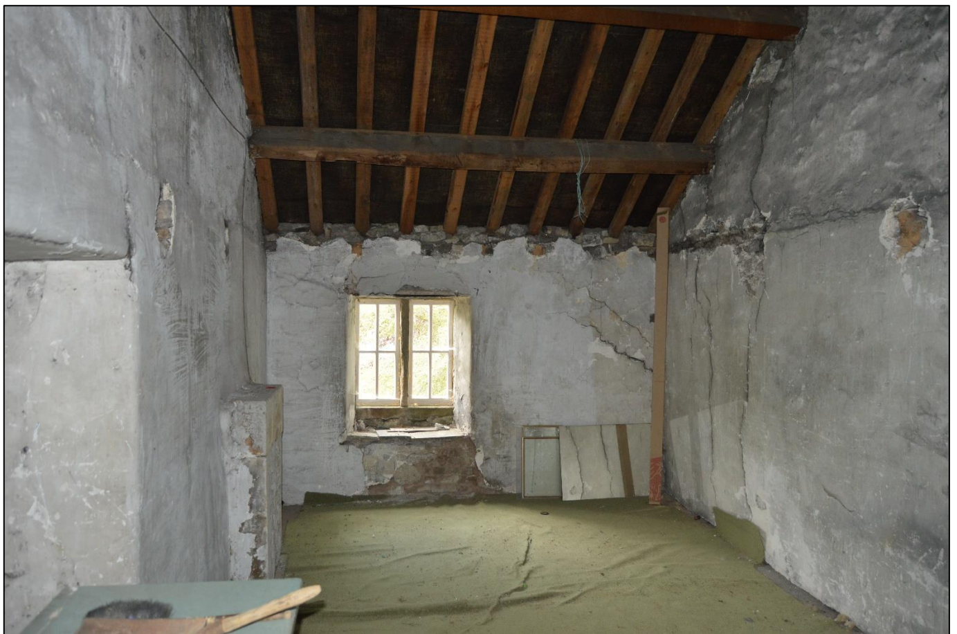
PL29: View south west at first floor level.
