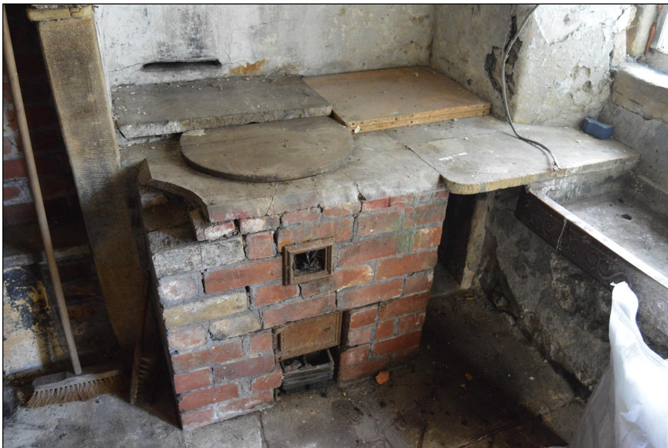
PL18: View of brick oven / stove to the ground floor living room.
