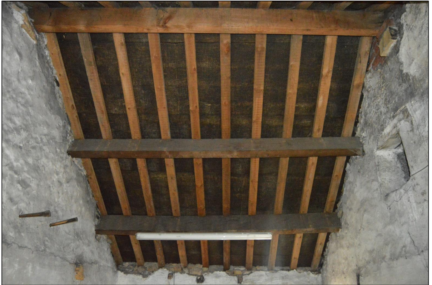
PL28: View of the roof structure to the north east roof slope.
