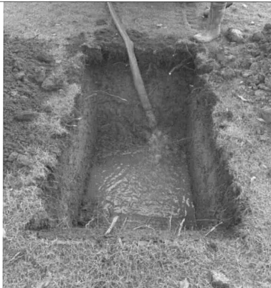
SA1 Surface Water Infiltration Test
