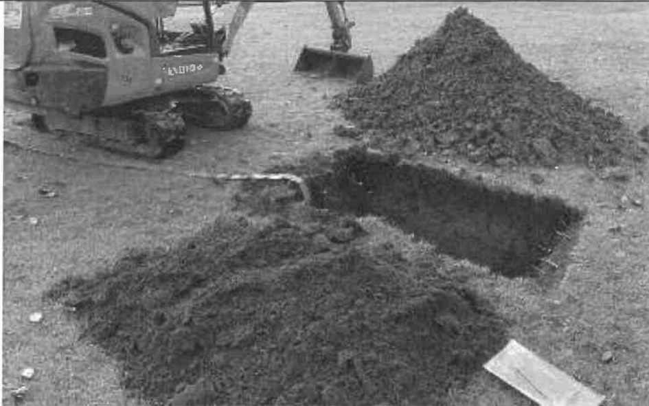
SA1 Surface Water Infiltration Test
