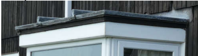
Bay window roof
