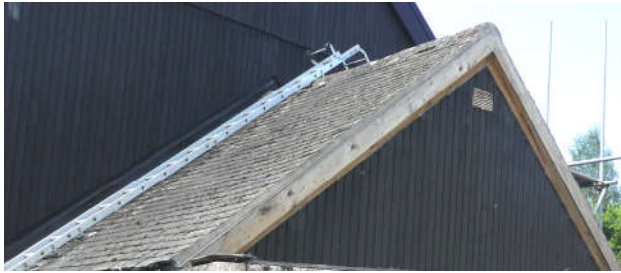
Single storey roof
