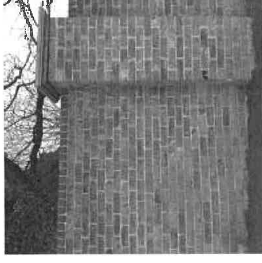
Brick screen wall as a noise mitigation measure
