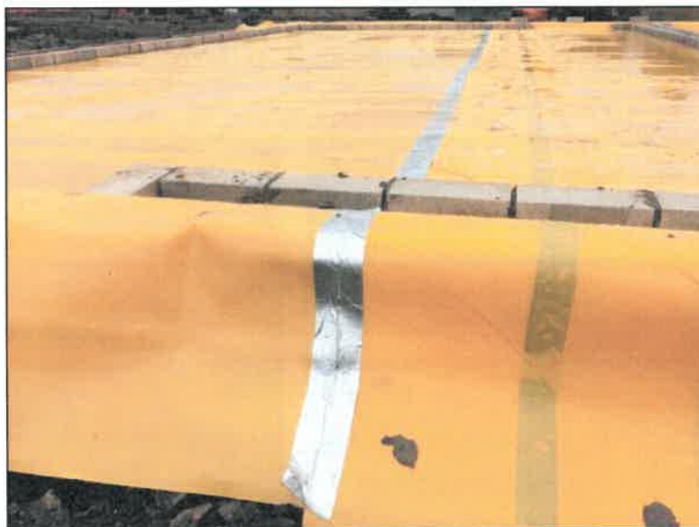
Photographs 20 and 21: Check >150mm overlaps of membranes and proprietary tapes placed and sealed with photographs taken
