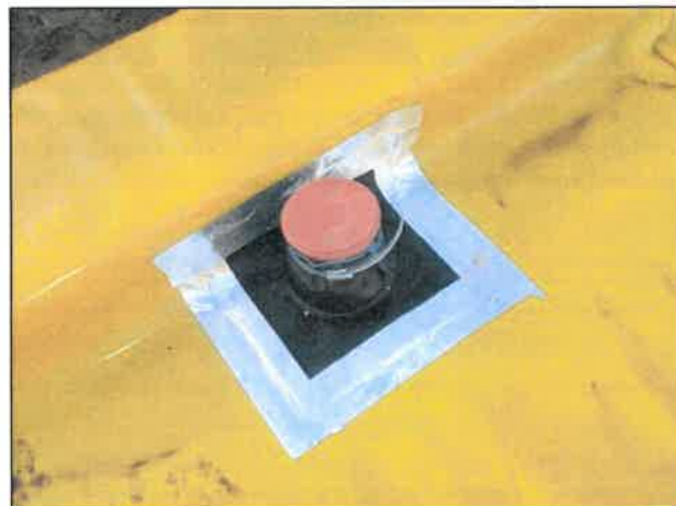
Photographs 22 and 23: Check tophat is sealed to membrane and pipework with tapes, and Jubilee clip
