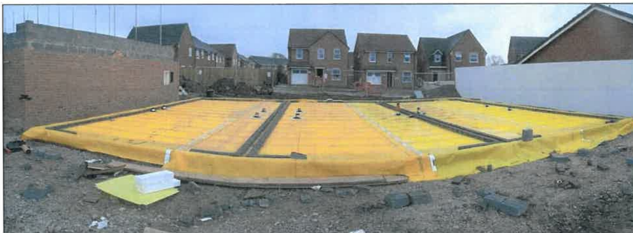
Photograph 19: Check general condition of membrane for punctures/tears etc – take panoramic photograph showing general condition
