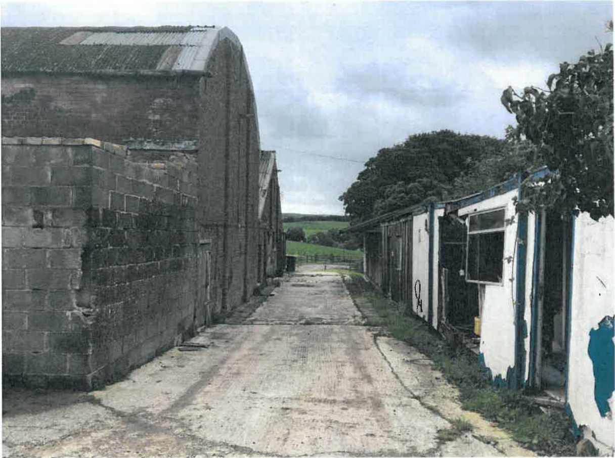
Photograph 5: Western elevation showing portacabins and sheds to be demolished.
