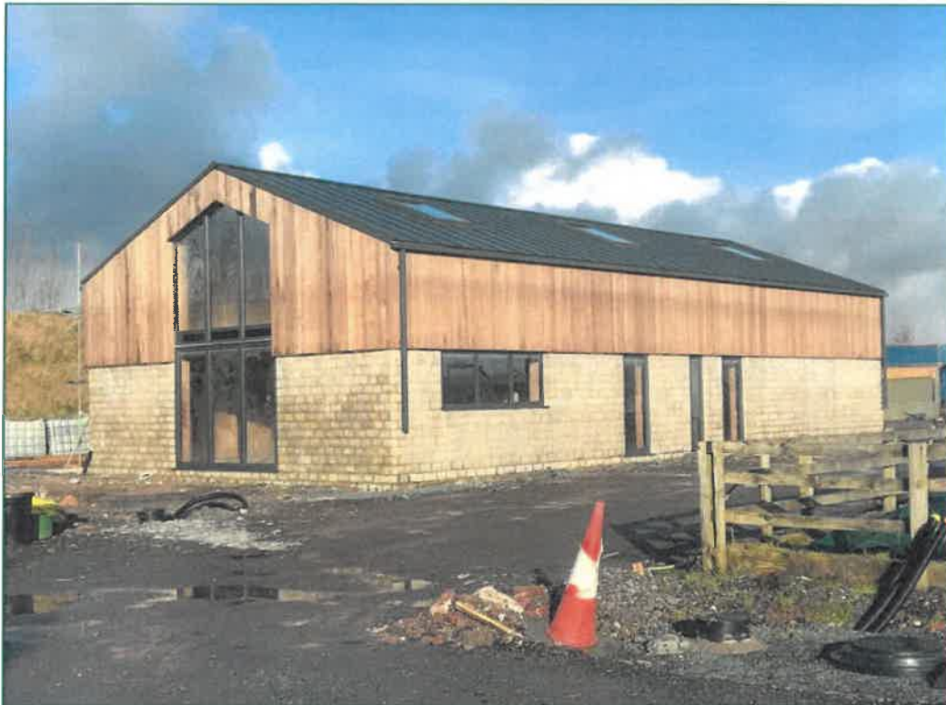
Photo of Completed Class Q conversion
