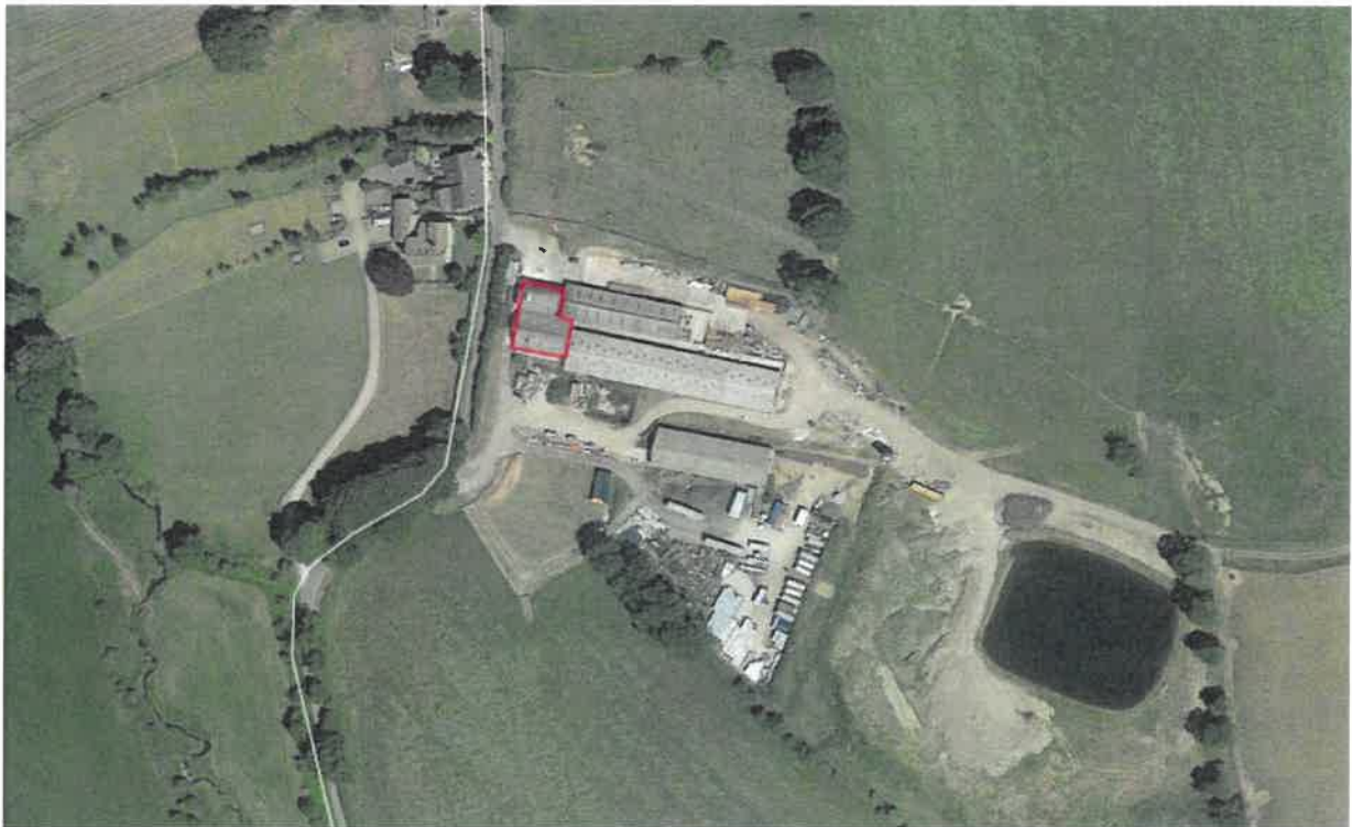
Figure 4: Location of buildings on western edge of Horton Grange Farm farmyard.
