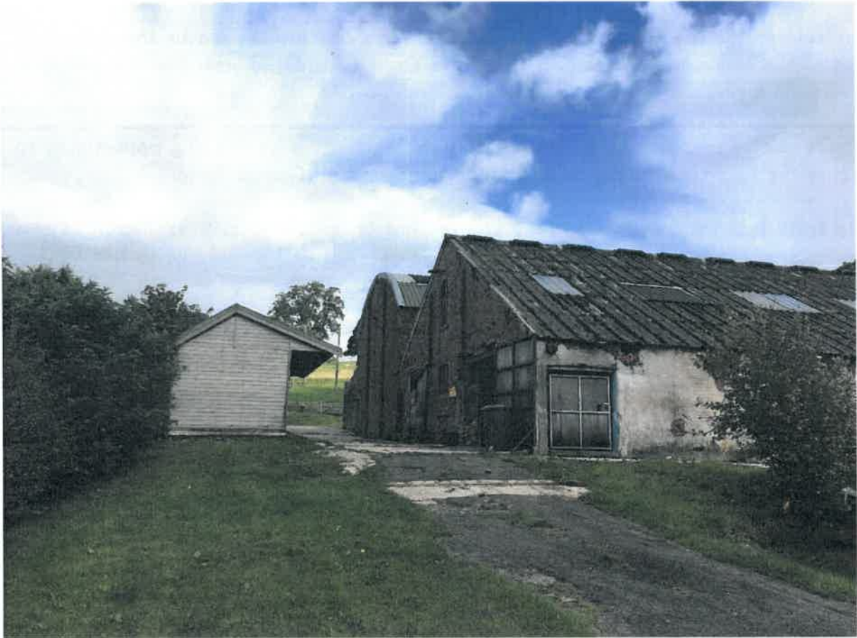
Photograph 1: Proposed buildings viewed from the south
