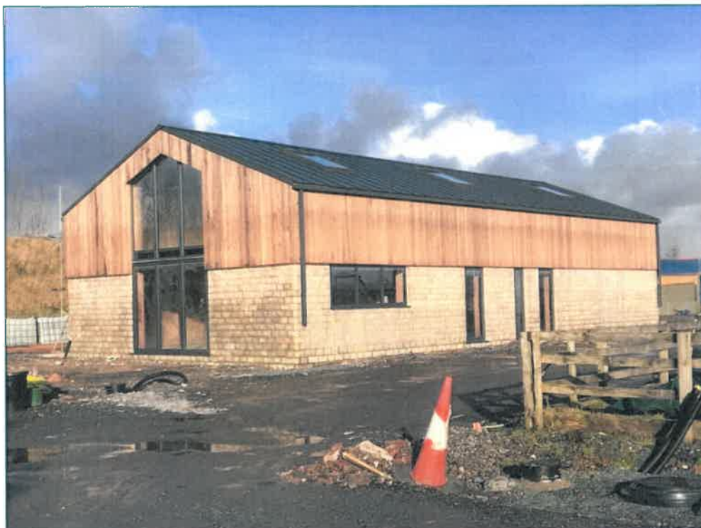
Photo of Completed Class Q conversion
