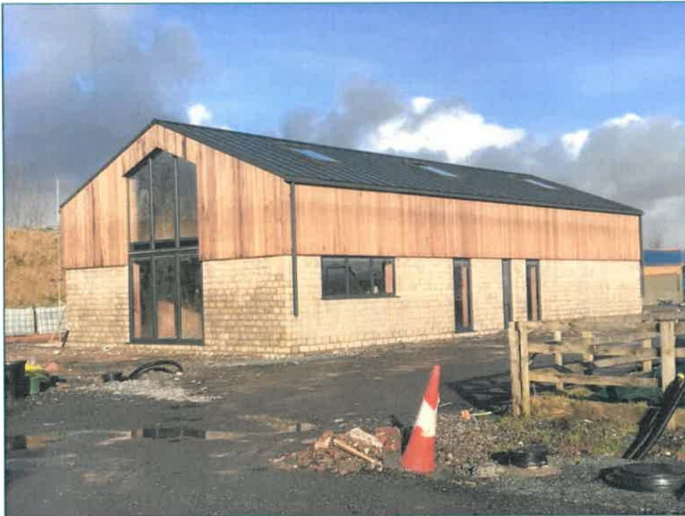
Photo of Completed Class Q conversion
