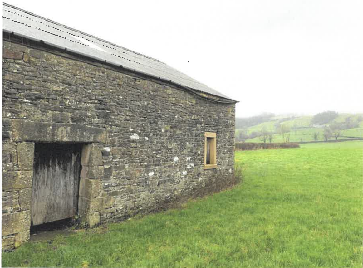
Photo 15 - South Elevation – mid section
