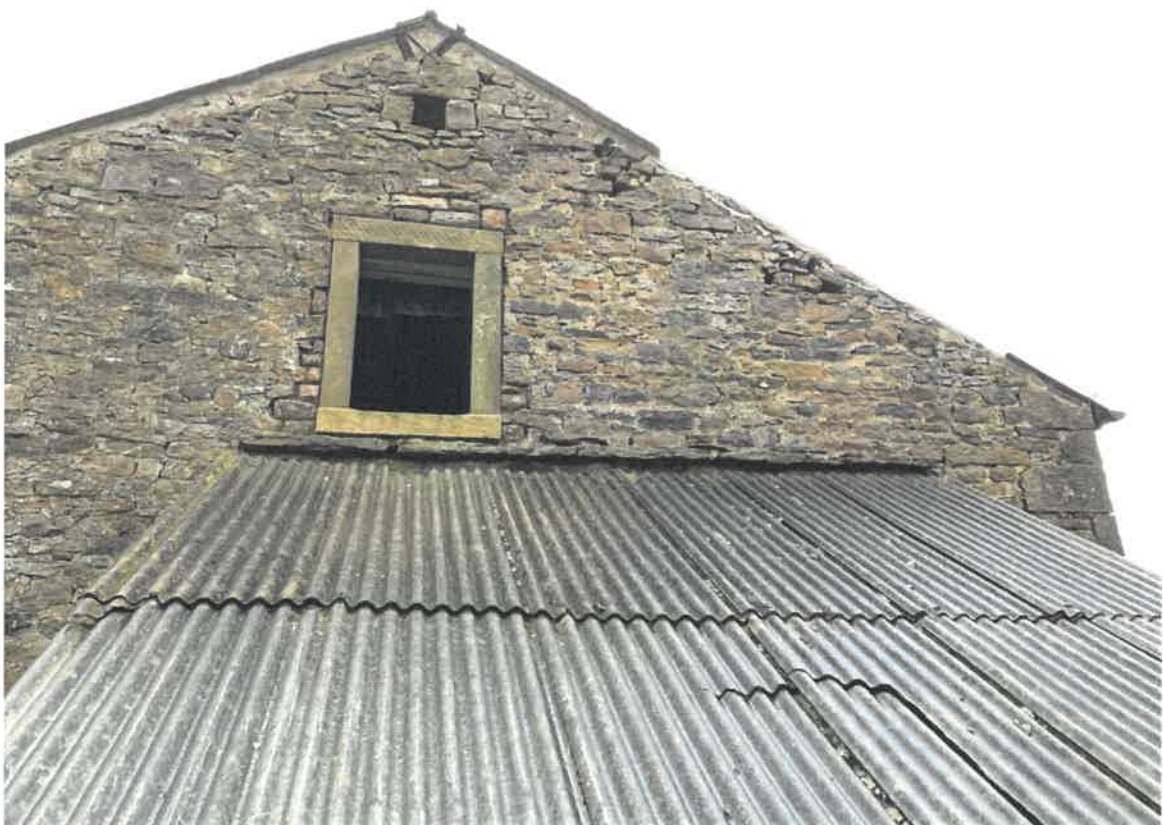
Photo 22 – East gable Upper and roof to lean to
