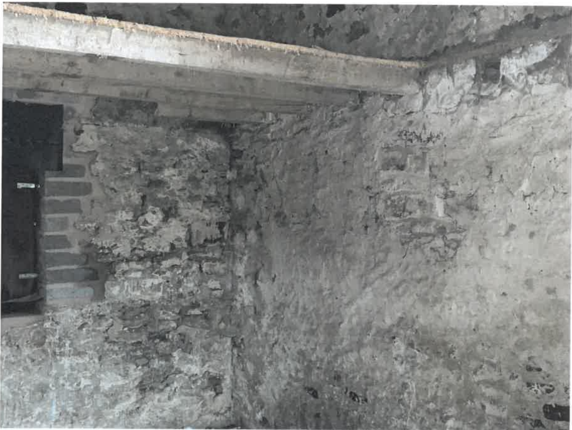
Photo 28 – Timbers to loft
