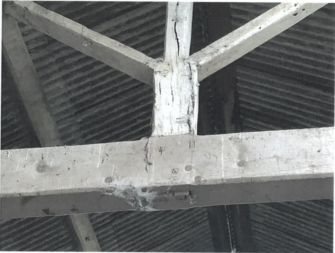
Photo 27 – Roof Truss detail
