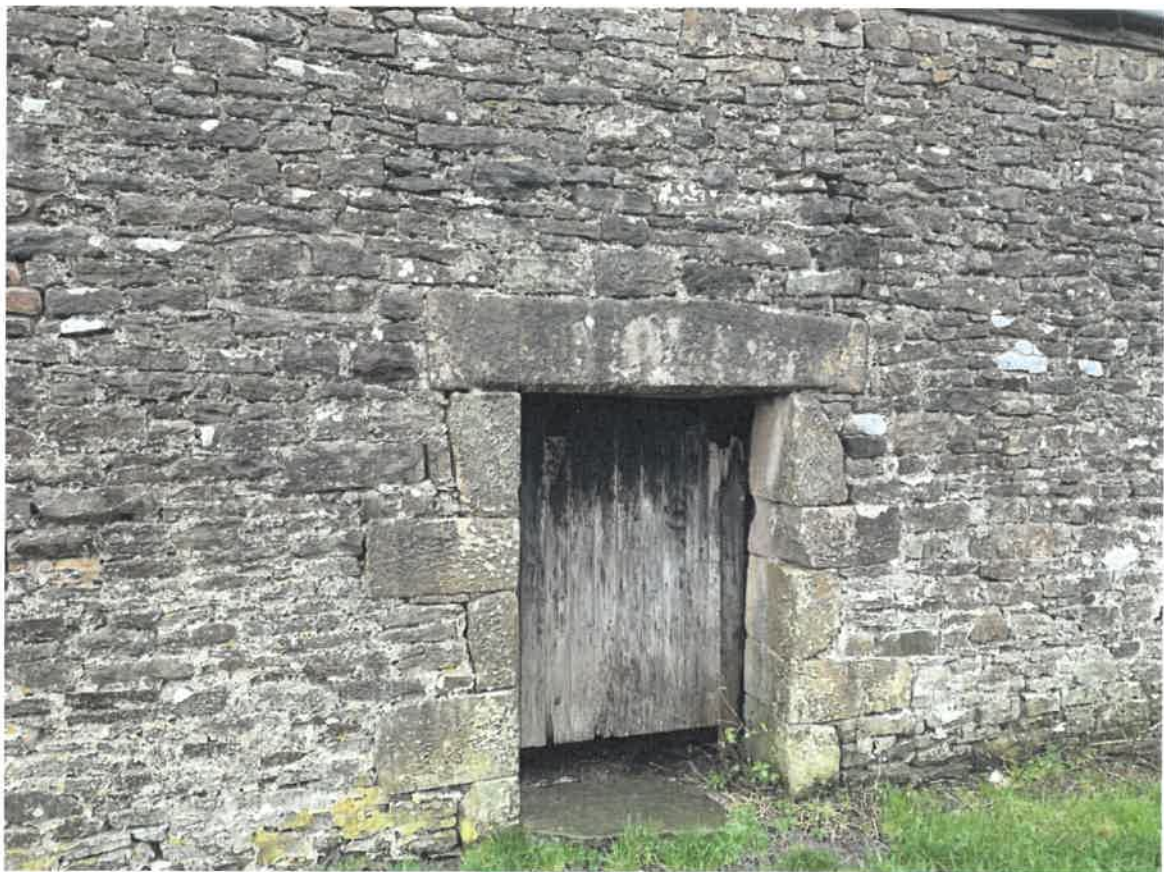
Photo 16 - South Elevation – Door
