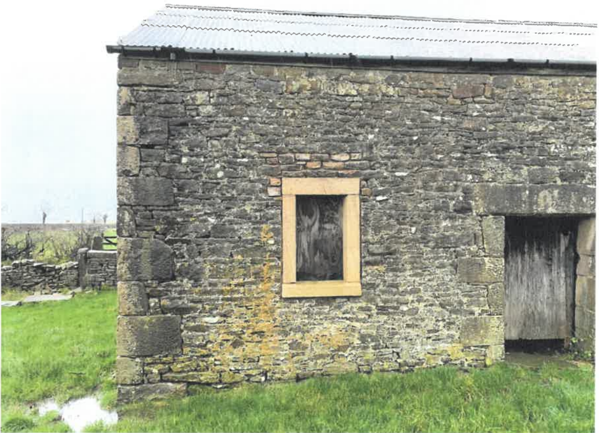
Photo 14 - South Elevation – West End
