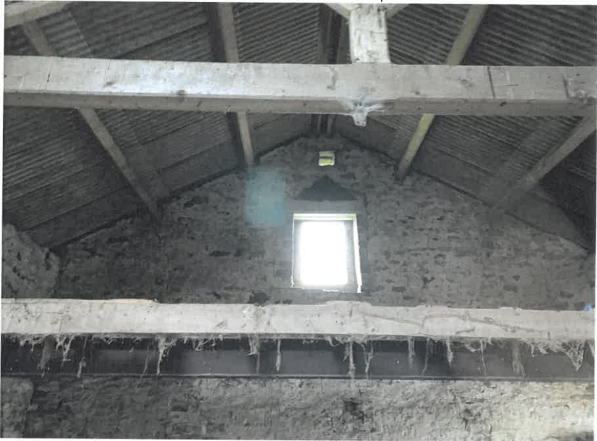
Photo 29 – Truss and loft timber
