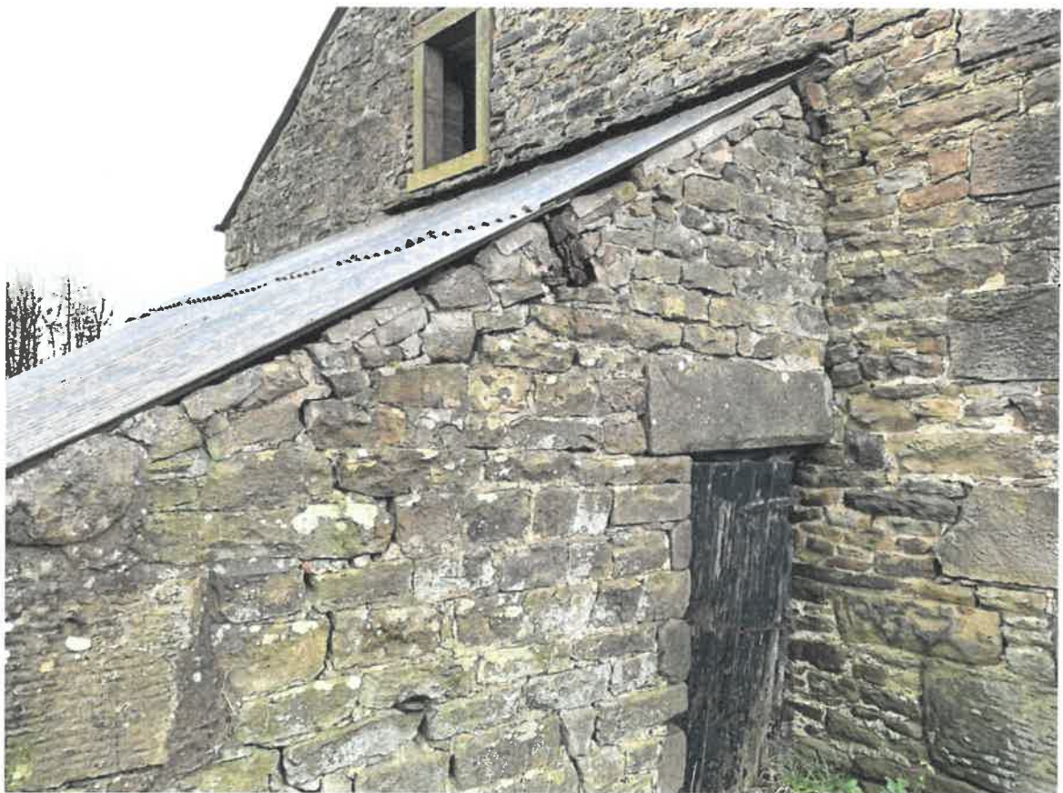
Photo 2 – North Elevation – Lean to
