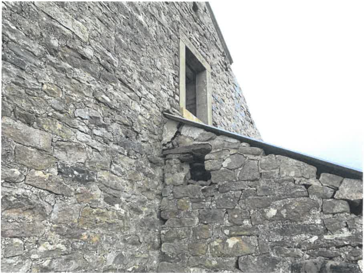
Photo 21 – East gable and lean to
