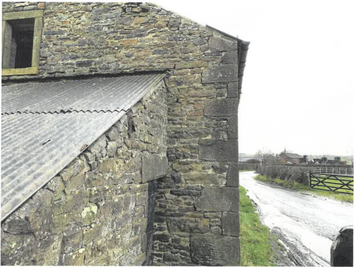
Photo 3- North Elevation – Lean to and North East Corner
