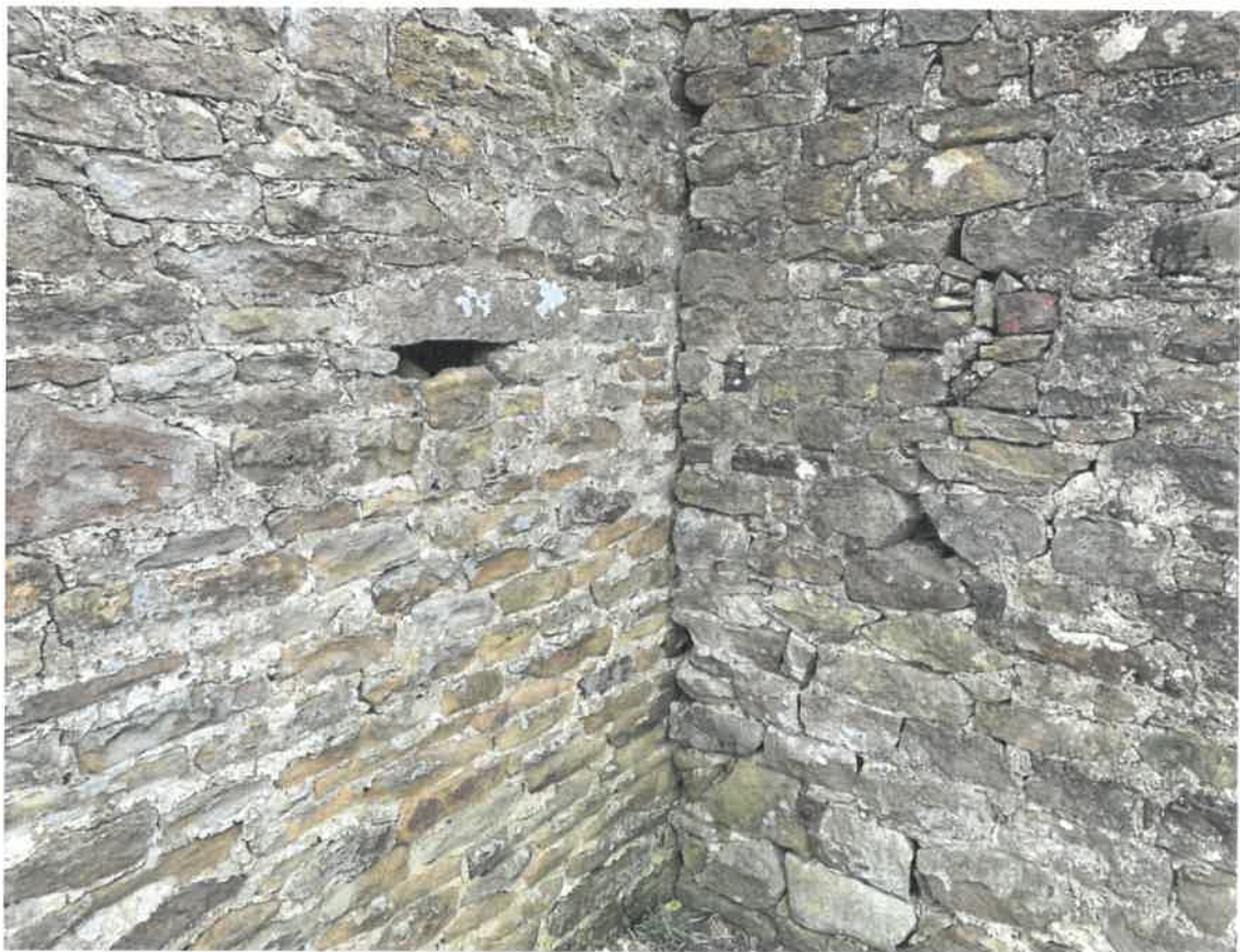
Photo 20 – East gable – joint with Lean to
