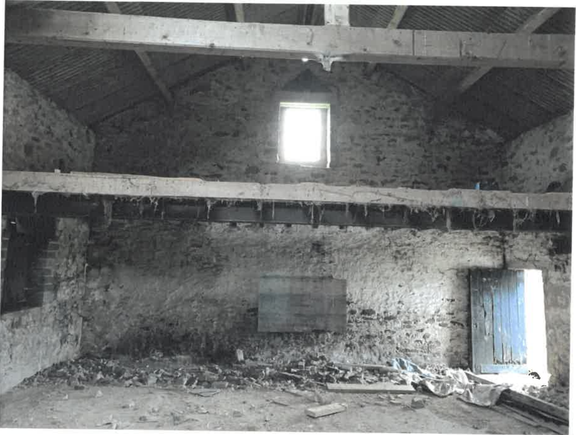
Photo 23 – Internal looking west
