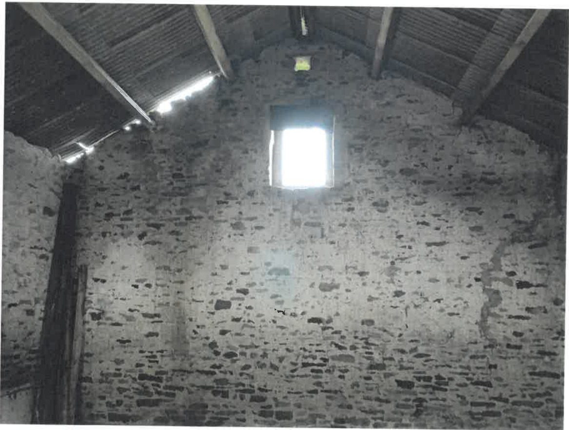
Photo 24 – Internal looking east
