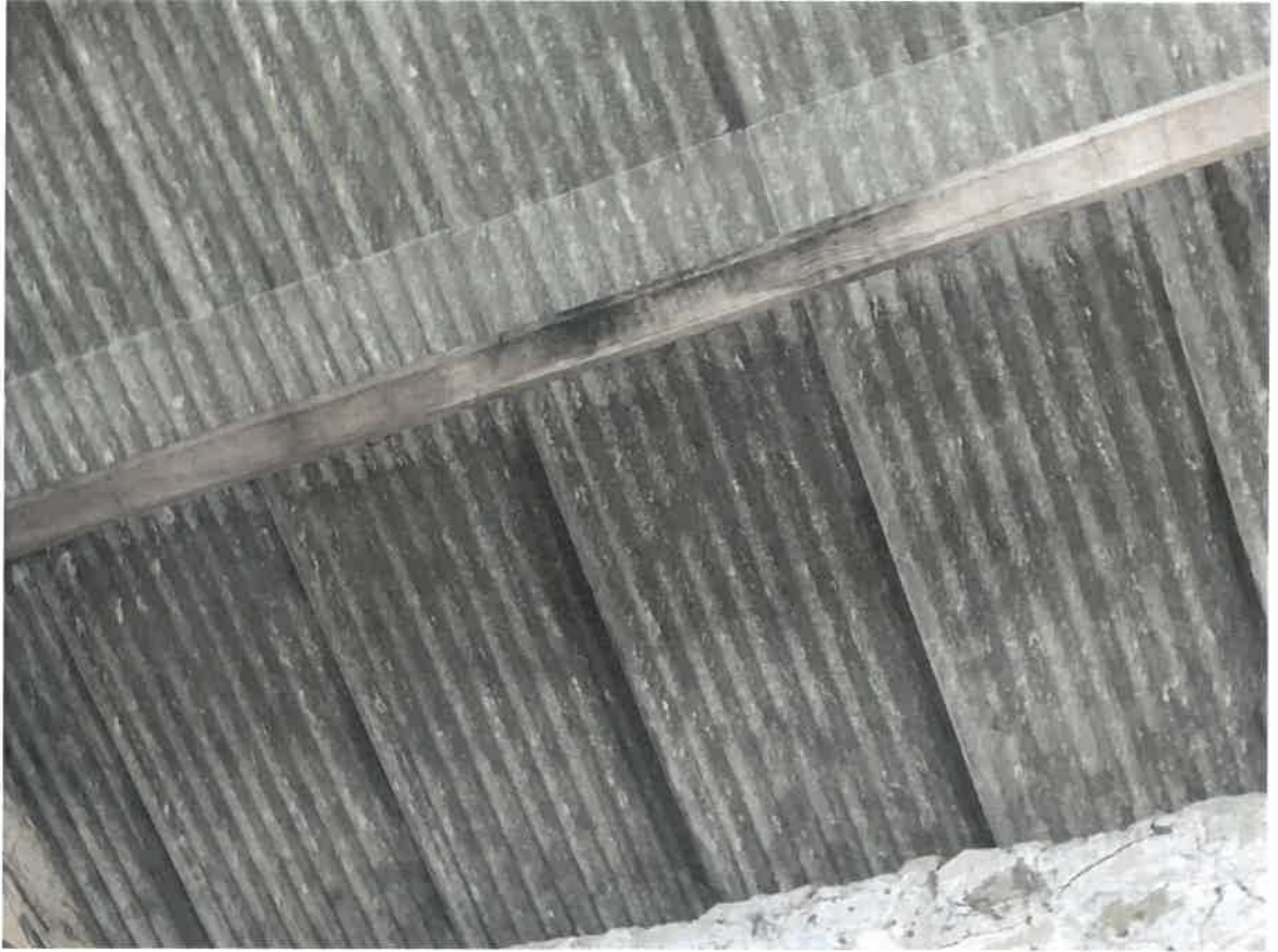
Photo 37 – Roof Purlin and sheeting
