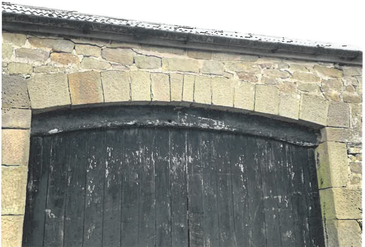
Photo 4 – North Elevation - Door
