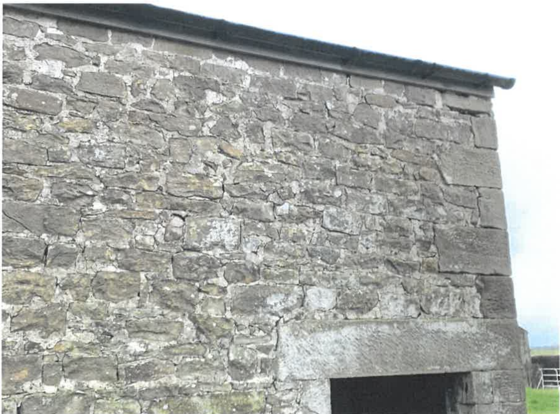
Photo 6 – North Elevation West Corner
