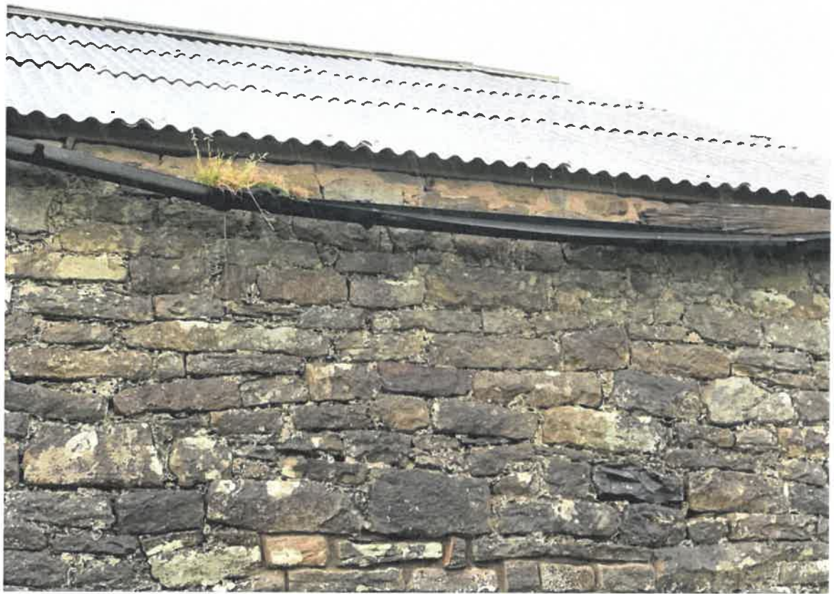
Photo 17 - South Elevation – upper section with gutter
