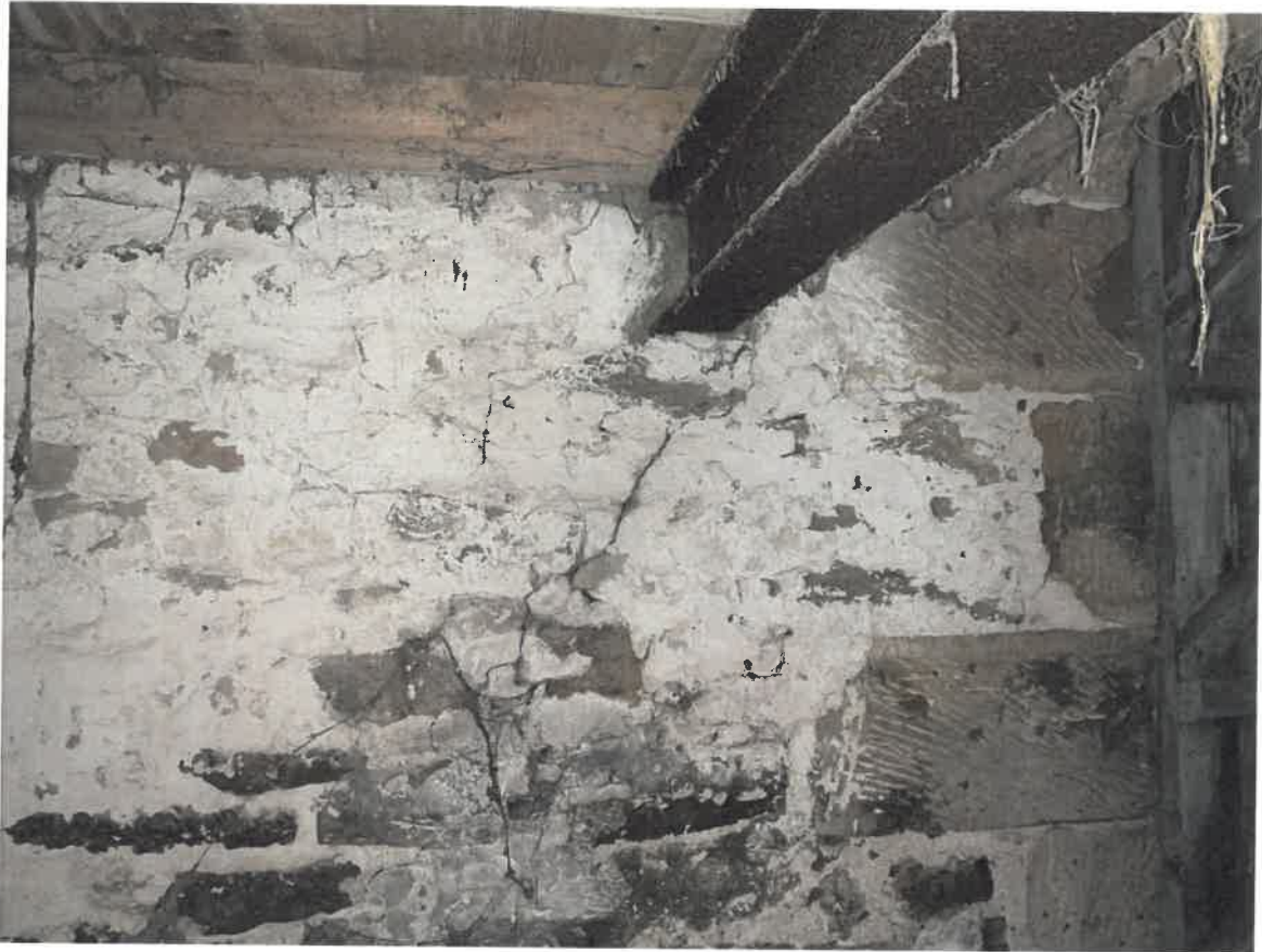
Photo 25 – Steel beam to loft
