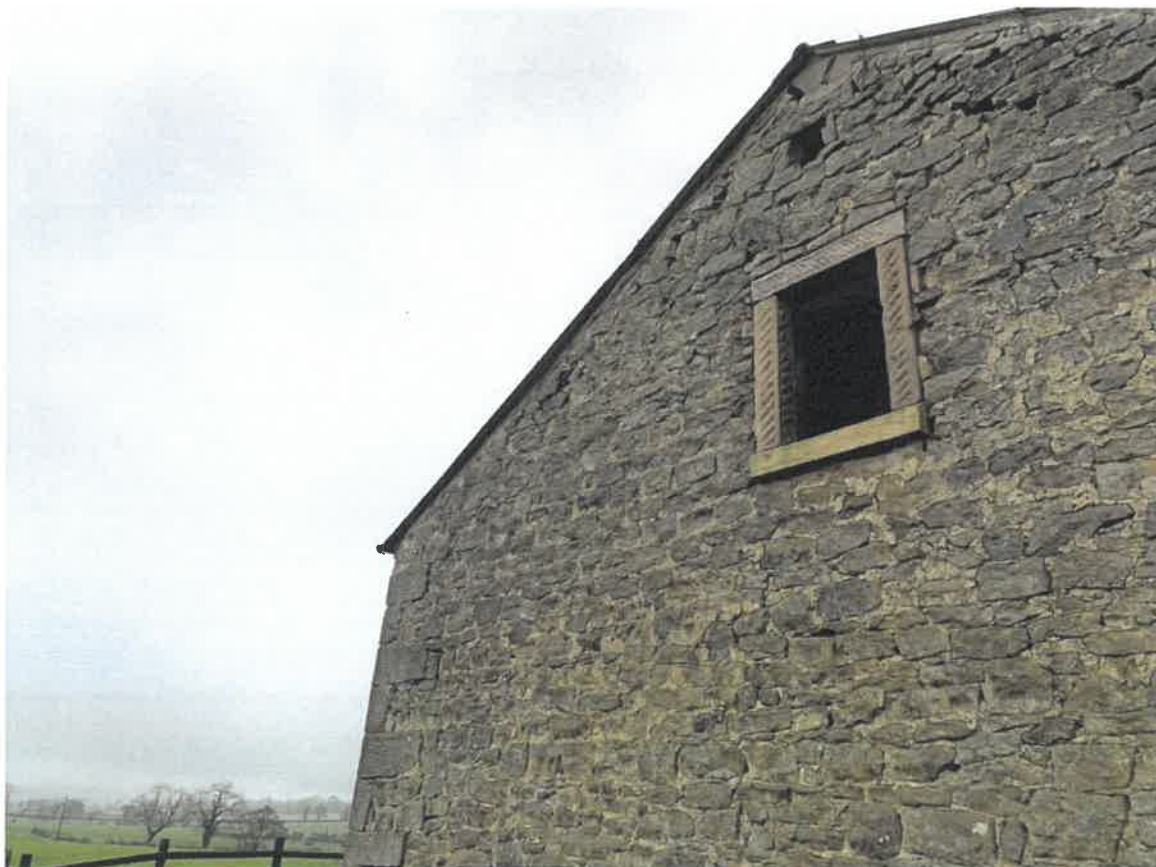
Photo 12 – West Gable – Higher Window and Owl Box
