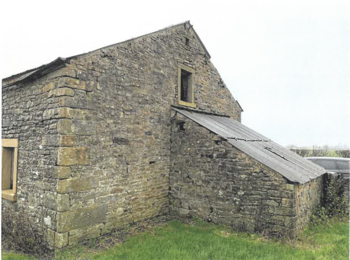
Photo 18 - East gable and Lean to
