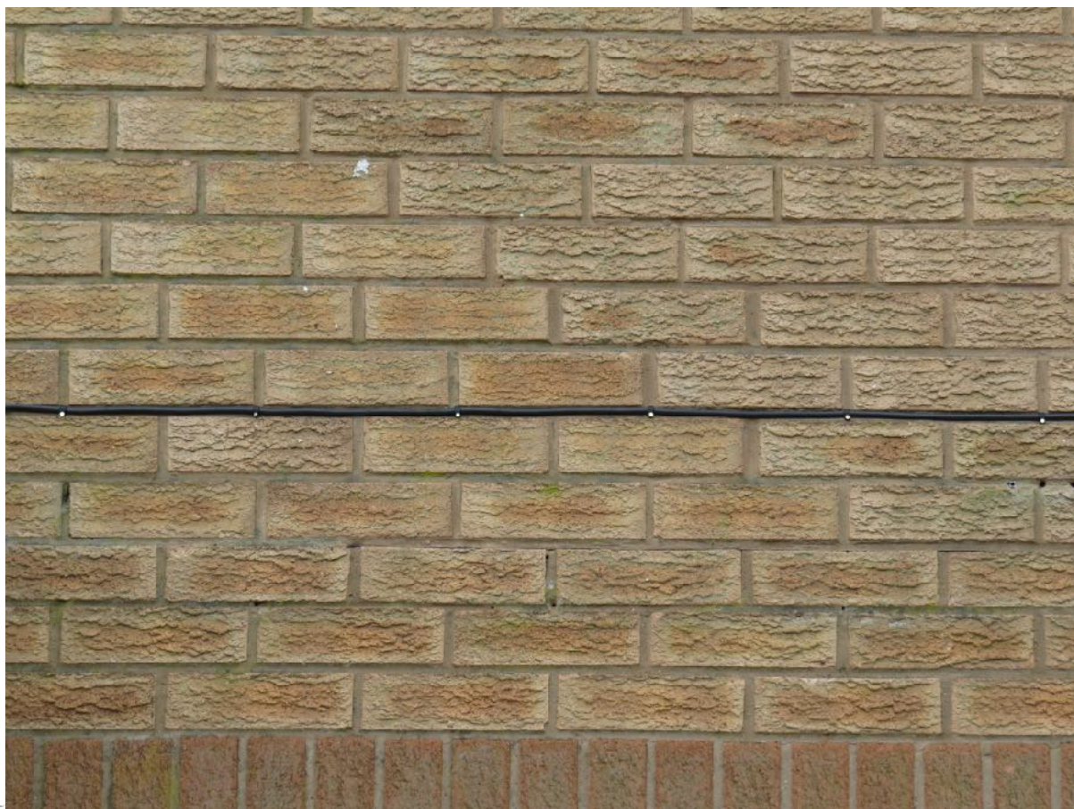
6 – Brickwork is in good condition with no gaps in mortar.
