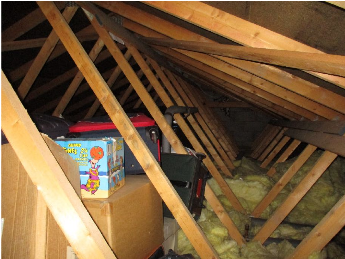
3.2a – The main roof void.
