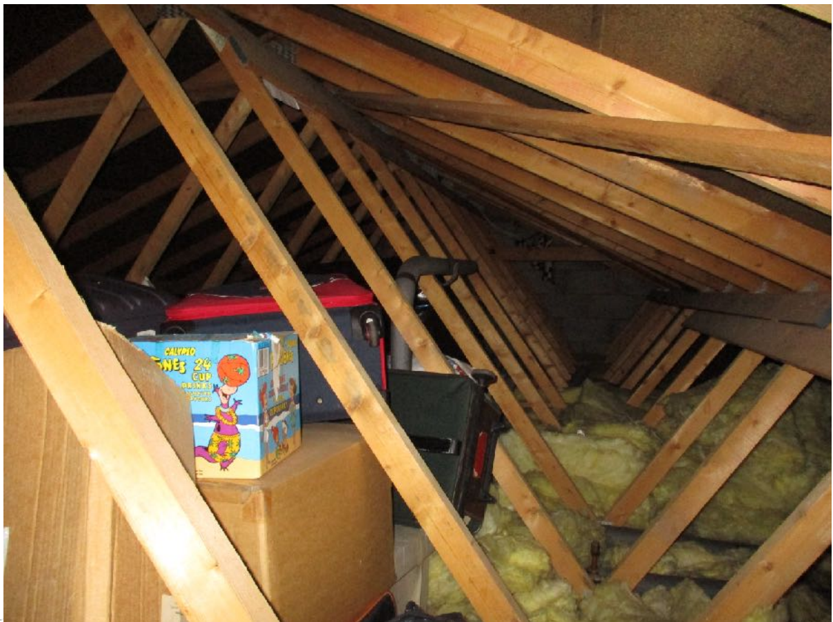
10 – The house has a single roof void lined with bitumen felt.
