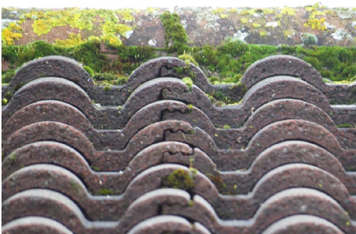
3 – Ridge tiles are sealed with cement, roof tiles are tightly fitted.
