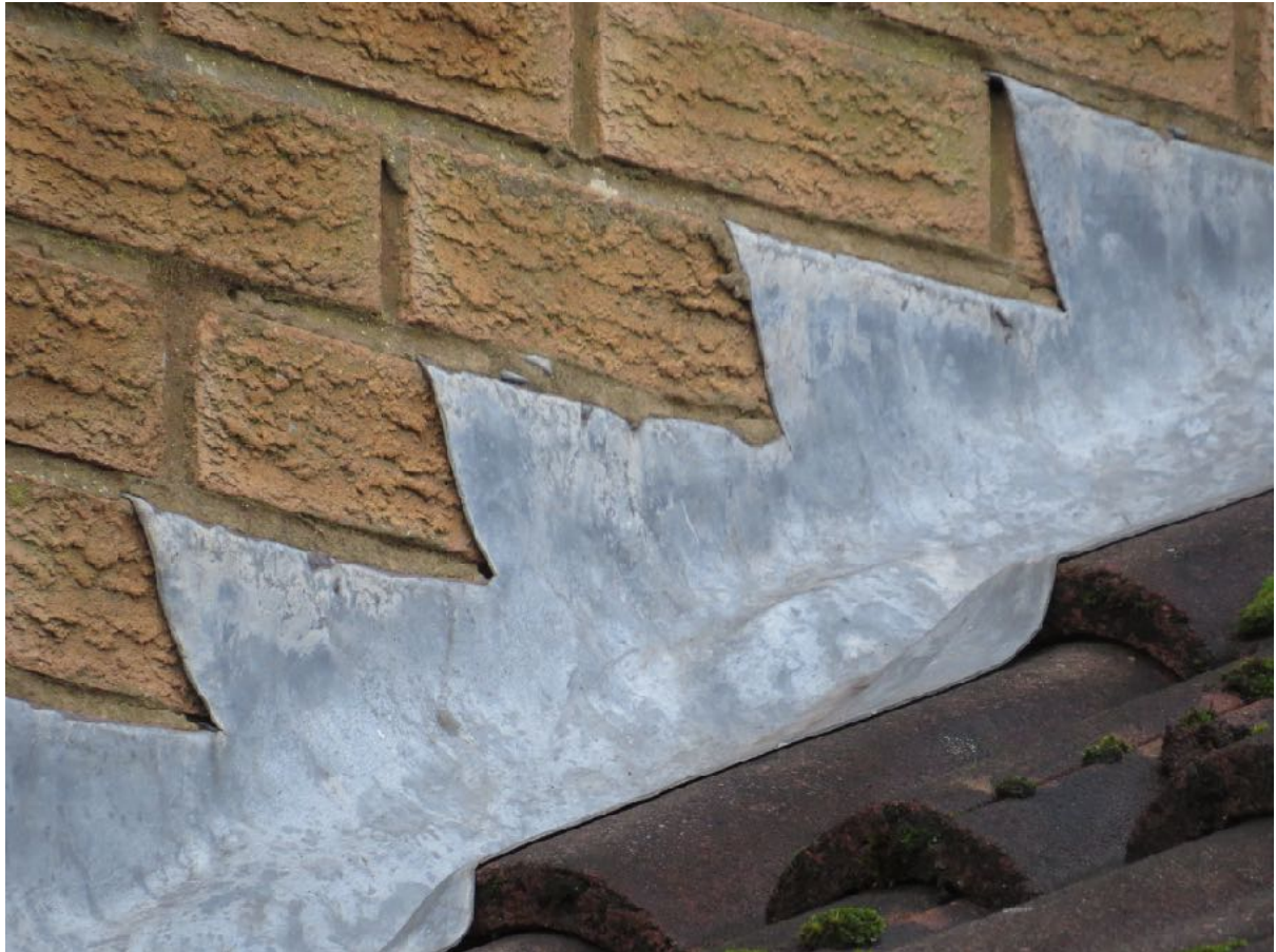
9 – Lead flashing is tightly fitted with no suitable gaps.
