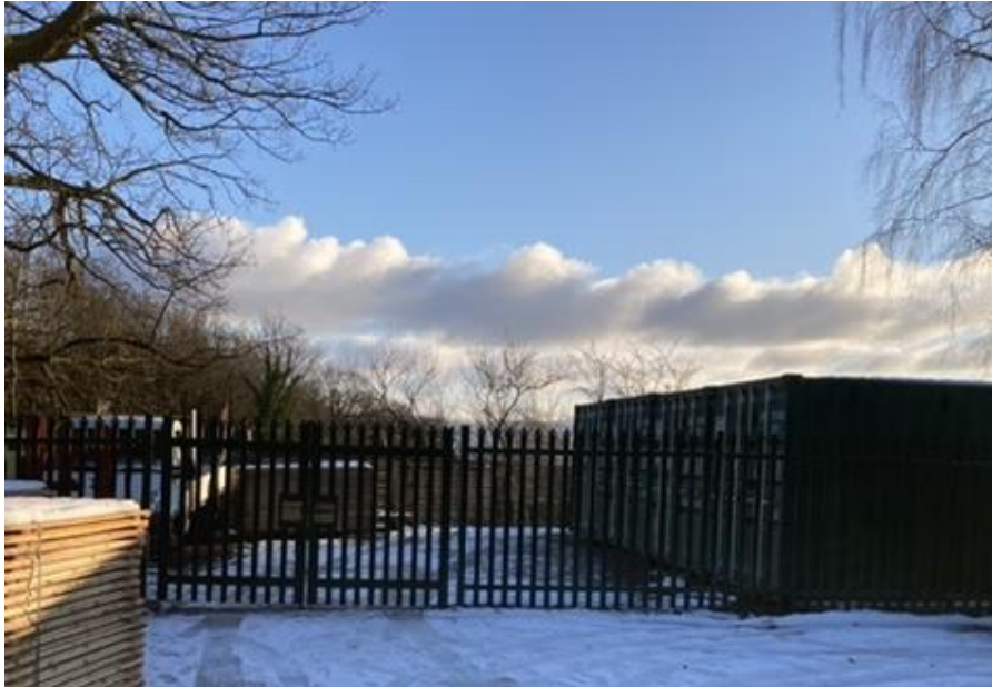
Existing secure perimeter fencing and containers
