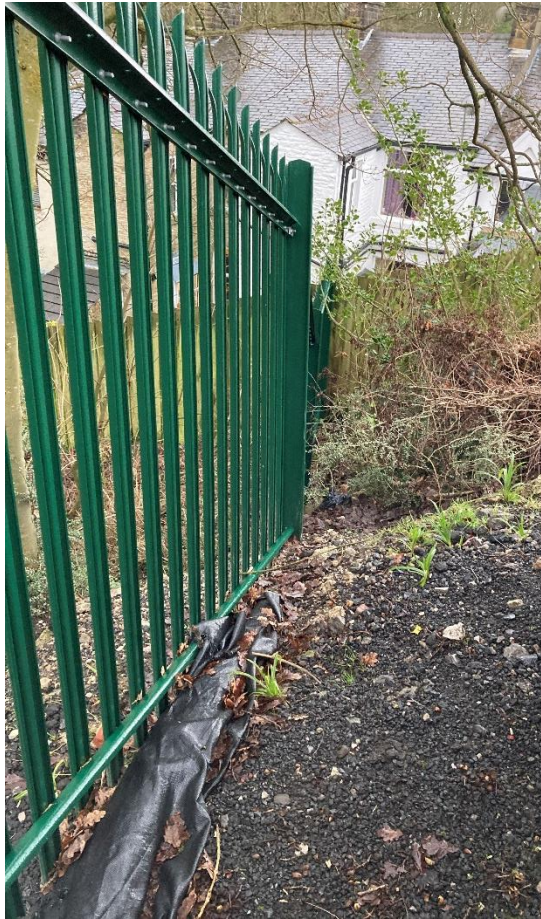
Existing secure perimeter fencing
