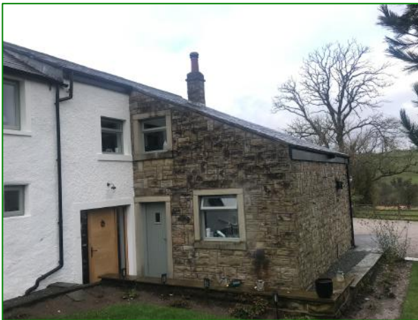
The southeast elevation of the garage extension
