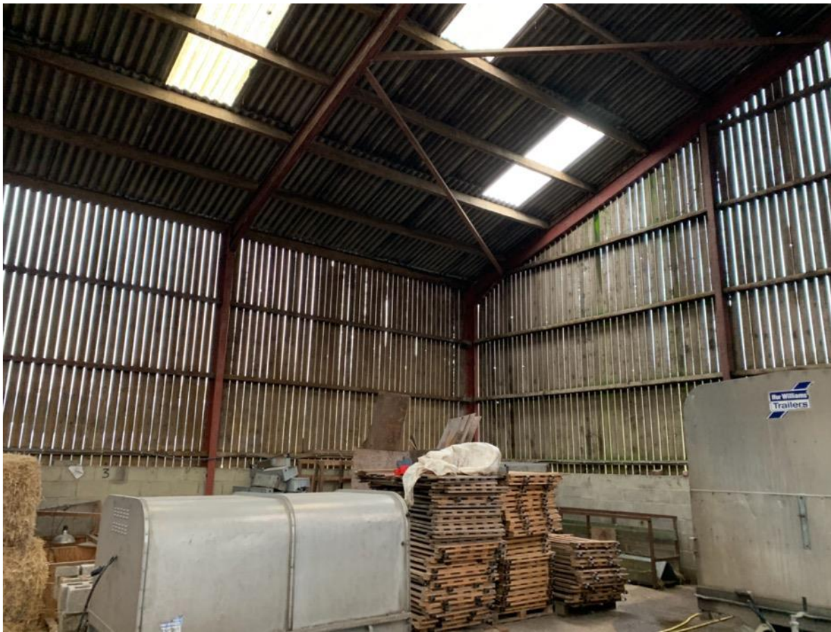
Photo 21 – Internal – North East Corner
