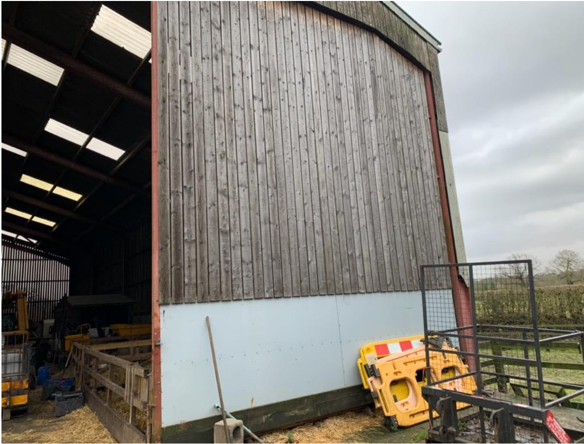
Photo 2 – West Elevation (South Corner)
