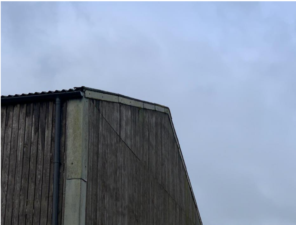
Photo 13 – South East Corner
