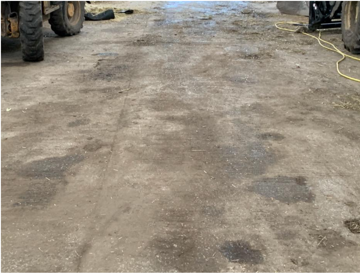
Photo 24 – Internal – Floor Slab
