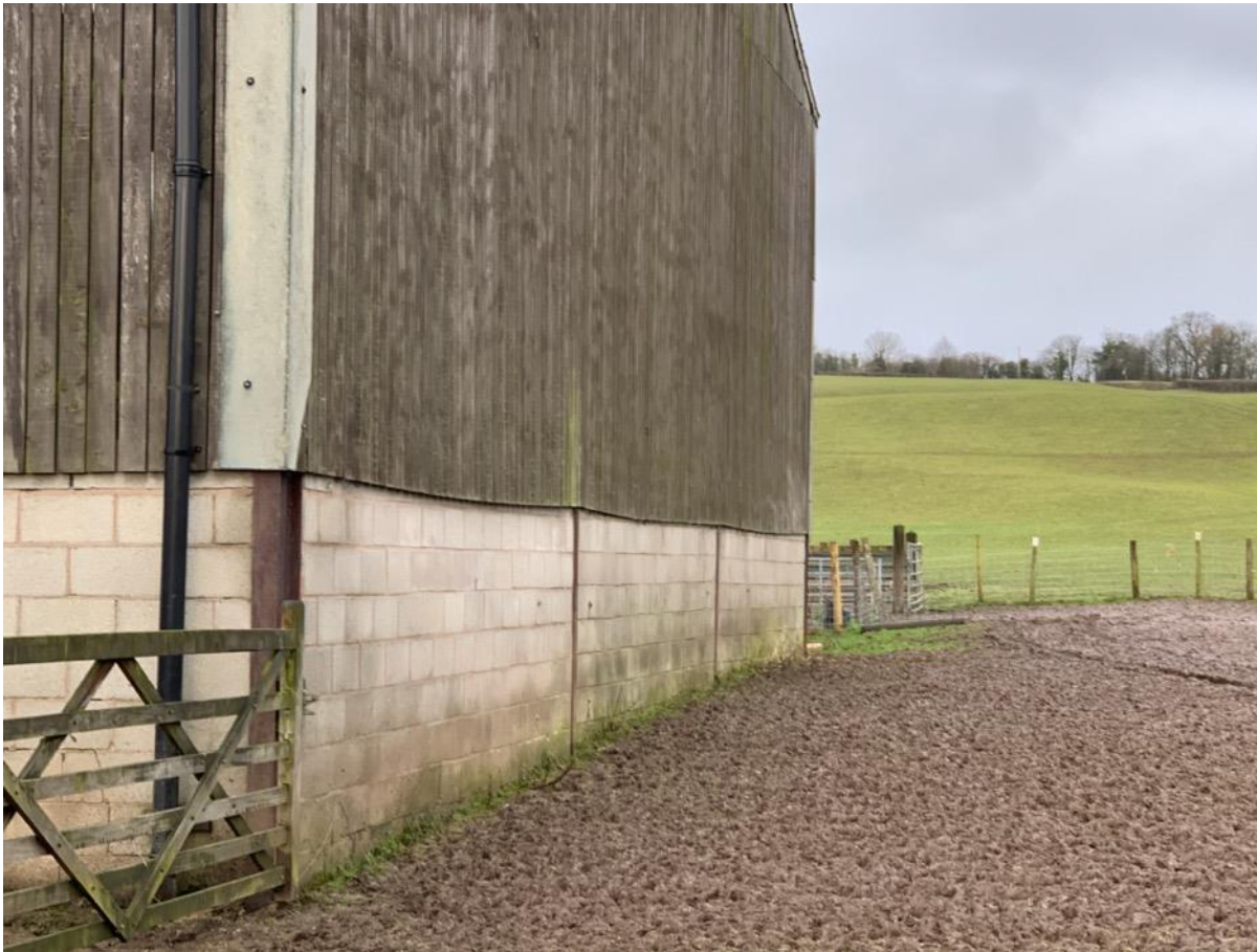
Photo 14 - East Elevation looking North
