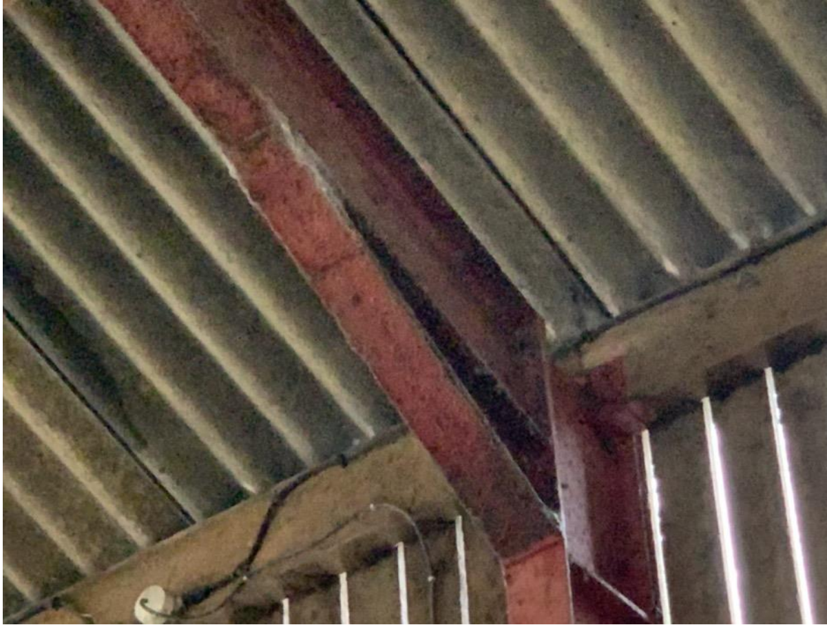
Photo 26 – Internal – Frame Haunch Detail
