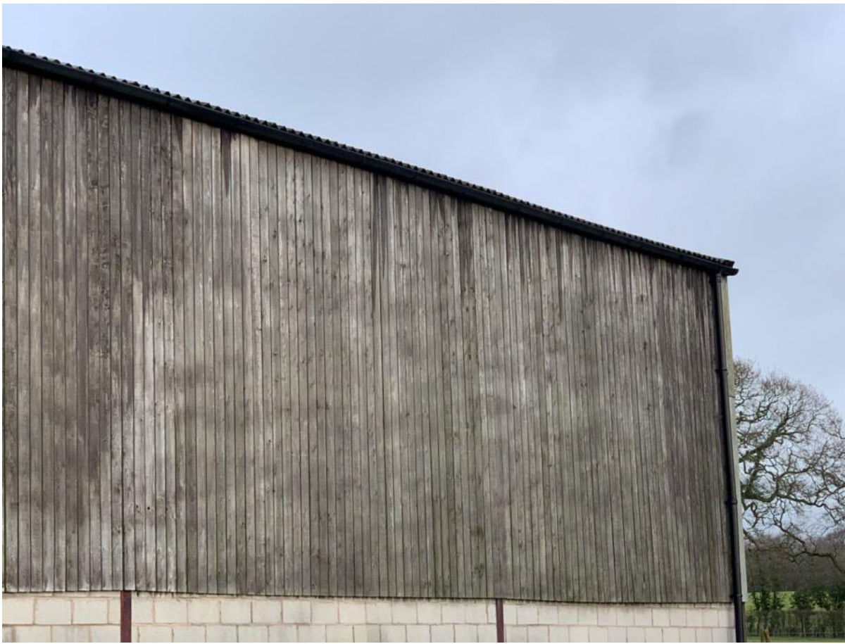
Photo 11 – South Elevation looking east
