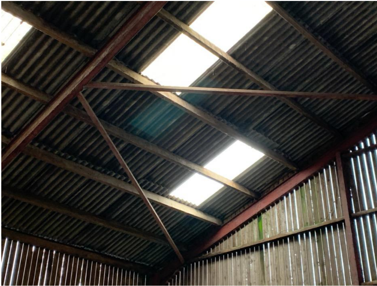
Photo 22 – Internal at North East Corner showing roof bracing
