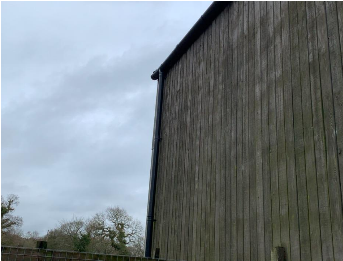
Photo 8 – Cladding and downspout to North Elevation at East end
