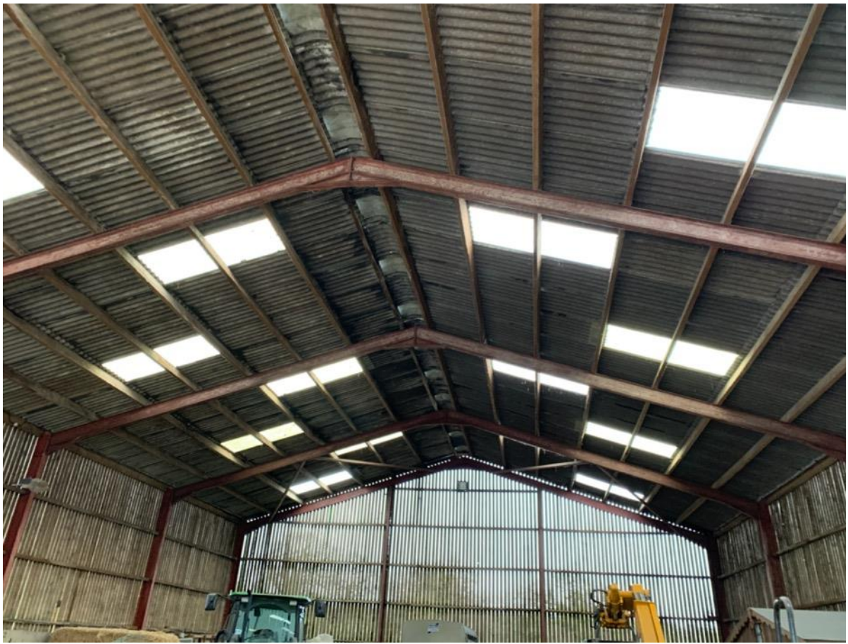
Photo 17 – Internal looking East
