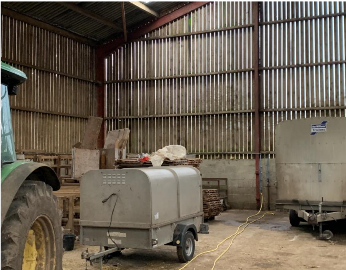
Photo 19 – Internal - North East corner
