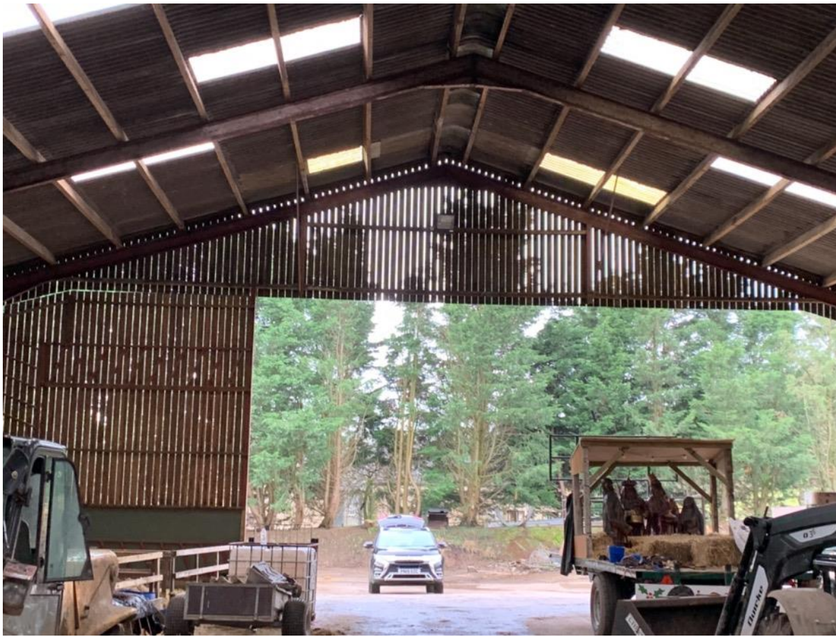
Photo 25 – Internal looking West
