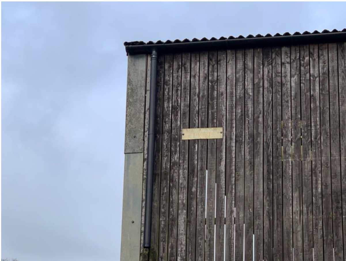
Photo 10 – West elevation at west end showing cladding, guttering and downspout
