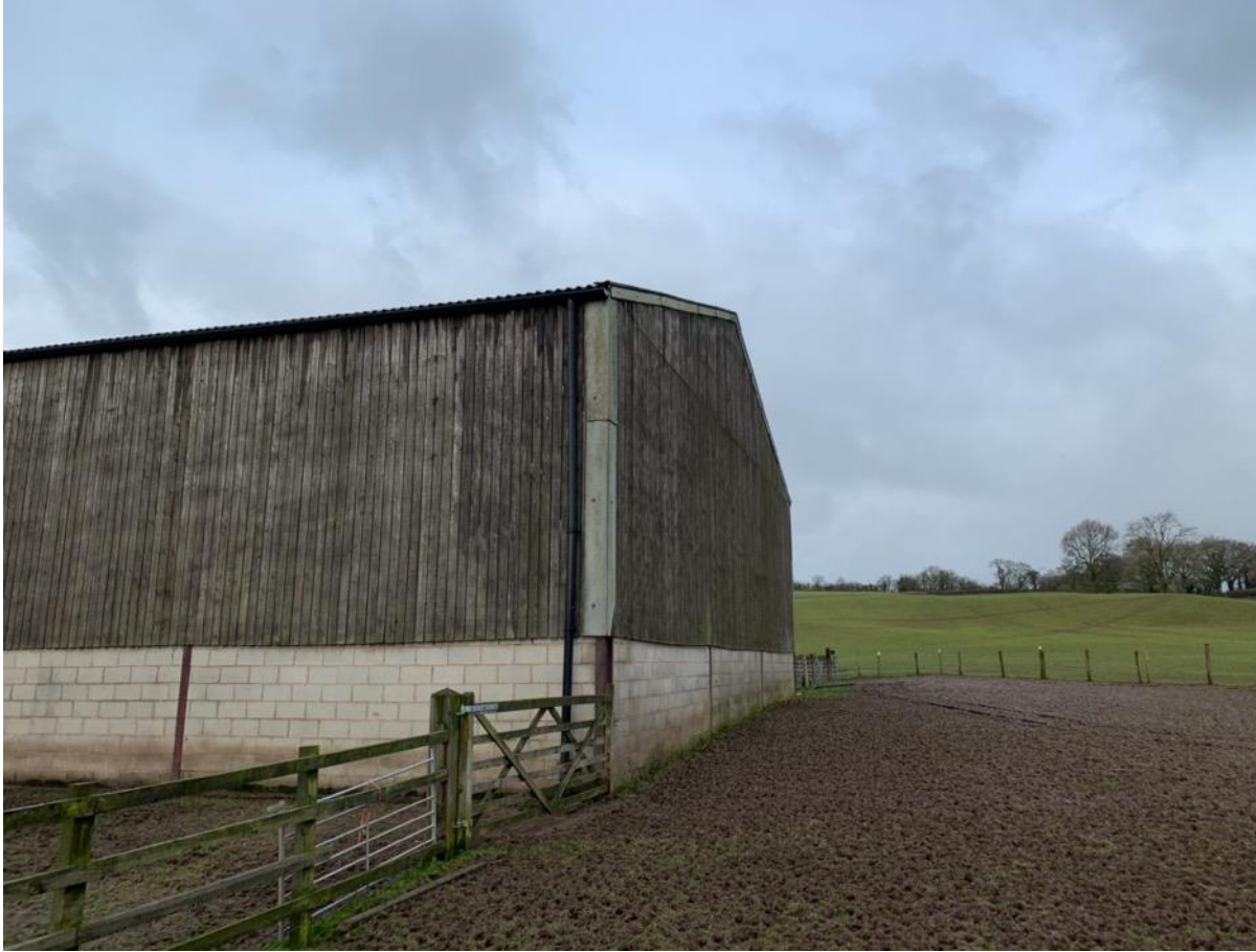
Photo 12 – South and East Elevations
