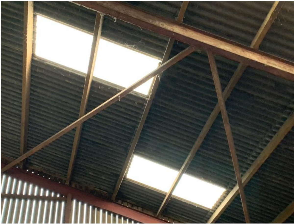
Photo 23 - Internal at North West Corner showing roof bracing
