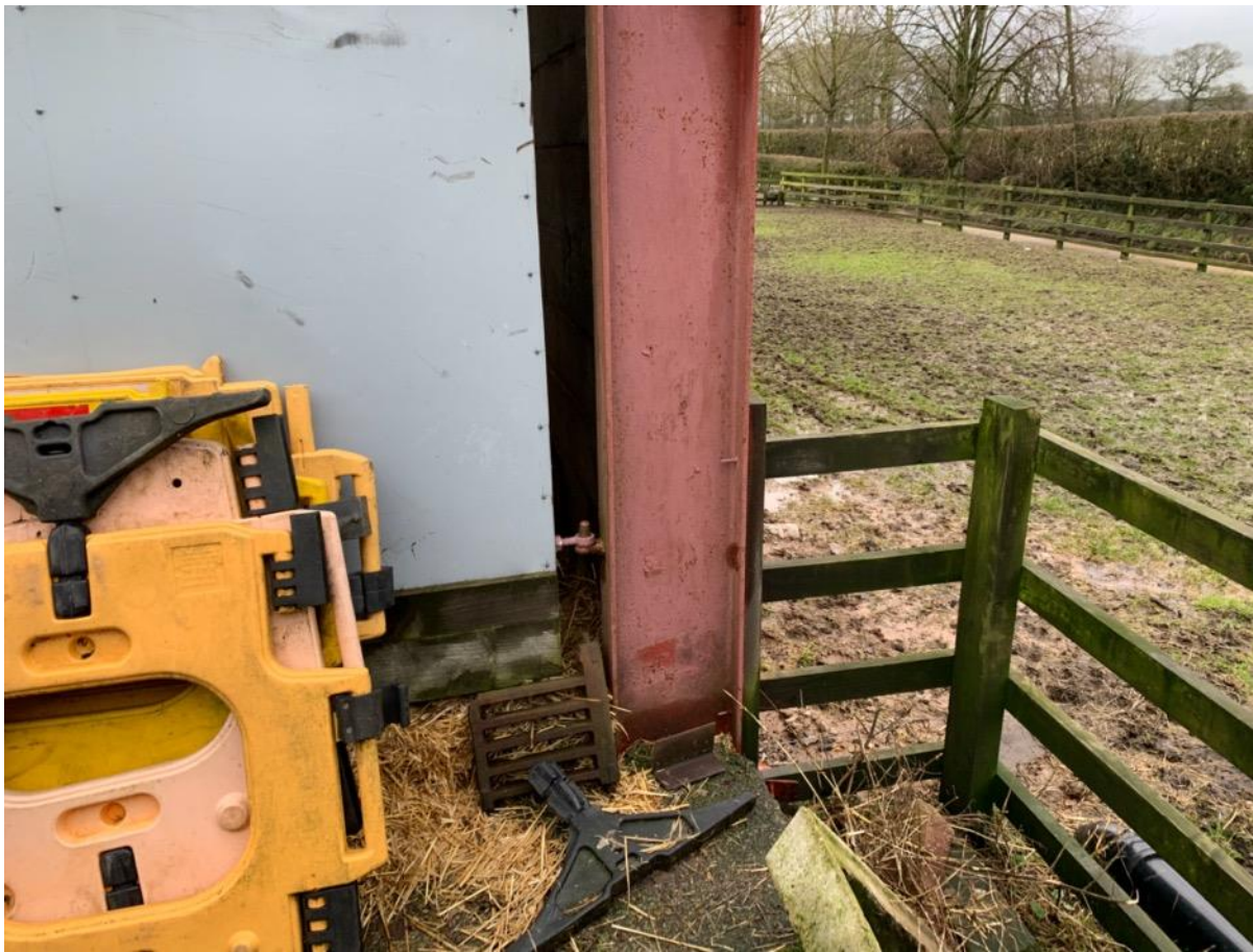
Photo 3 – Column at South West Corner
