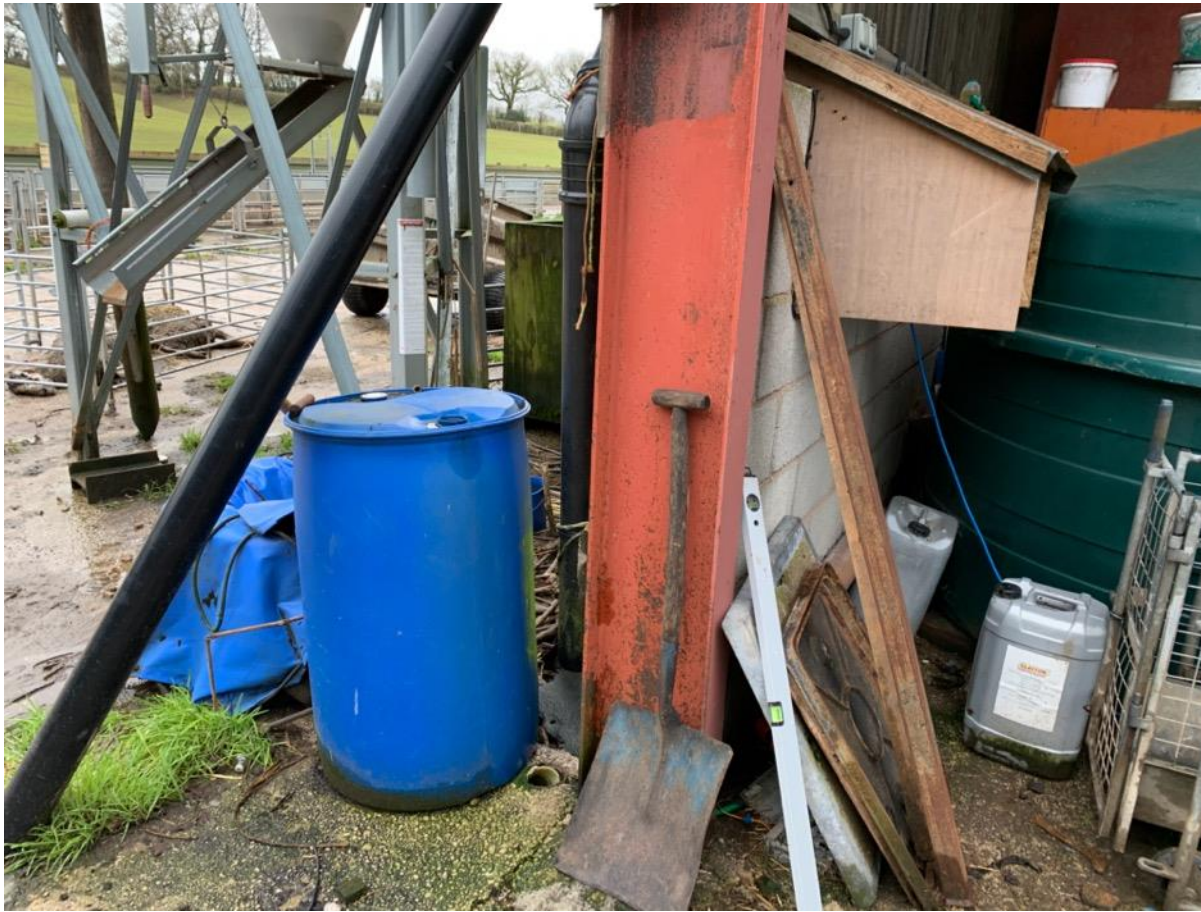
Photo 4 – Column at North West Corner
