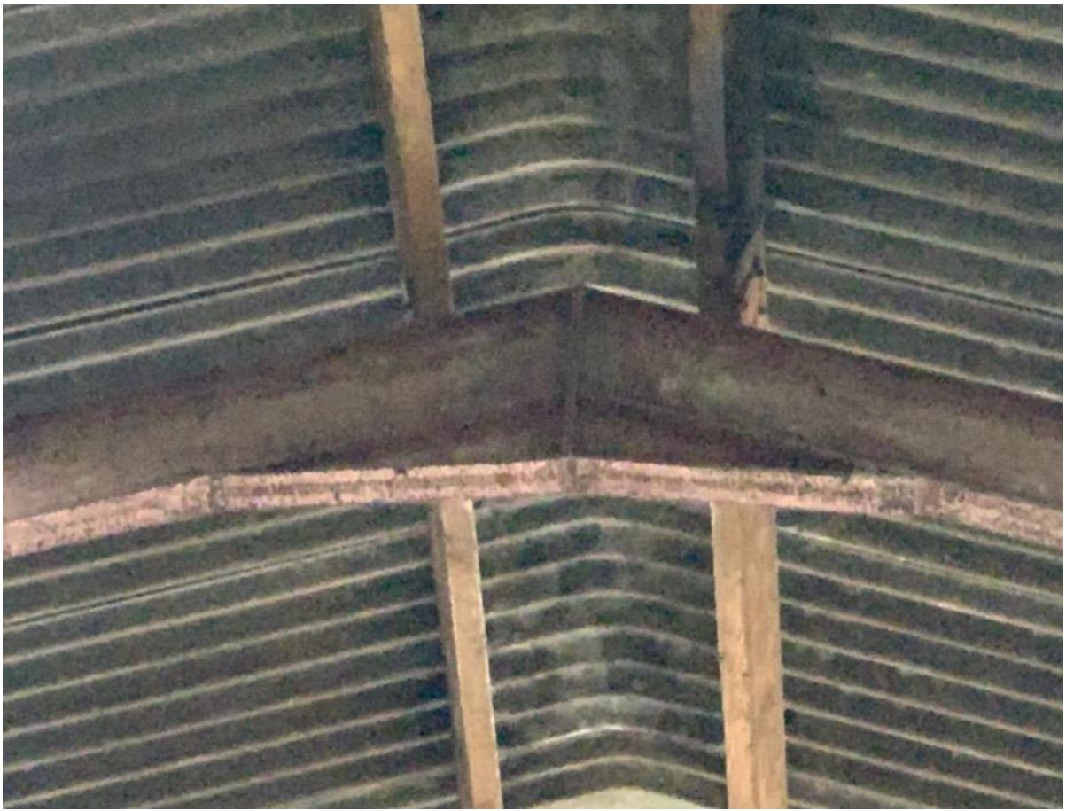
Photo 27 – Internal – Frame Apex
