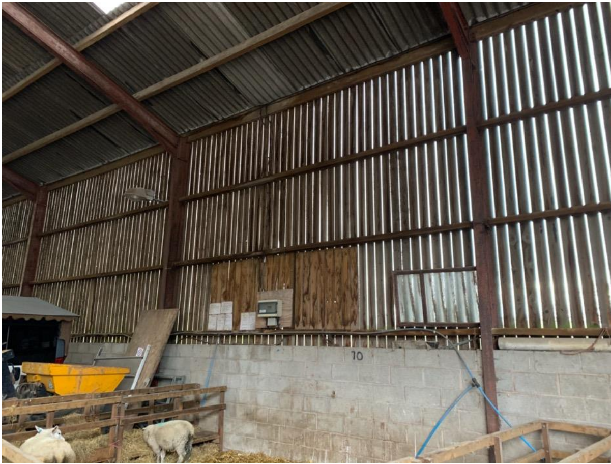
Photo 16 – Internal South Elevation
