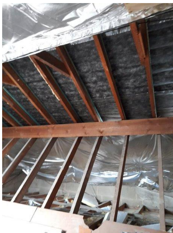
Plate 4: An image showing some of the under felt where the conversion done by the previous owner started.
