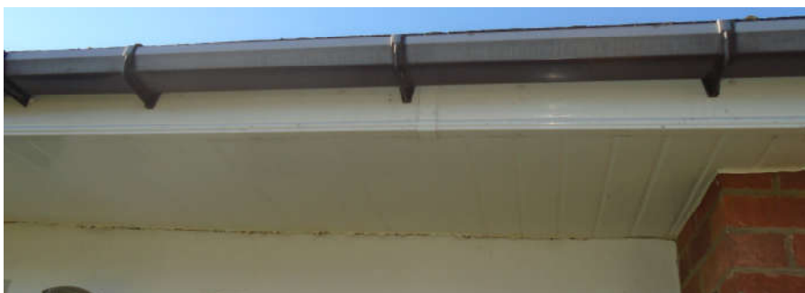
Section of roof adjacent to the proposed porch.
