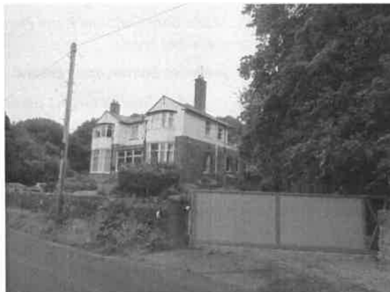
Photo 2: North-western and south-western elevations of the house at Whins Lodge and woodland surrounds
