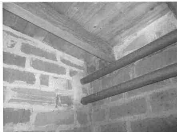
Photo 29: Interior of kennel building with sealed / pointed walls
