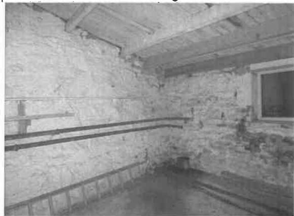
Photo 24: Interior of garage
