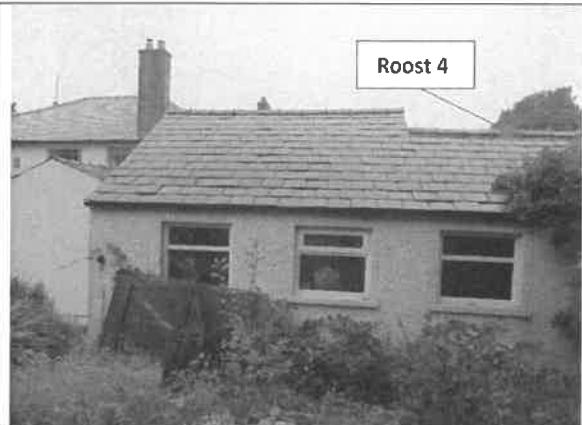
Photo 20: Roof and south-eastern elevation of outbuilding and location of Roost 4
