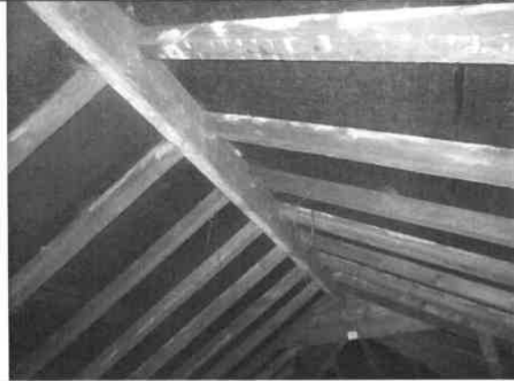
Photo 14: Traditional ridge board and bitumen undertile felt at the main house
