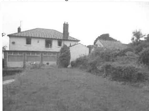
Photo 4: South-eastern (rear) elevation of Whins Lodge
