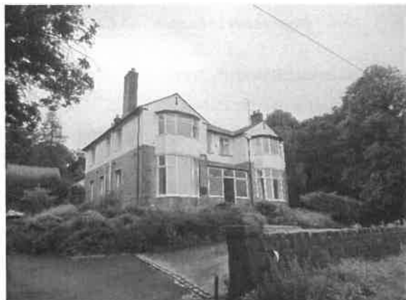
Photo 1: North-eastern and north-western elevations of the house at Whins Lodge and woodland surrounds
