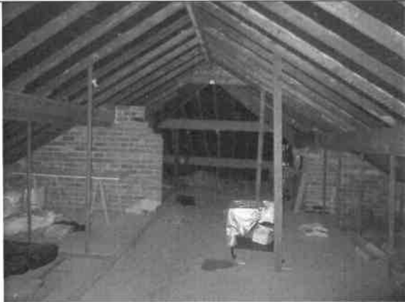
Photo 13: Roof void at the main house
