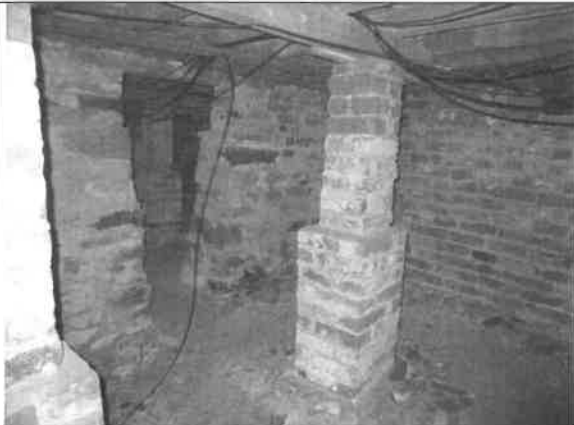
Photo 19: Cellar beneath the house
