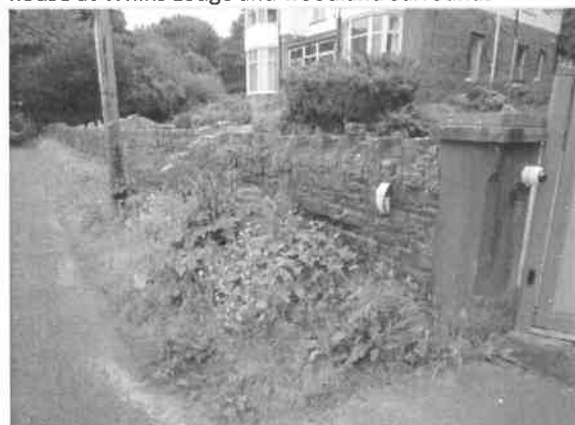
Photo 3: Wall along Whalley Old Road
