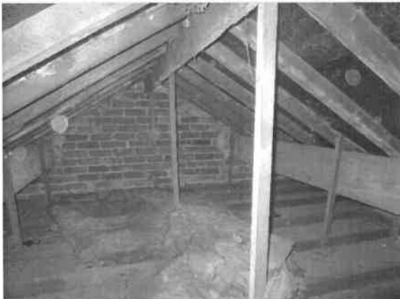
Photo 15: Roof void in the lower sections of roof at the house
