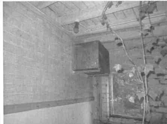
Photo 28: Interior of kennel building
