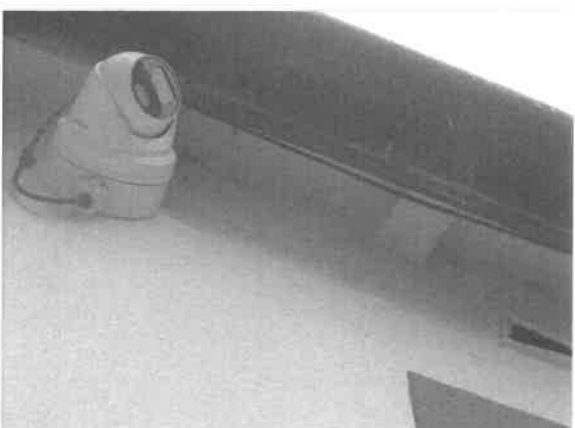
Photo 11: Sealed soffits at the house
