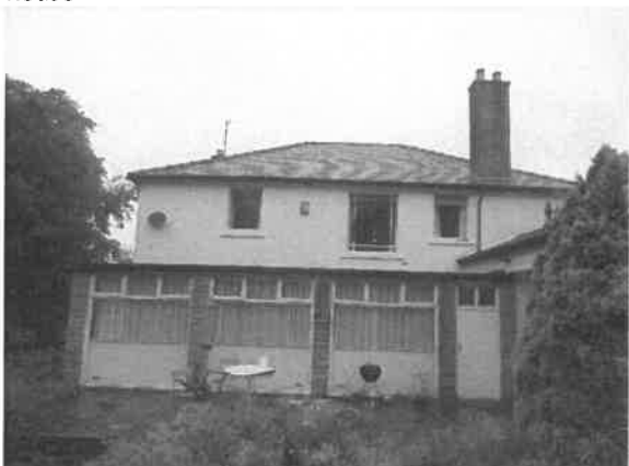
Photo 9: South-eastern elevation and roof of the house
