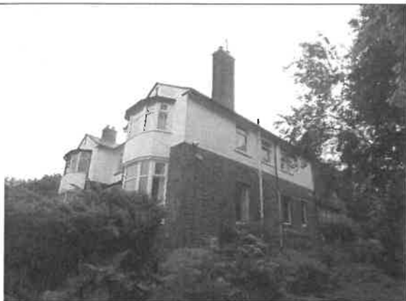
Photo 7: North-western and south-western elevations of the house
