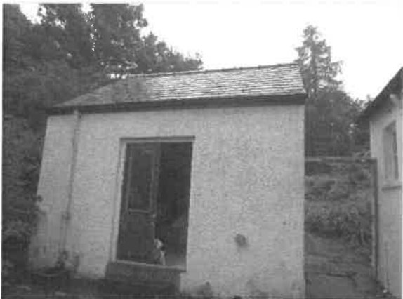
Photo 21: North-western elevation of the outbuilding
