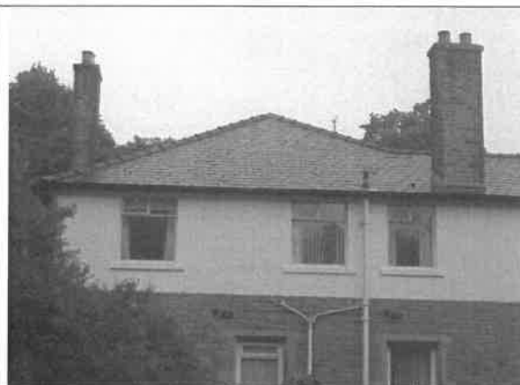
Photo 8: South-western elevation and roof of the house
