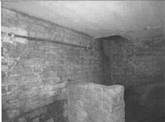
Photo 25: Annex to the north-west of the garage with sealed internal walls
