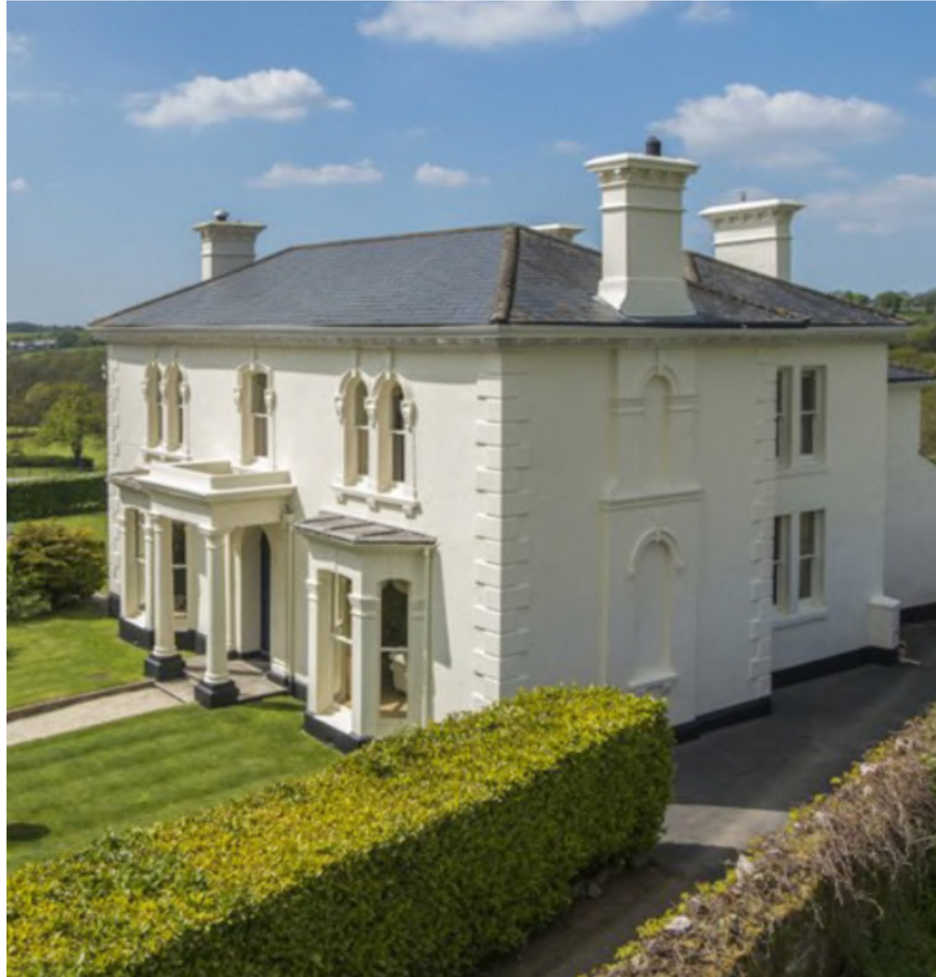
Precedent images of property examples containing similar architectural features which have been incorporated into the proposal
