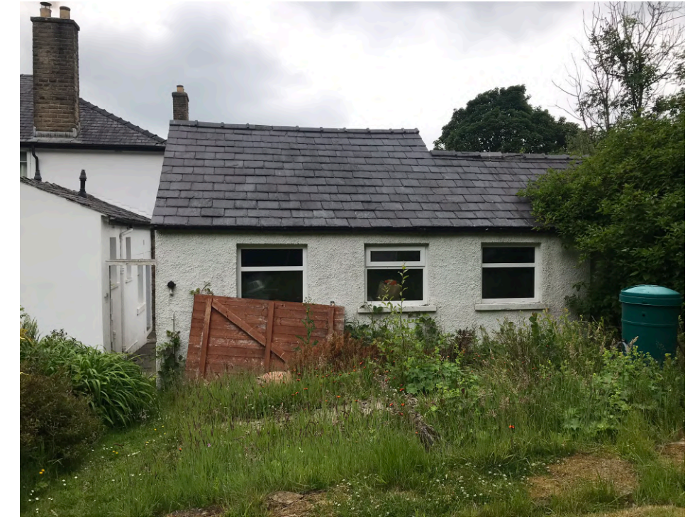
Rear elevation of out-building 1
