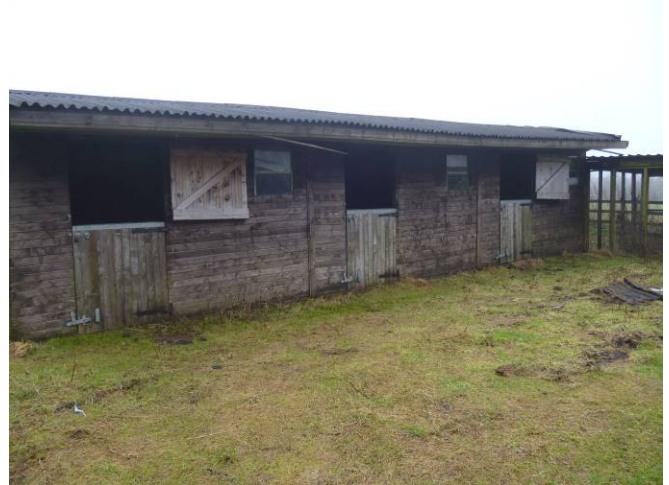
Timber stables with negligible bat roost potential.
