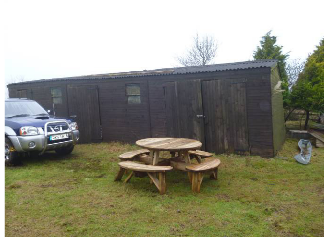
Timber stables with negligible bat roost potential.
