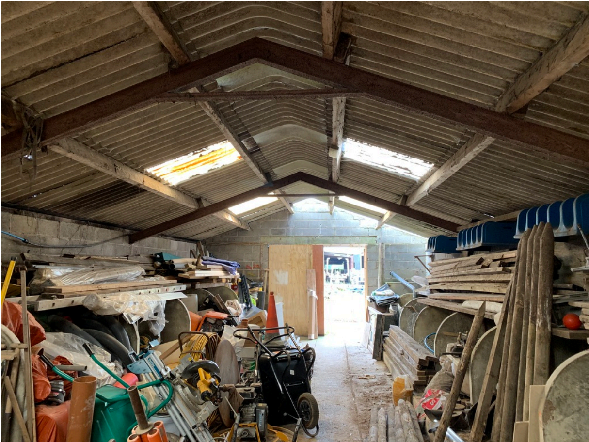
Photo 13 – Internal looking west
