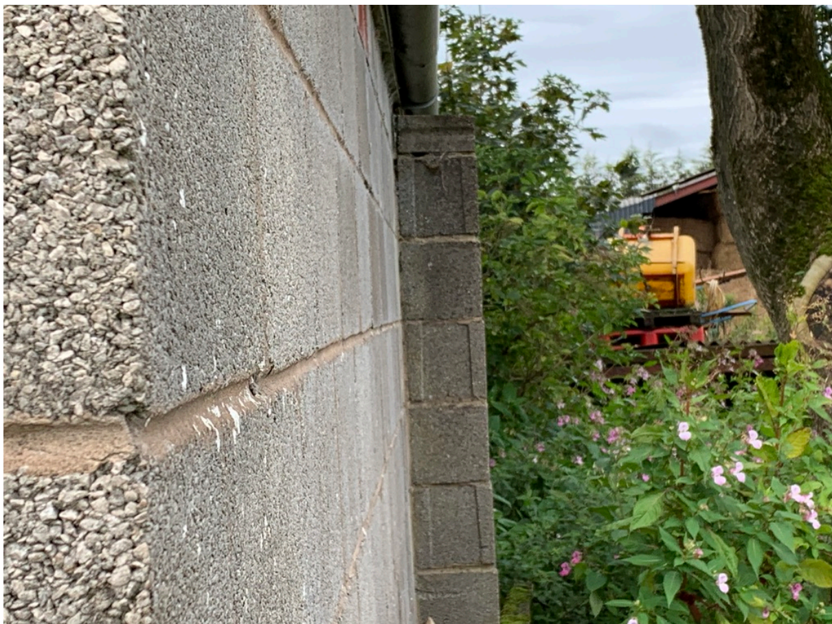
Photo 8 – North Elevation – pier/buttress
