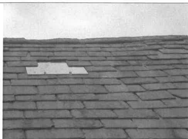
Photo 11: Gaps beneath ridge copings at B2
