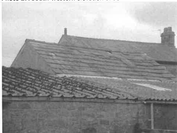
Photo 29: Stone tile roof of B5 and corrugated sheet covered roofs at B4 (left) and B5a (right)
