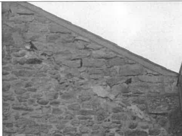
Photo 18: Gaps in the stone wall at the south-eastern elevation of B3
