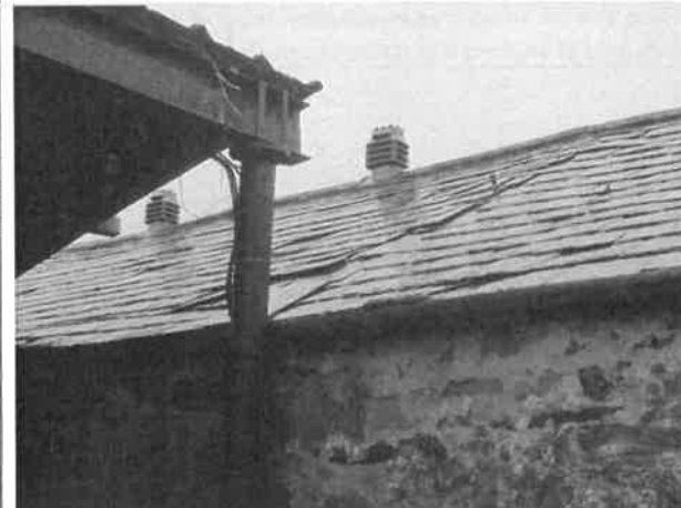
Photo 10: Gaps beneath slates at B2
