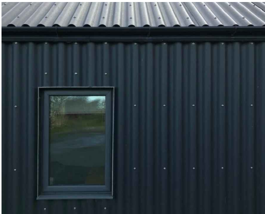
corrugated cladding and roofing to the garage
