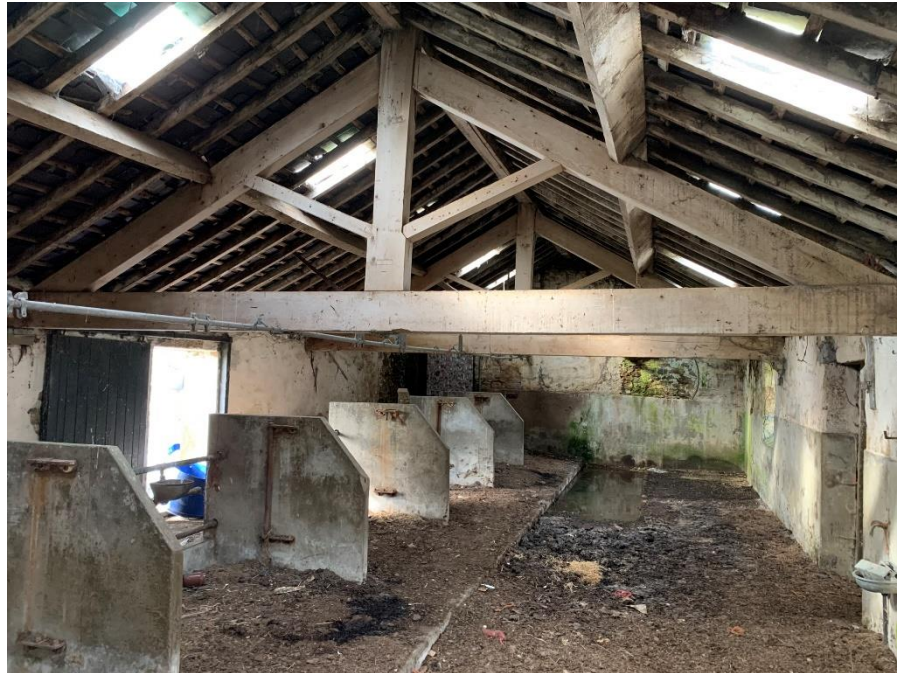
9) Single storey barn roof trusses
