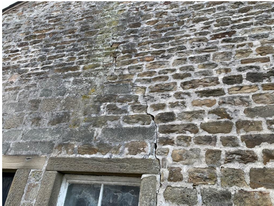
2) Minor cracking above window.
