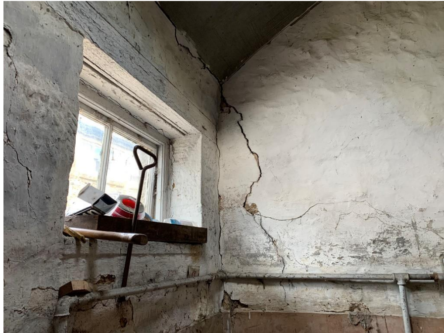
11) Internal cracking front elevation of outbuilding
