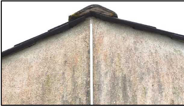
View showing sealed roof edges (lhs) and roof covering with occasional gaps present between slates (rhs)
