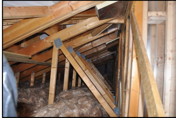
View of roof void, showing modern liner, truss supports and rock wool
