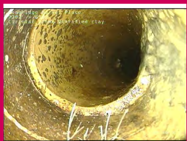
14, 00:07:22, 38.38 m Defective junction, damaged at 3 o'clock, diameter: 150mm
