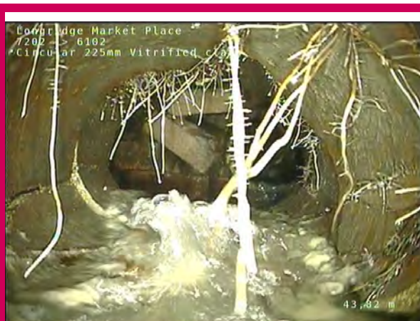
15, 00:08:19, 43.78 m Broken pipe from 3 o'clock to 9 o'clock
