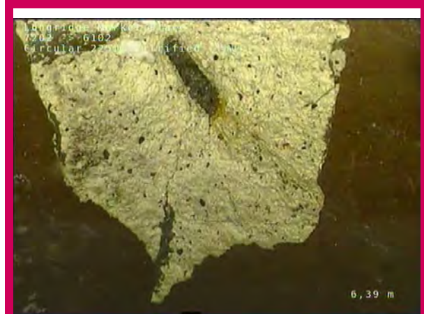
2, 00:01:05, 6.39 m Hole in drain or sewer at 3 o'clock
