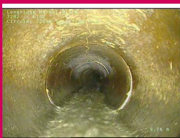
1, 00:00:10, 0.76 m Crack, longitudinal at 12 o'clock, start
