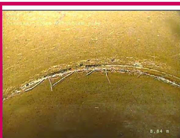
5, 00:01:59, 8.84 m Roots, fine at joint
