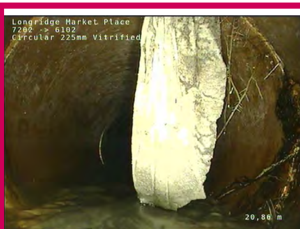
9, 00:04:33, 20.83 m Other obstacles at joint from 11 o'clock to 1 o'clock, 10% cross-sectional area loss, Rag
