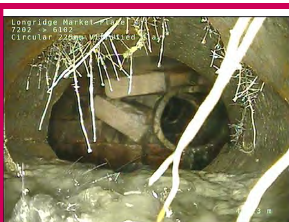
17, 00:08:36, 44.23 m Fracture, longitudinal at joint at 12 o'clock
