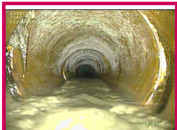
12, 00:06:03, 28.49 m Other obstacles at joint at 10 o'clock, 10% cross-sectional area loss, Rag
