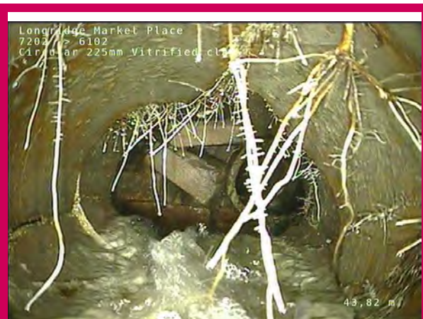
16, 00:08:26, 43.82 m Deformed drain or sewer, 10%
