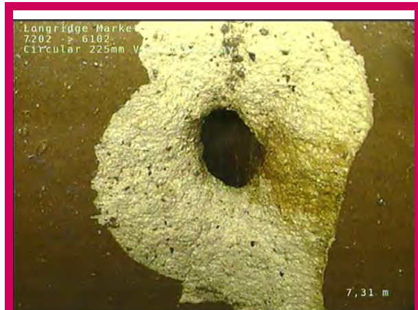
4, 00:01:33, 7.31 m Hole in drain or sewer at 2 o'clock
