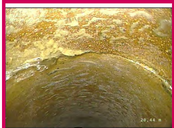
8, 00:04:03, 20.44 m Infiltration, running at joint at 11 o'clock
