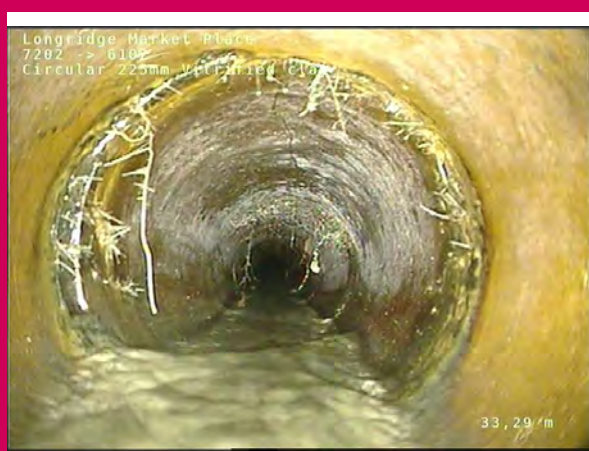
13, 00:06:42, 33.29 m Roots, fine at joint, start
