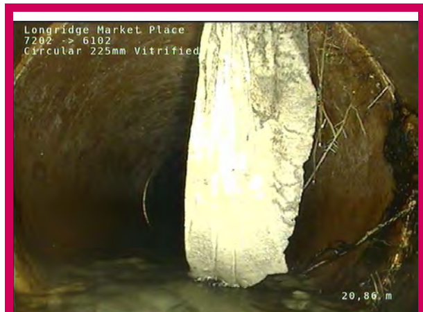
10, 00:04:28, 20.86 m Roots, fine at joint
