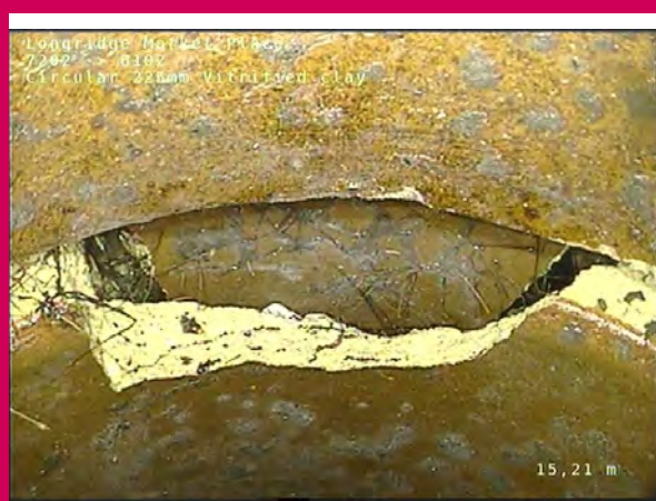
7, 00:02:56, 15.21 m Hole in drain or sewer from 11 o'clock to 1 o'clock
