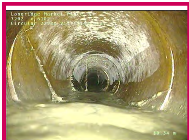
6, 00:02:16, 10.34 m Roots, fine at joint, start
