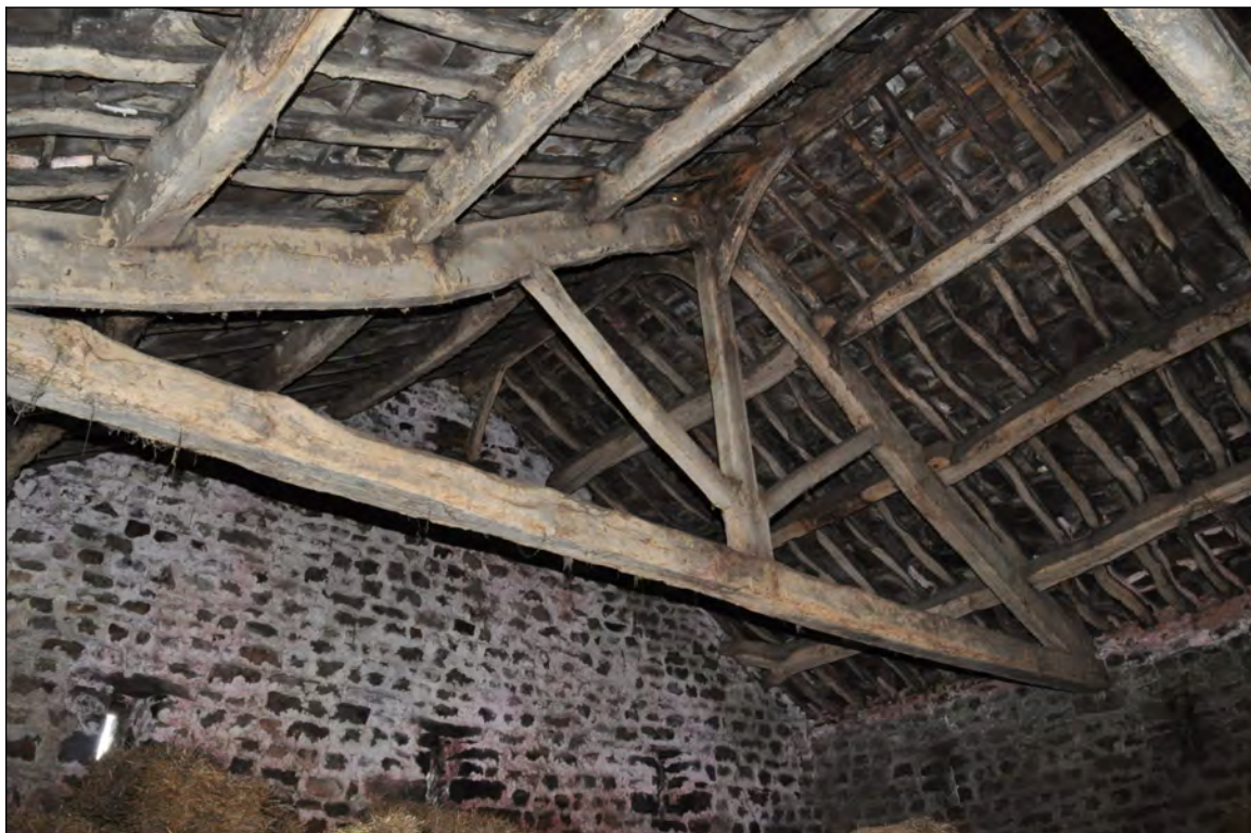
Photo 6: Roof structure over hayloft
