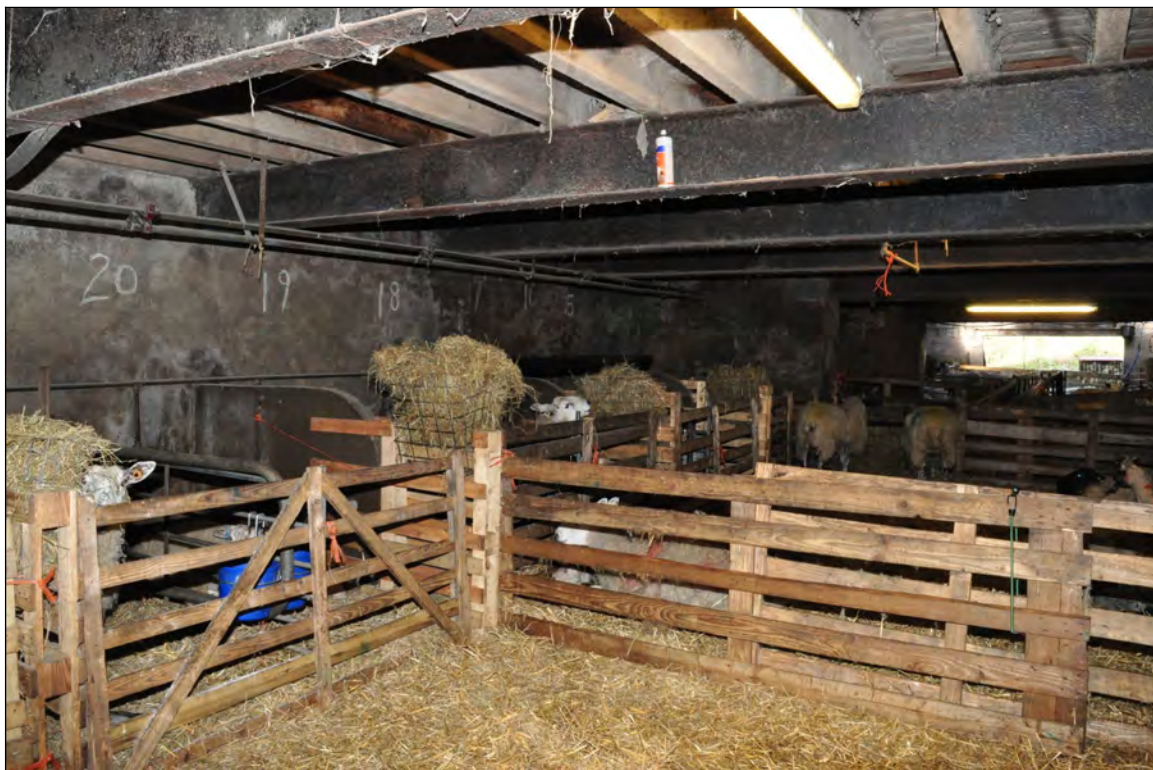
Photo 5: Ground floor. Entirely modern in character
