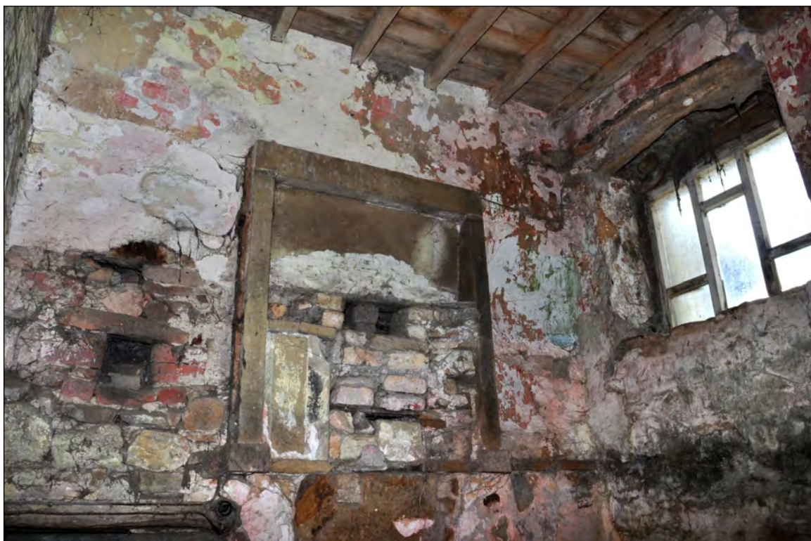
Photo 8: Fireplace and attic floor above, within domestic extension
