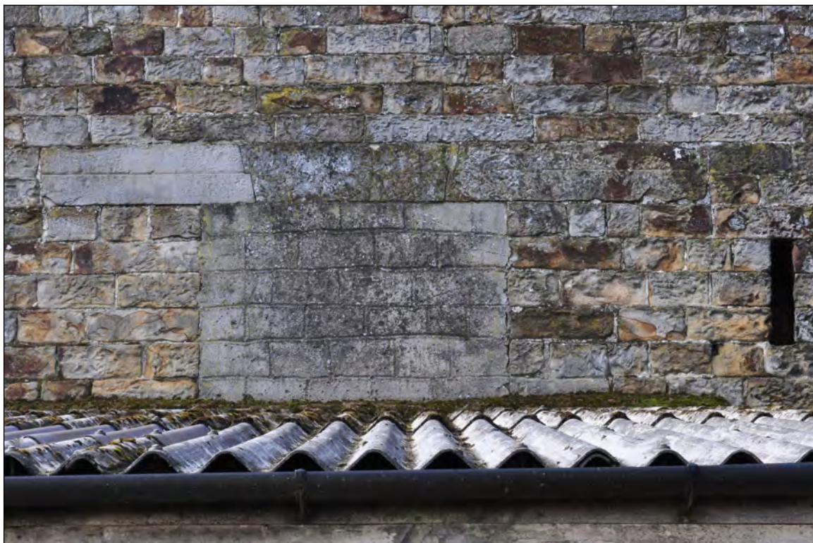
Photo 3: Blocked winnowing door to hayloft in north-east side, with distinctive lintel
