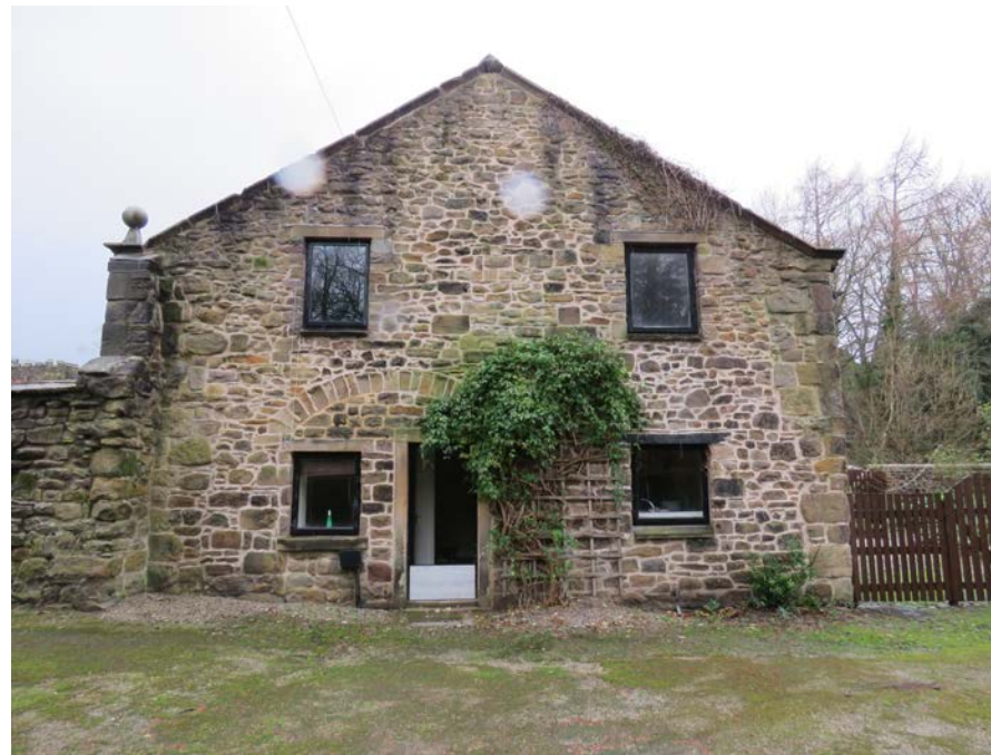
Existing south elevation of Whalley Lodge.
