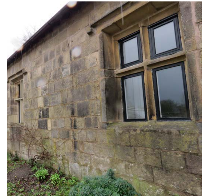
Existing west facade of Whalley Lodge.
