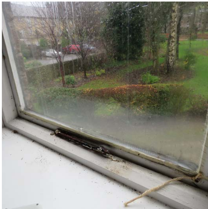
Existing condition of first floor windows.
