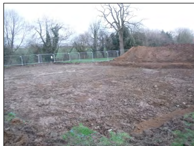
Open area, looking NW.
