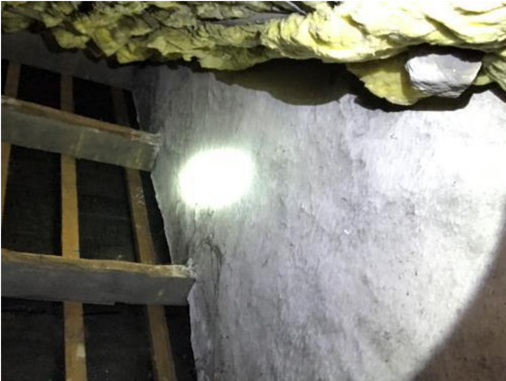
Plate 11 – Internal character of the loft space viewed via a loft hatch
