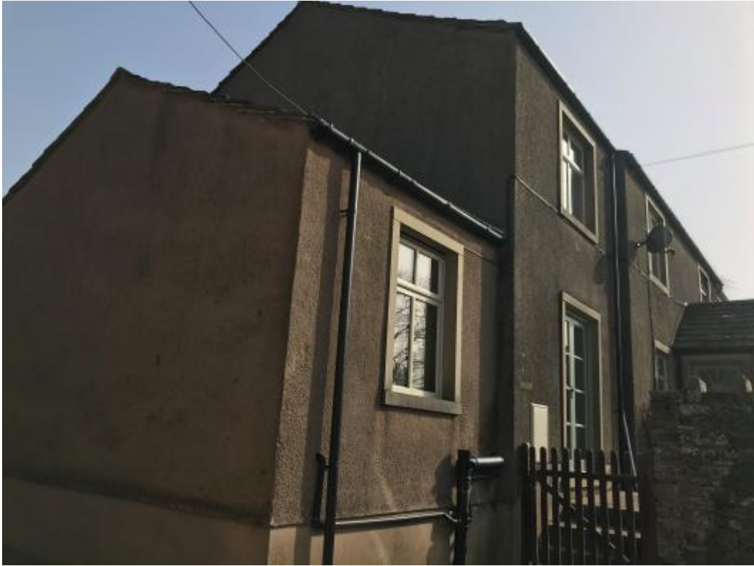
Plate 4 – Western elevation with existing single-storey entrance way
