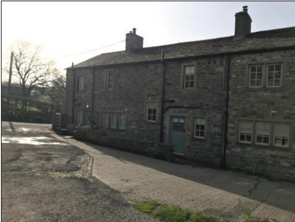
Figure 7.1 – The front elevation of the disused dwelling
