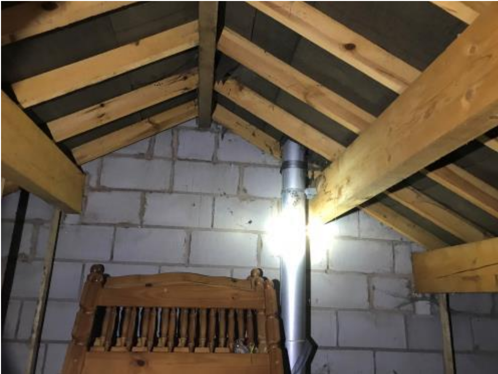
Plate 10 – Internal character of the fully accessible loft space
