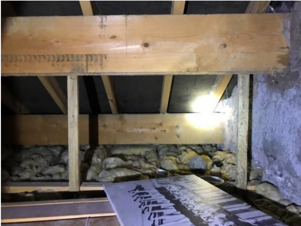
Plate 9 – Internal character of the fully accessible loft space
