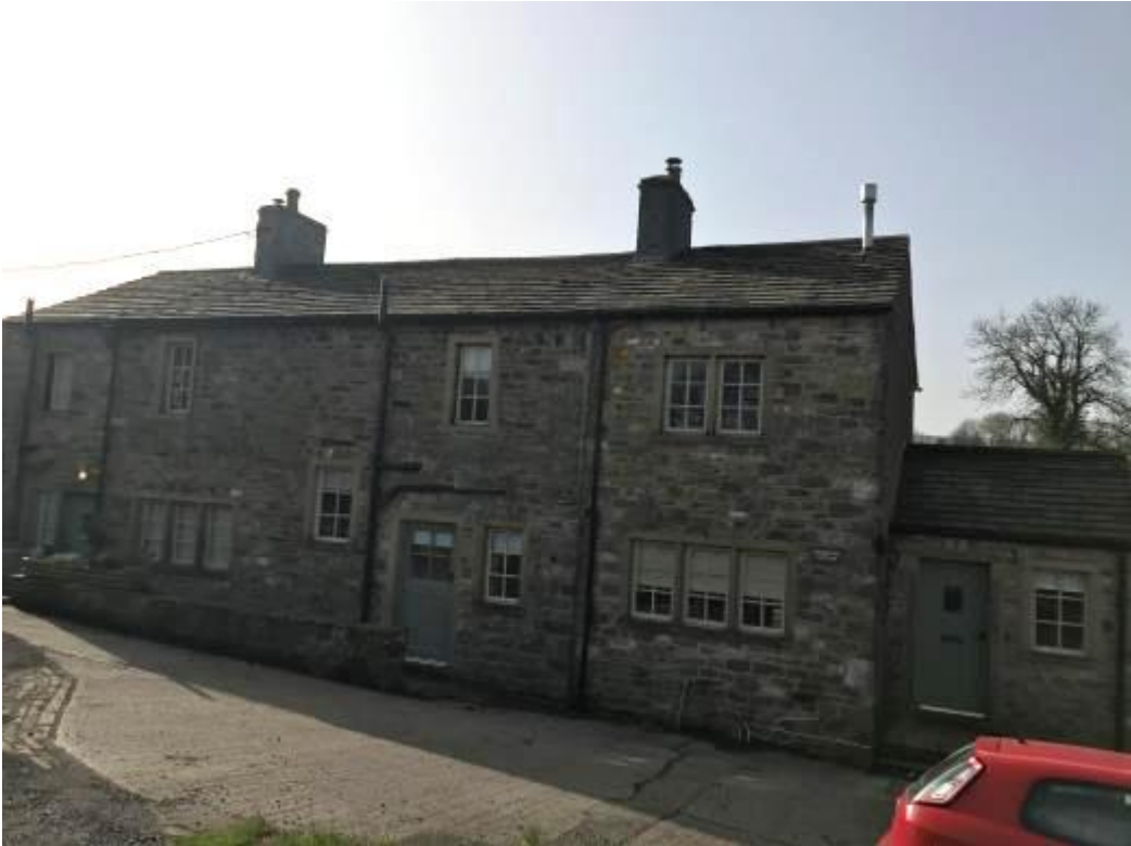
Plate 1 – Northern elevation of Bridge End Cottage
