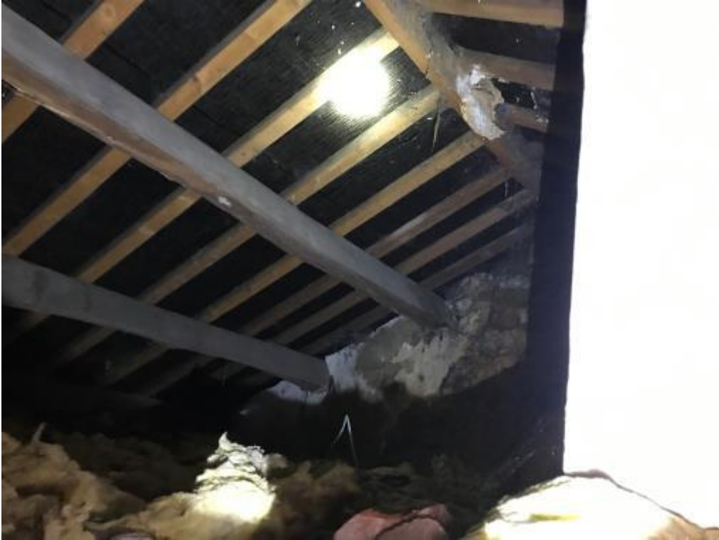
Plate 10 – Internal character of the loft space viewed via a loft hatch
