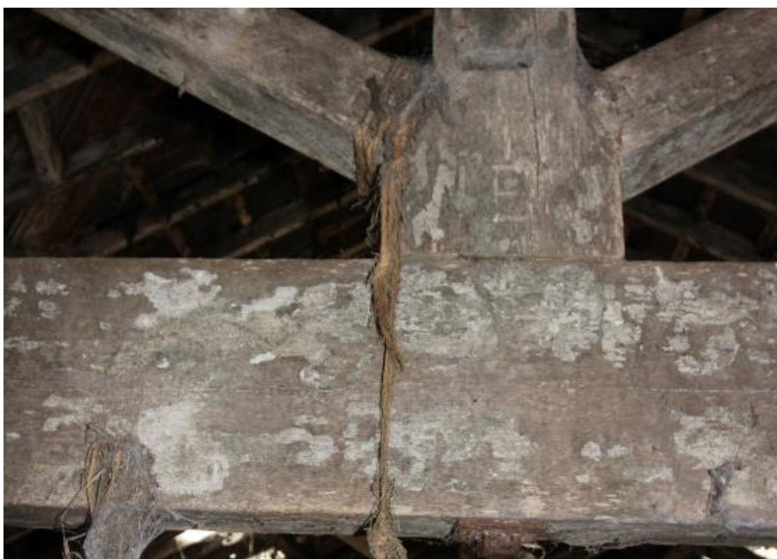
Plate 74: Inscribed letter 'B' at base of King-post truss
