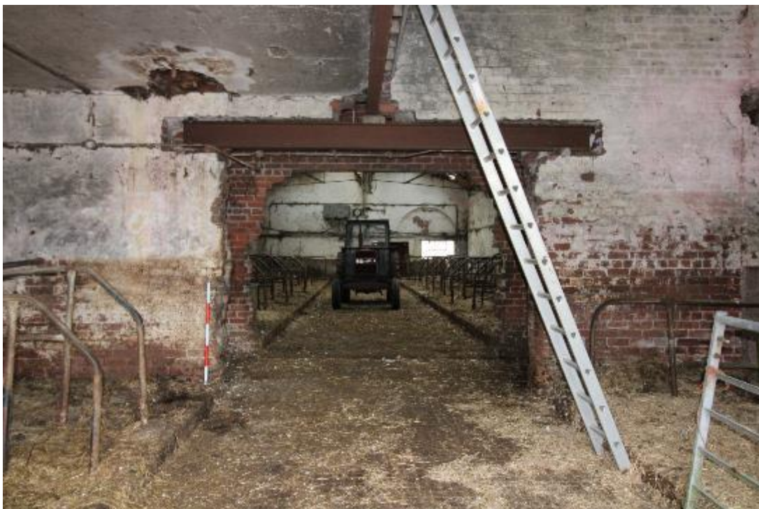
Plate 20: Knocked-through entrance into the converted Covered Yard
