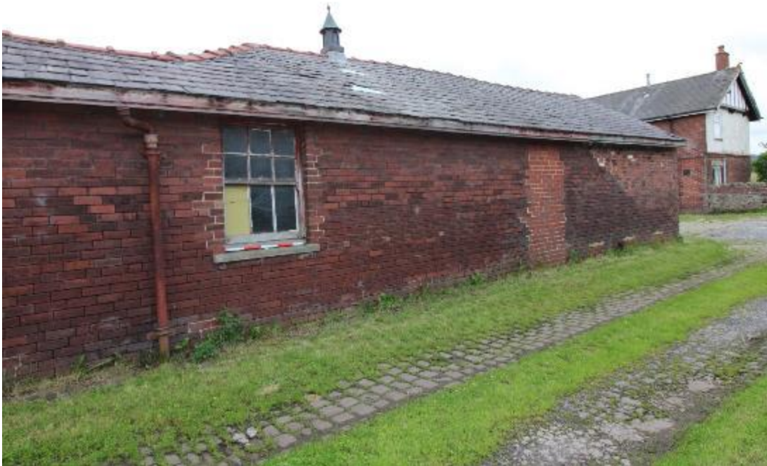
Plate 36: Inserted window, with blocked doorway to right, 1m scale
