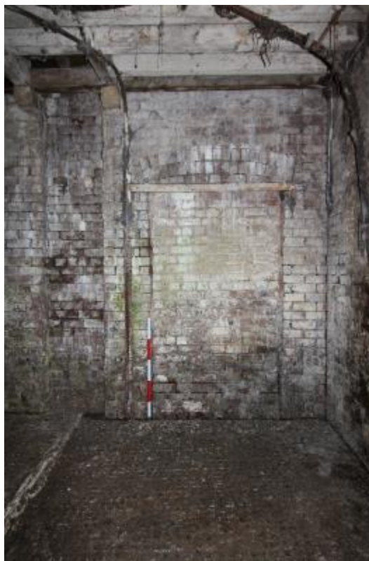
Plate 70: Blocked doorway at northern end of western wall, with 1m scale. Note vertical channel to the left of frame
