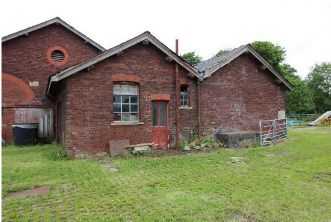
Plate 26: Eastern end of the southern elevation, showing inserted doorway to WC
