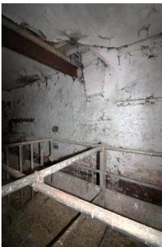
Plate 59: Corbelled brick flue on western wall of eastern cell
