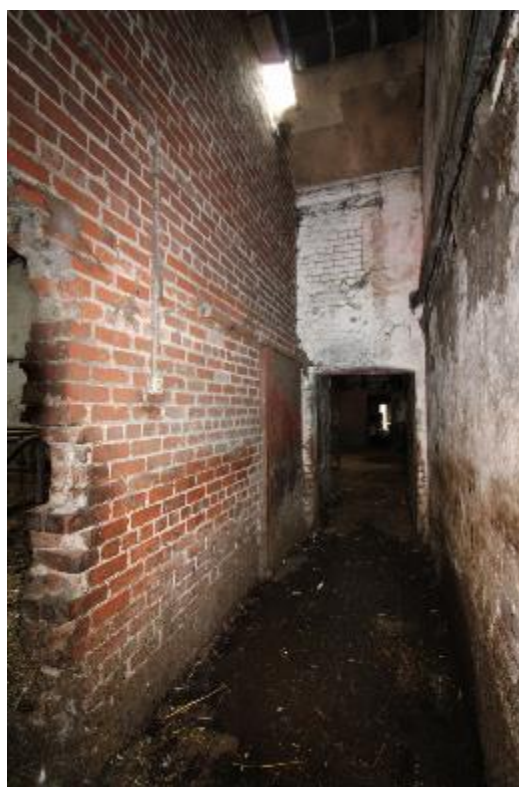
Plate 49: Blocked clerestory window above the door, with later wall to left of frame
