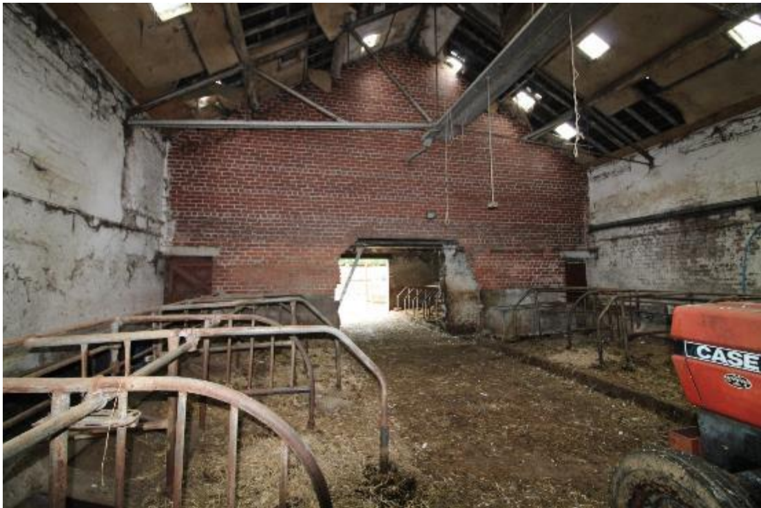
Plate 46: Northern wall of Covered Yard, with later knocked-through central opening
