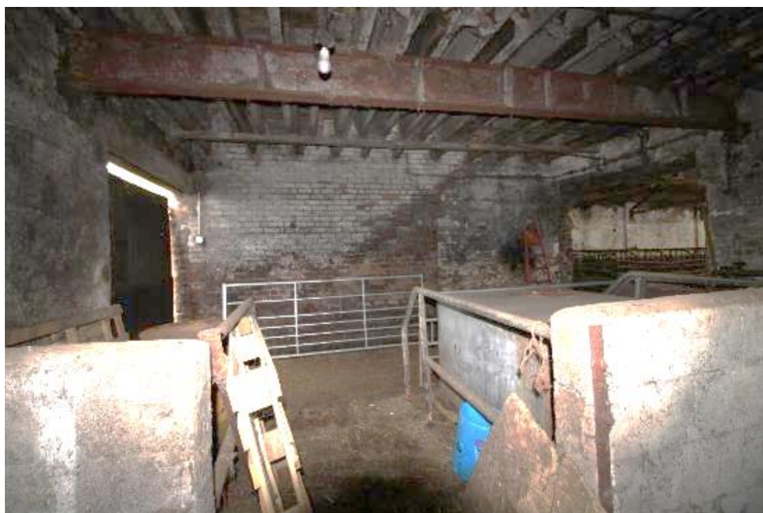
Plate 65: Root House, showing diagonal staircase scar on the eastern wall, facing east
