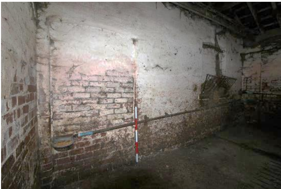
Plate 95: Blocked openings, formerly opening on to the Central Shippon, with 1m scale
