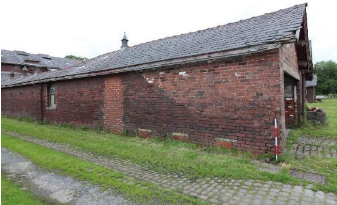
Plate 37: Southern end of western elevation, with 1m scale. Note the infilled apertures at the base of the wall (to the fowl houses labelled in Plate 7)
