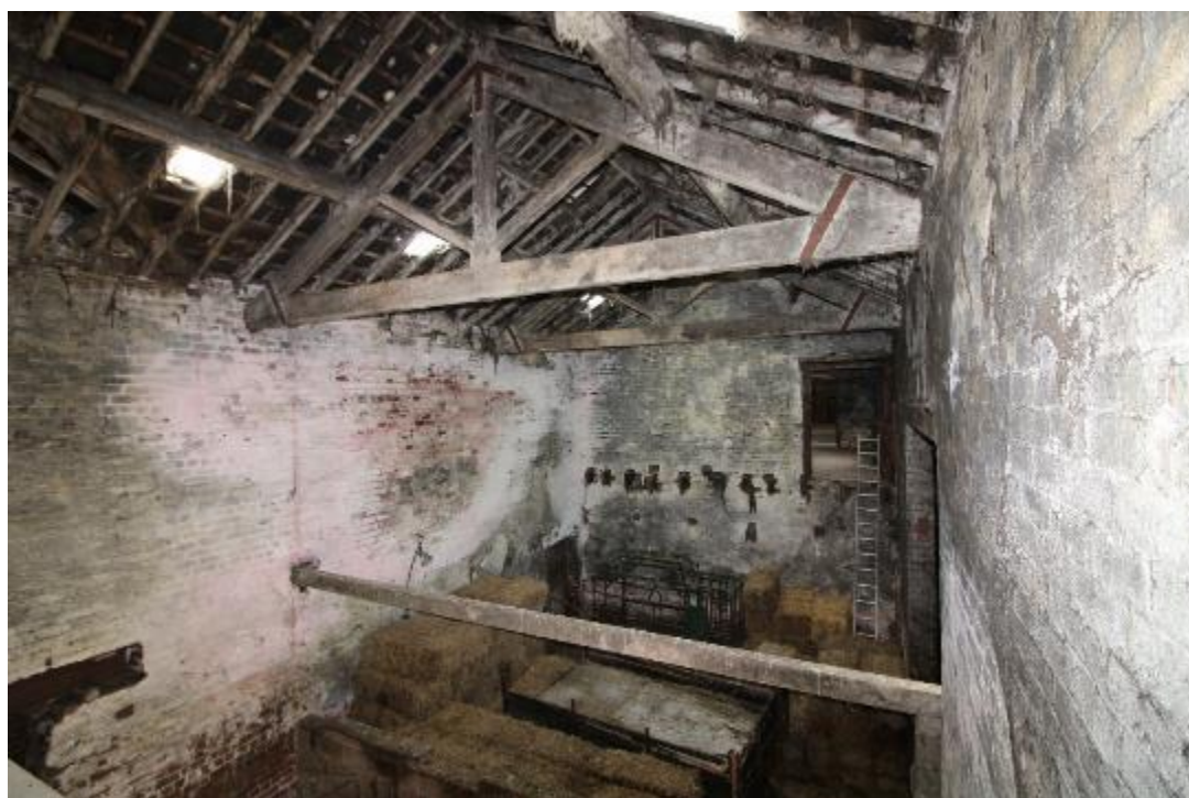
Plate 63: Barn, facing west, note the first-floor doorway to right of frame and truncated floor beams to left
