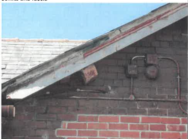
Photo 11: Gaps beneath the slates at the roof verge on southern elevation
