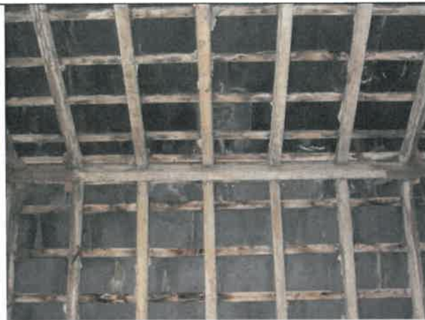
Photo 48: Rafters and cobweb free section of ridgeboard
