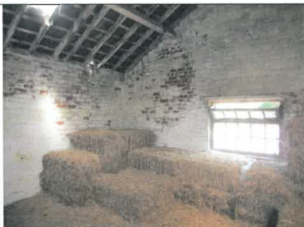
Photo 13: Interior of Section A showing mortared walls, underside of slates and skylights
