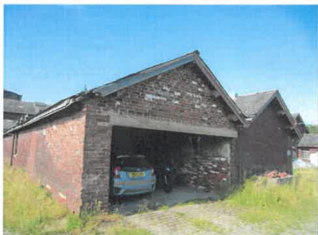
Photo 9: South-western corner (Section I) and damage to timber soffits and fascia
