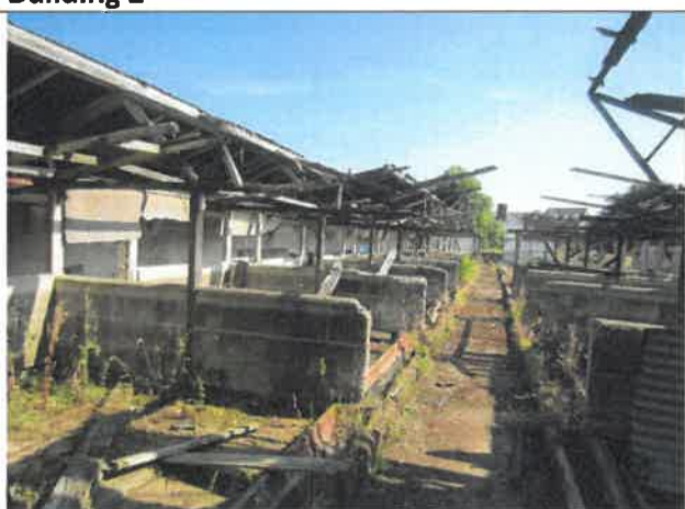
Photo 35: Damaged roof and exposed conditions
