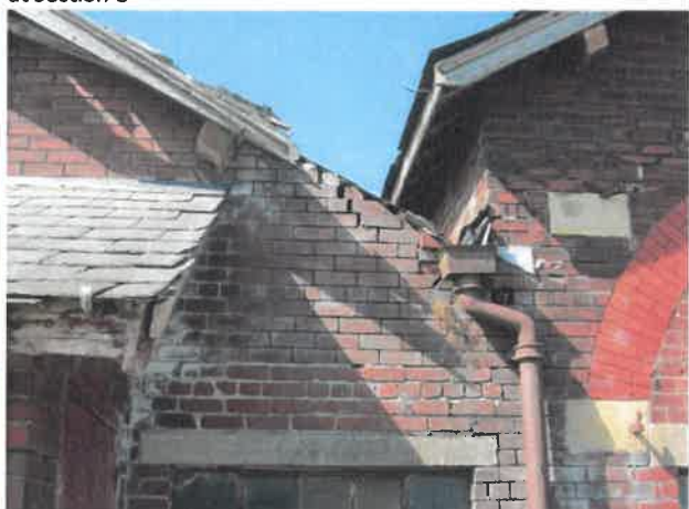
Photo 10: Gaps in brickwork at southern elevation
