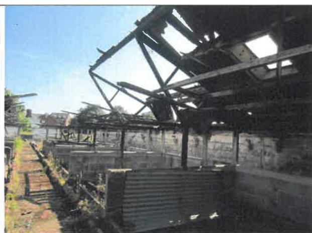
Photo 36: Damaged roof and exposed conditions
