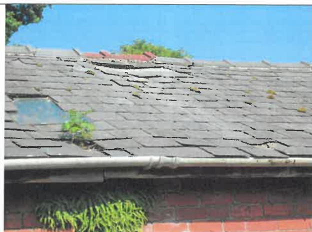
Photo 42: Gaps at the roof covering
