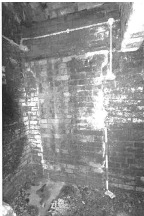
Plate 104: Blocked doorway at the northern end of the eastern wall, with 1m scale
