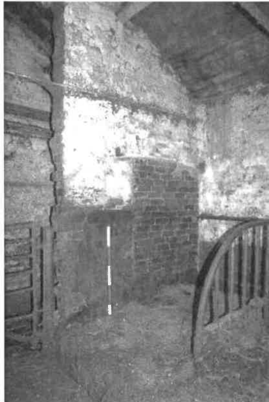
Plate 41: Blocked doorway in north-eastern corner of Shippon, with 1m scale
