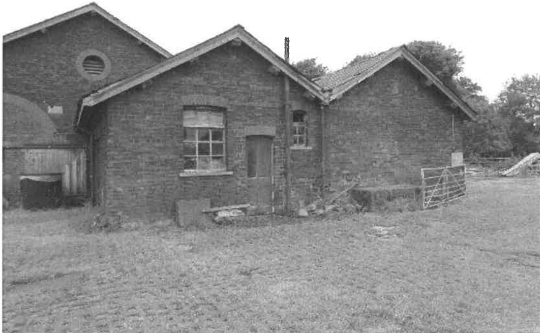
Plate 26: Eastern end of the southern elevation, showing inserted doorway to WC
