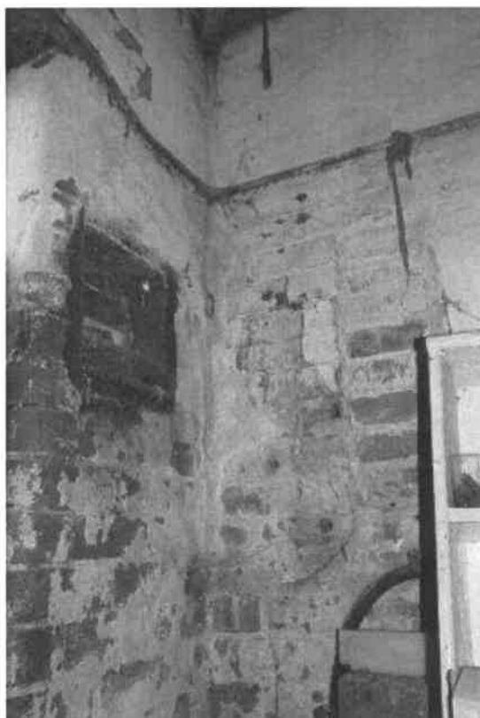
Plate 115: Bearing box and block aperture in north-western corner
