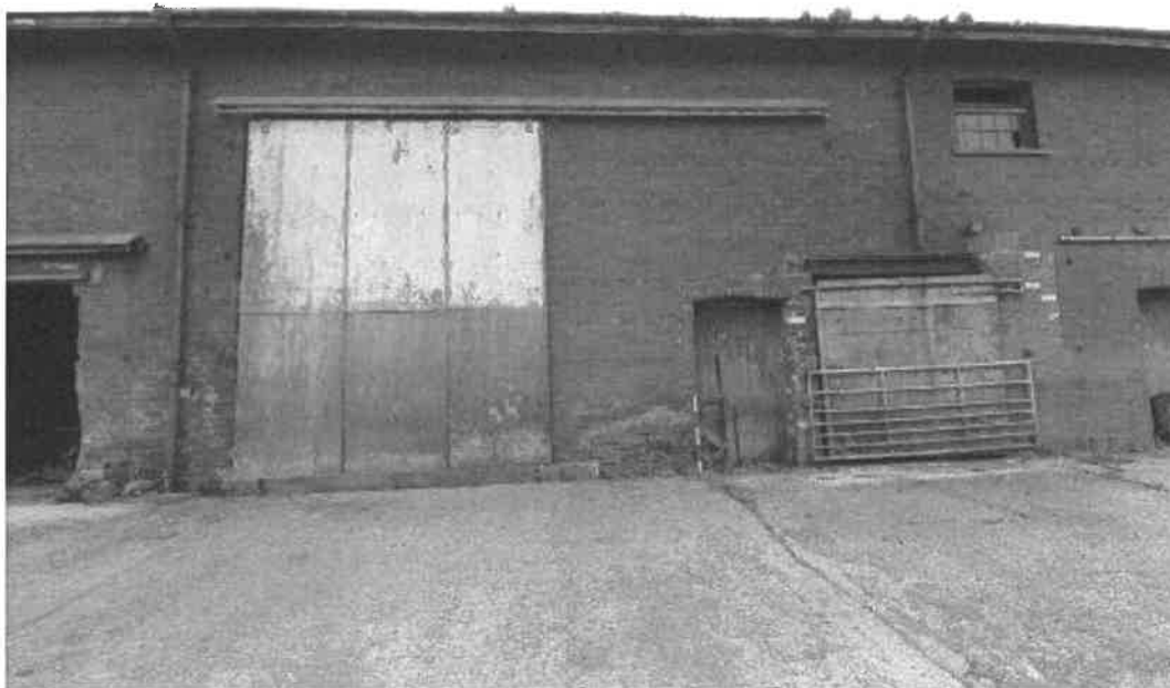
Plate 31: Two-storey sliding door at centre of the northern elevation
