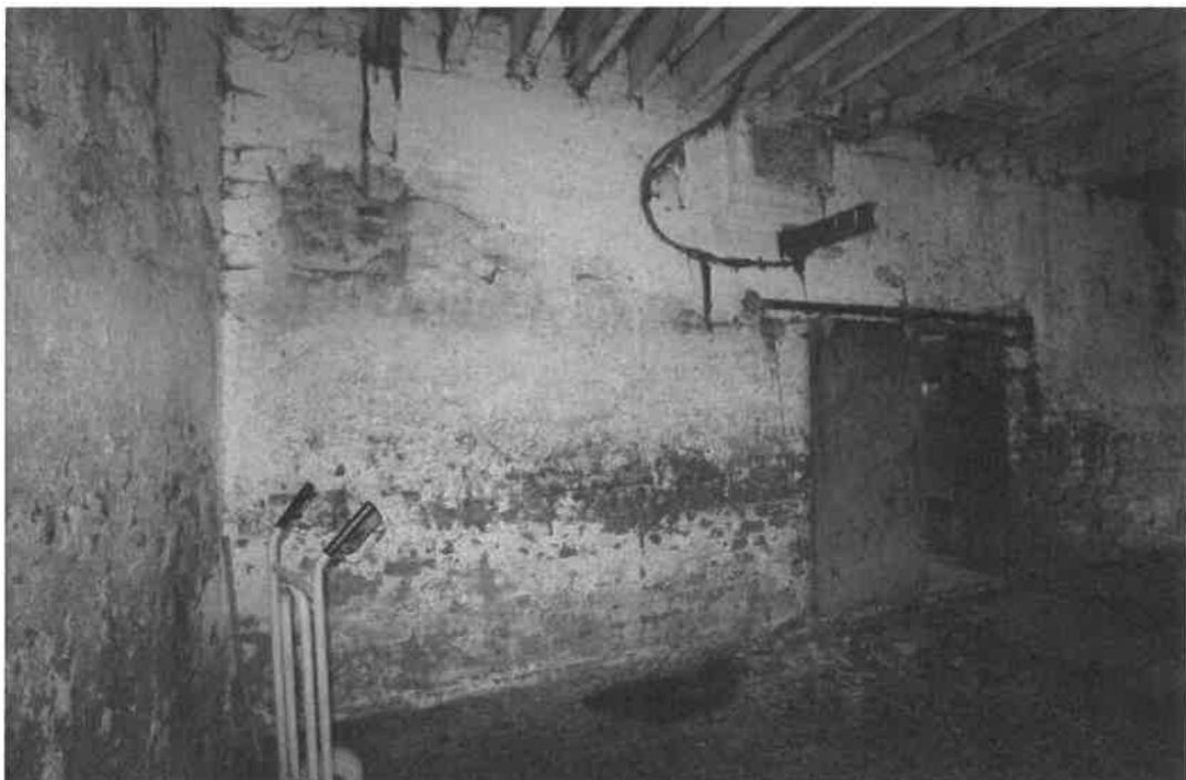
Plate 71: Southern entrance to the Milking Parlour with the ventilation aperture above and possible blocked bearing box to the left of frame
