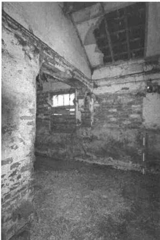
Plate 52: Blocked eastern doorway of northern passage, with widening doorway to left of frame
