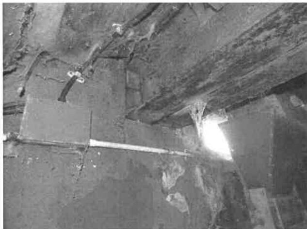
Image 47 – Surface corrosion
