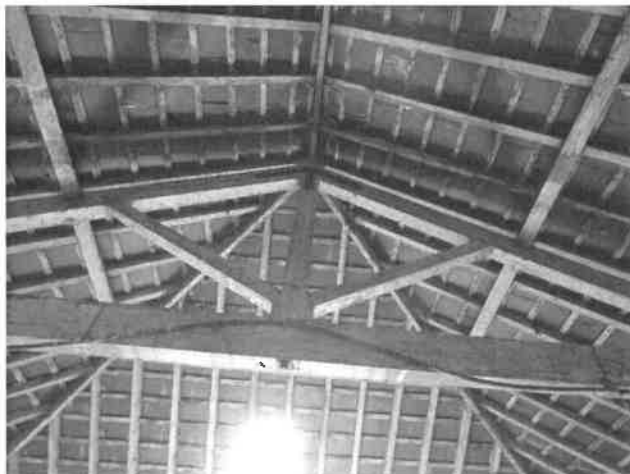
Image 23 – King Post Truss Roof Structure
