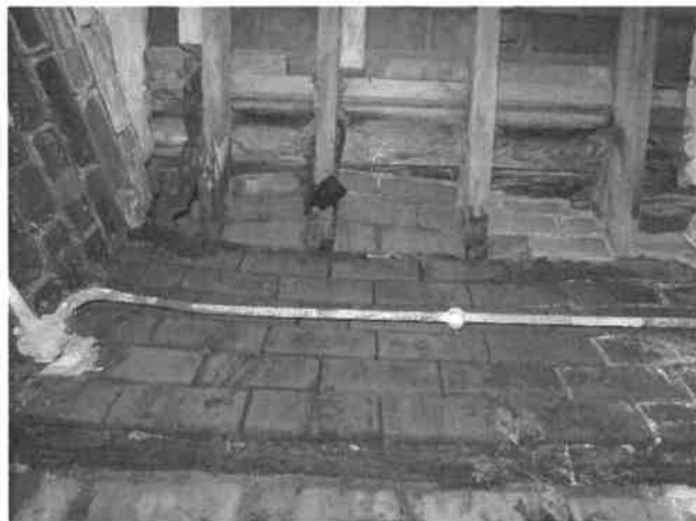
Image 35 – Minor movement/Water Ingress
