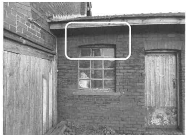
Image 66 – Cracking to defective brick arch
