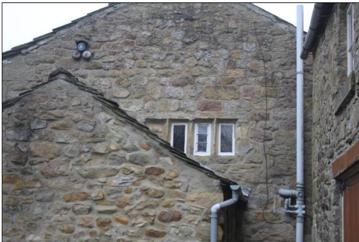
9. The 17 th century four-light window of the east gable is a crucial piece of evidence in the dating of the building
