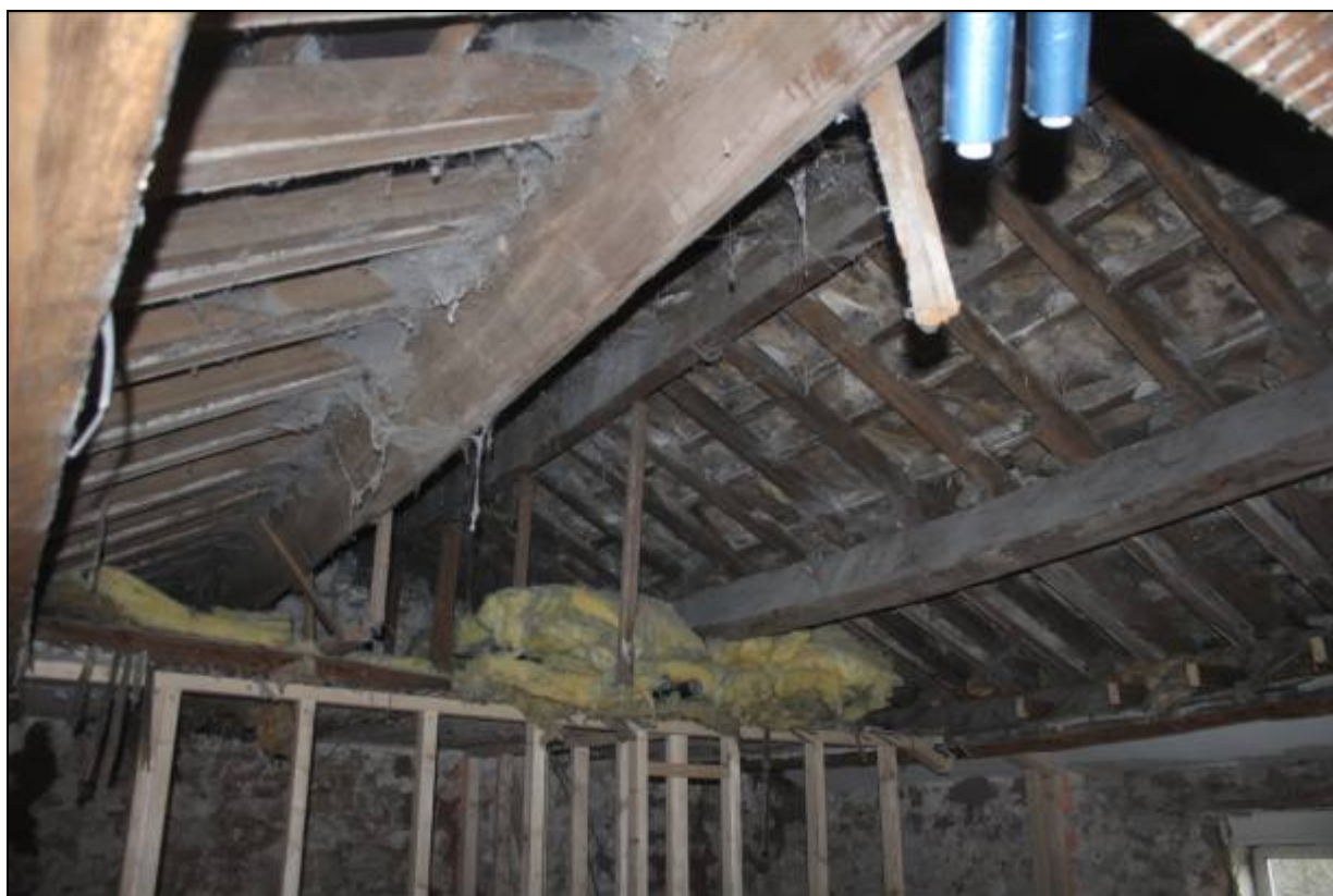
32. Roof above third bay
