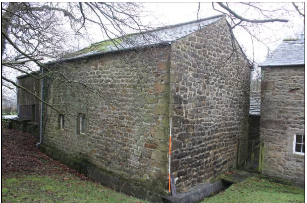
40. Rear of the former stable
