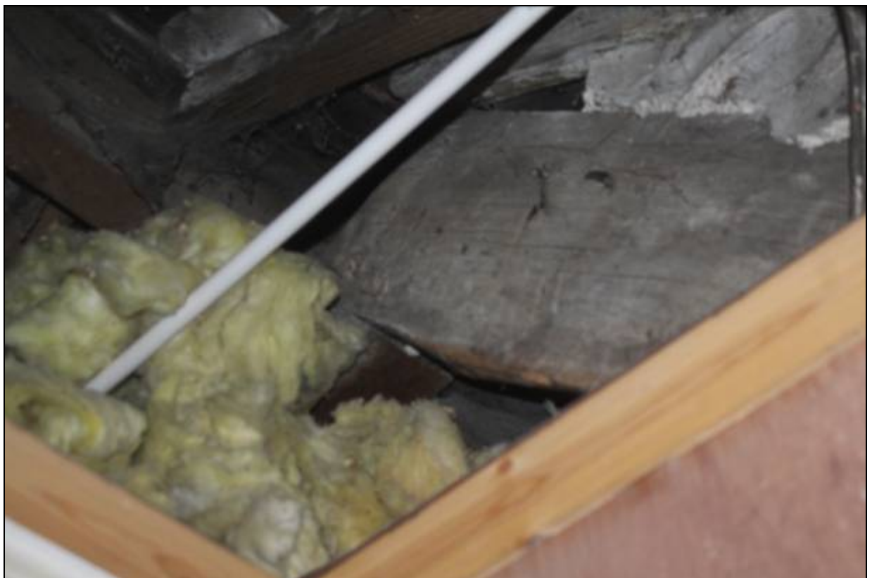
28. Apex of truss
