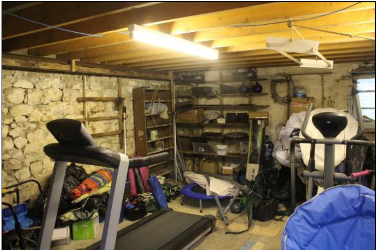
41. First bay of the garage
