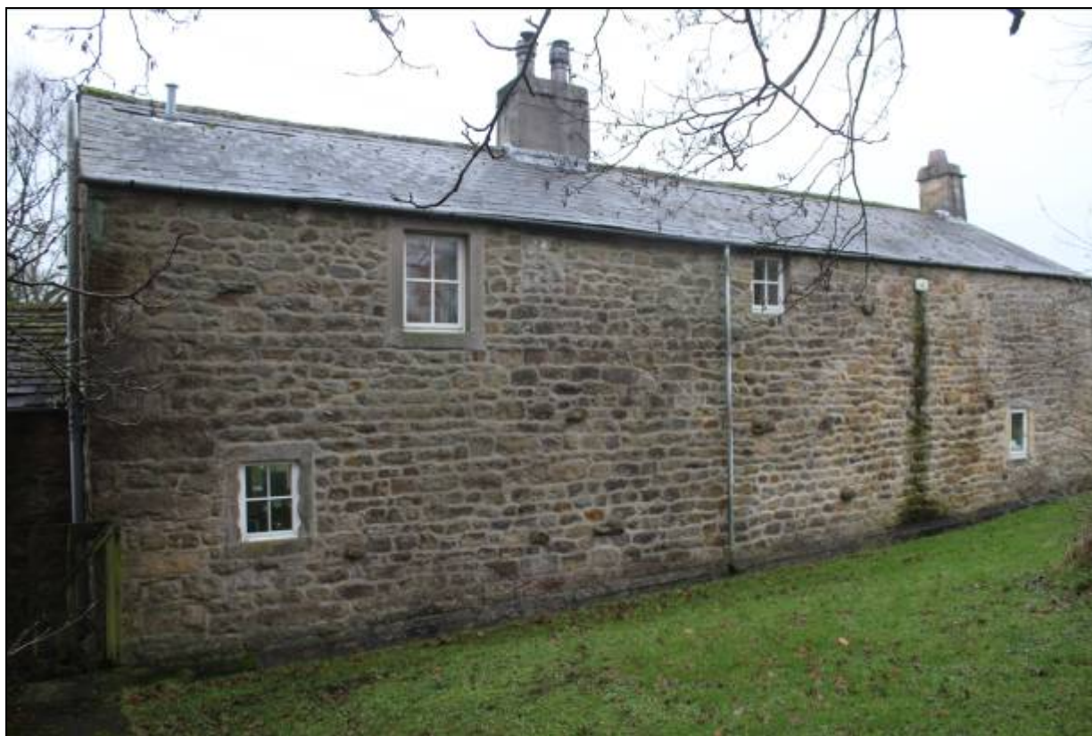
13. The plain north-facing rear of the main range
