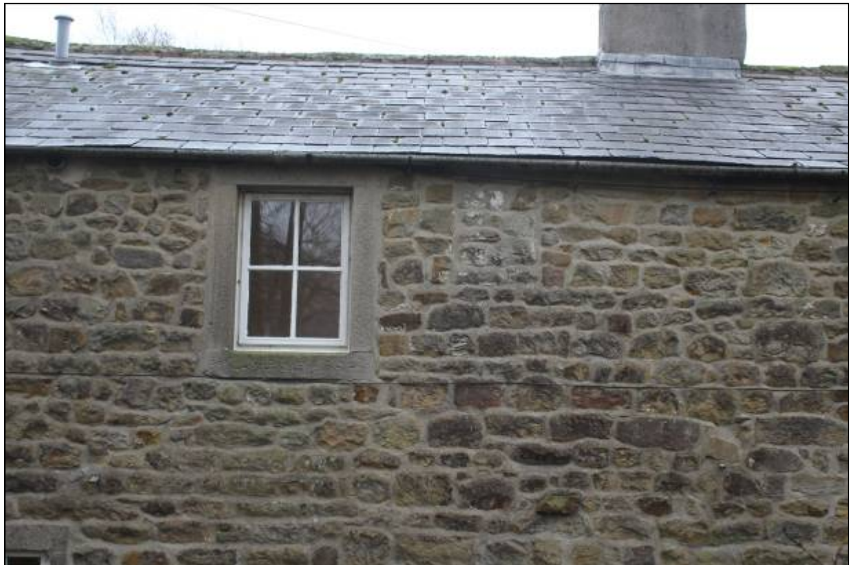
15. First floor window of third bay with blocked opening alongside
