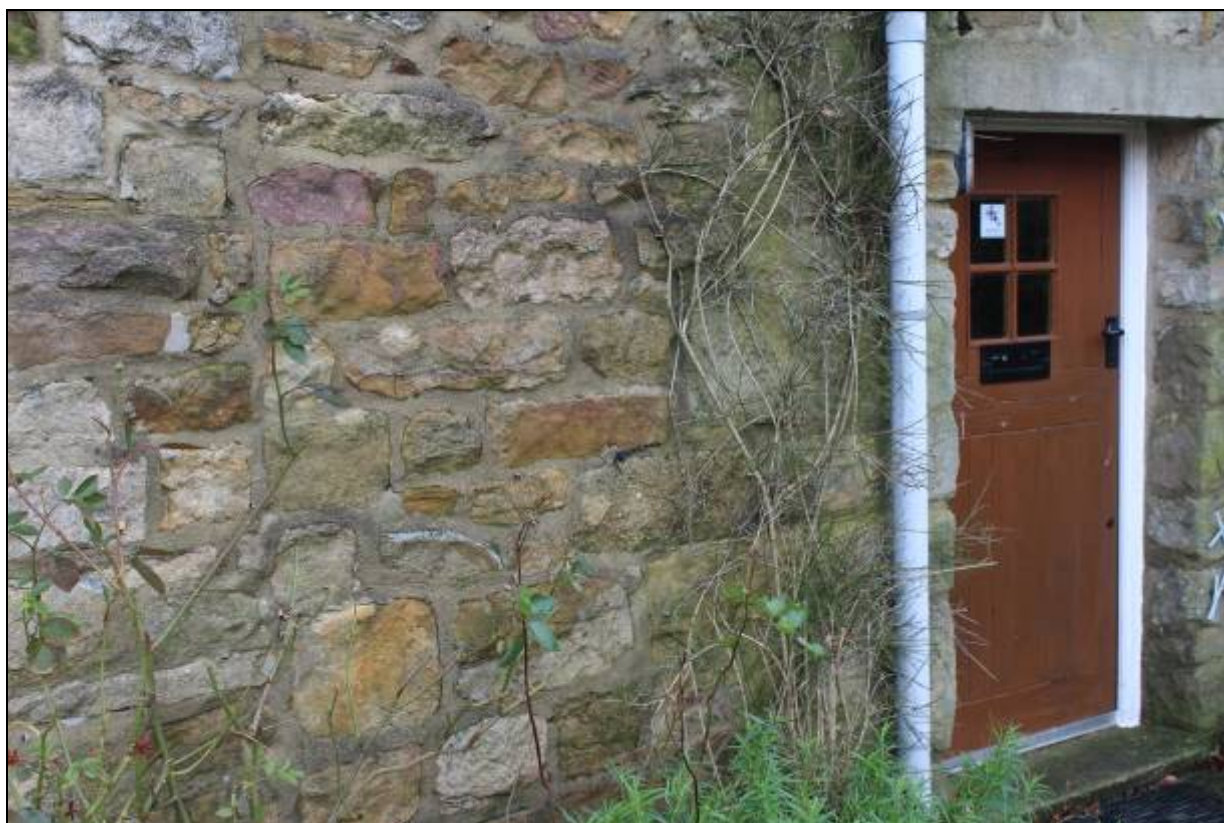
12. Evidence of possible blocked window at east end of main range
