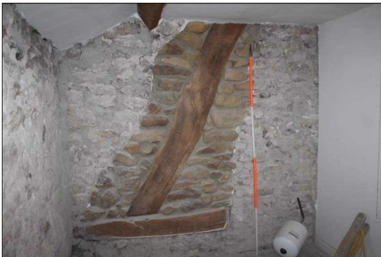
24. Southern blade, exposed within middle bedroom during renovation
