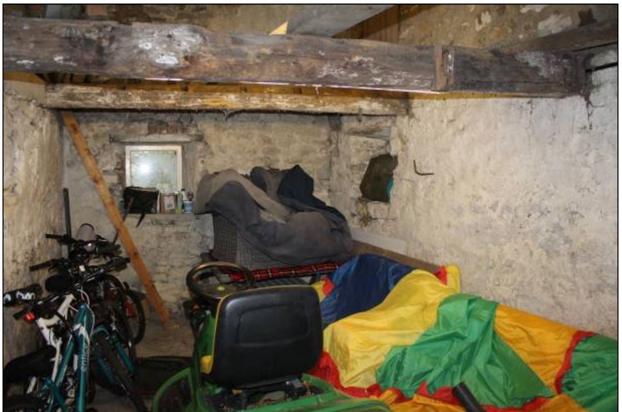
42. Second bay of the garage
