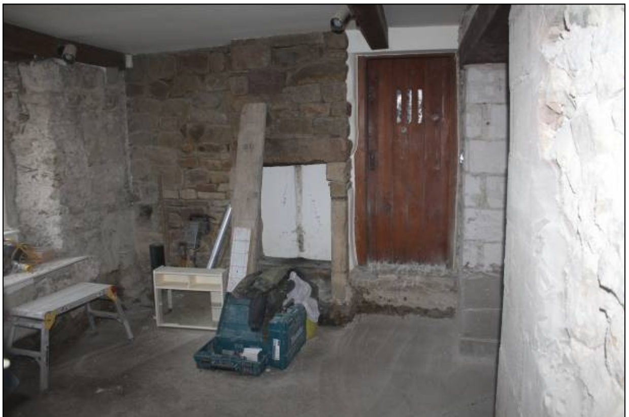
22. First bay during renovation, looking to ventilated door to outbuildings
