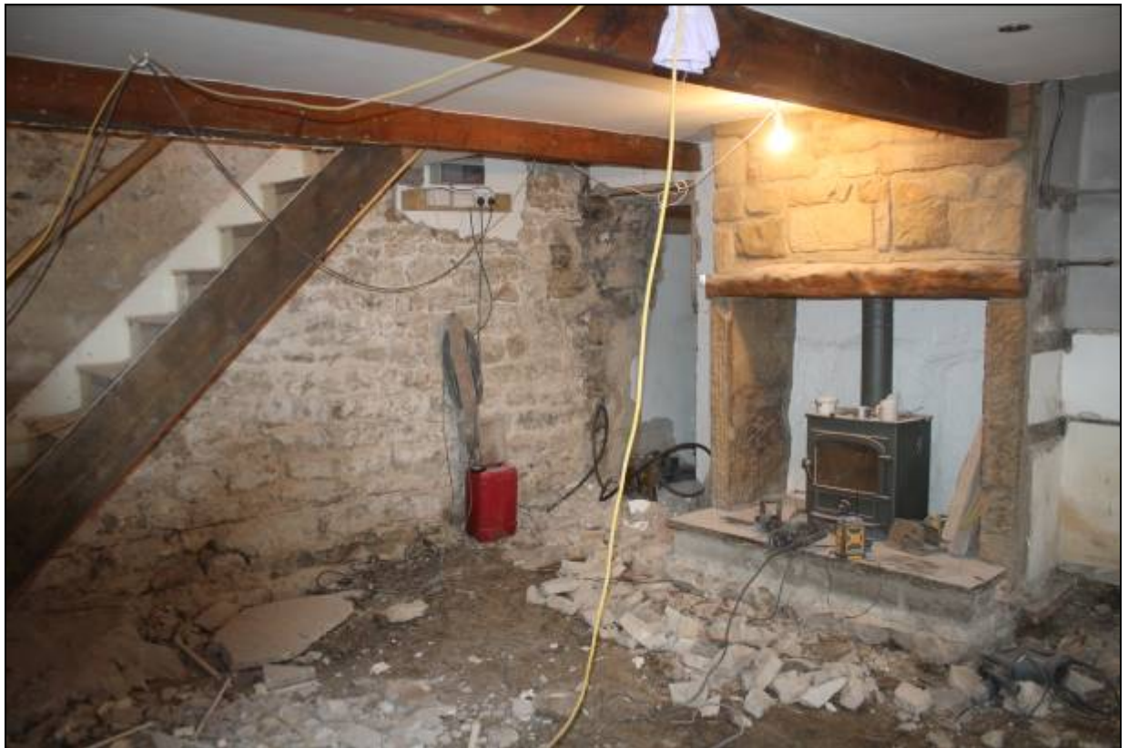
21. Housebody during renovation work
