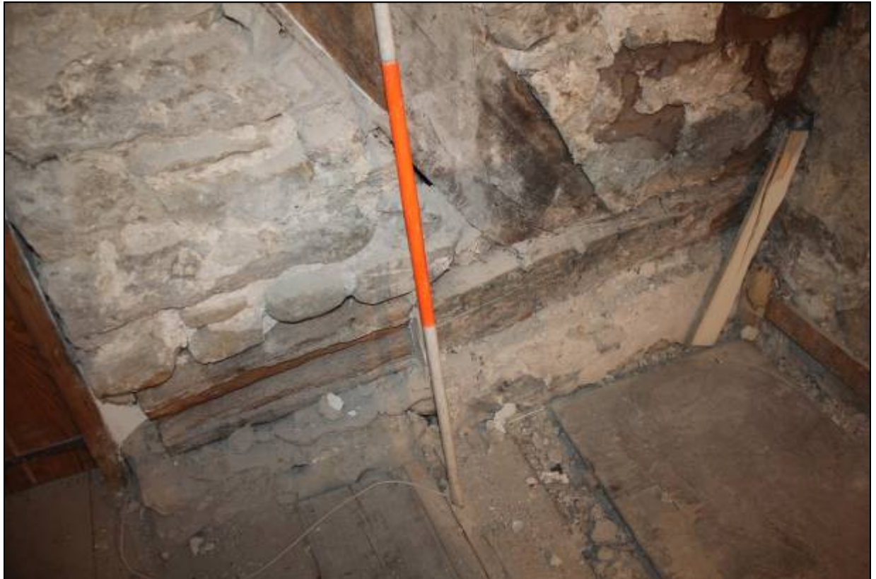
27. Termination of north blade
