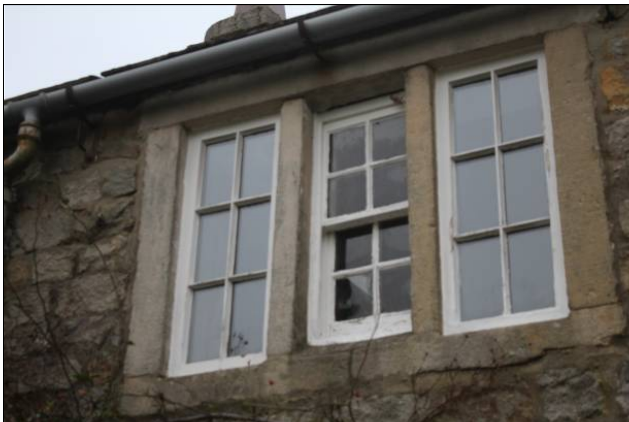
11. First floor window of the first bay, showing 19 th century centre light glazing and late 20 th century replacements in outer lights
