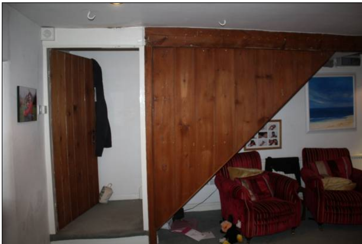
29. Staircase: its position in housebody is unlikely to be original
