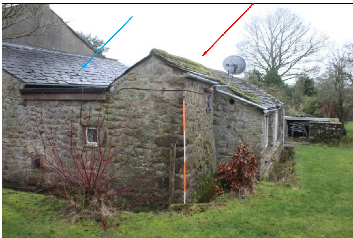
38. Rear of garden room, looking southwest, showing how it incorporates a small originally free-standing building, perhaps a privy (indicated by red arrow). To its left is the rear wall of the flat-roofed 1970s link (blue arrow)
