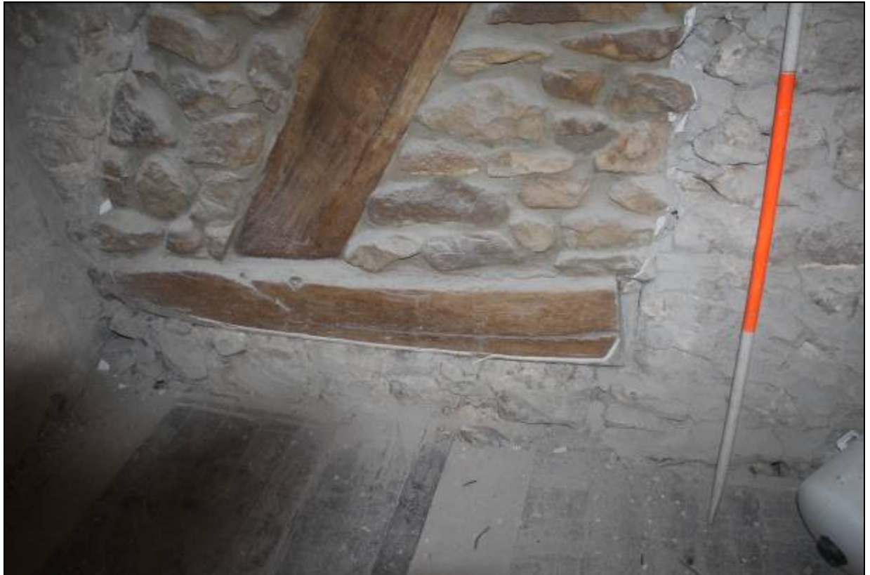
25. Truss is of upper cruck form, with blade terminating at tiebeam level
