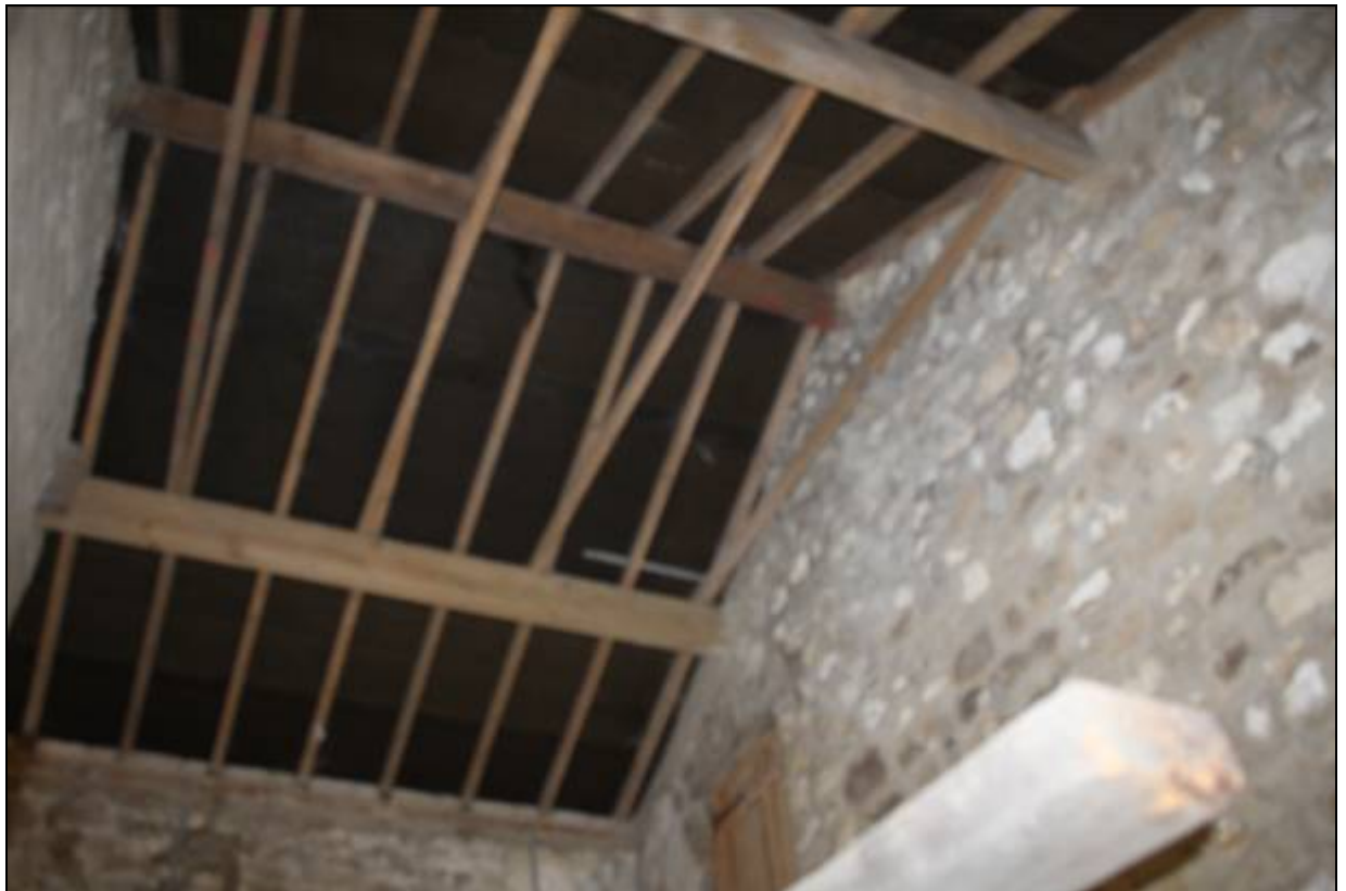
43. Renewed roof structure over garage
