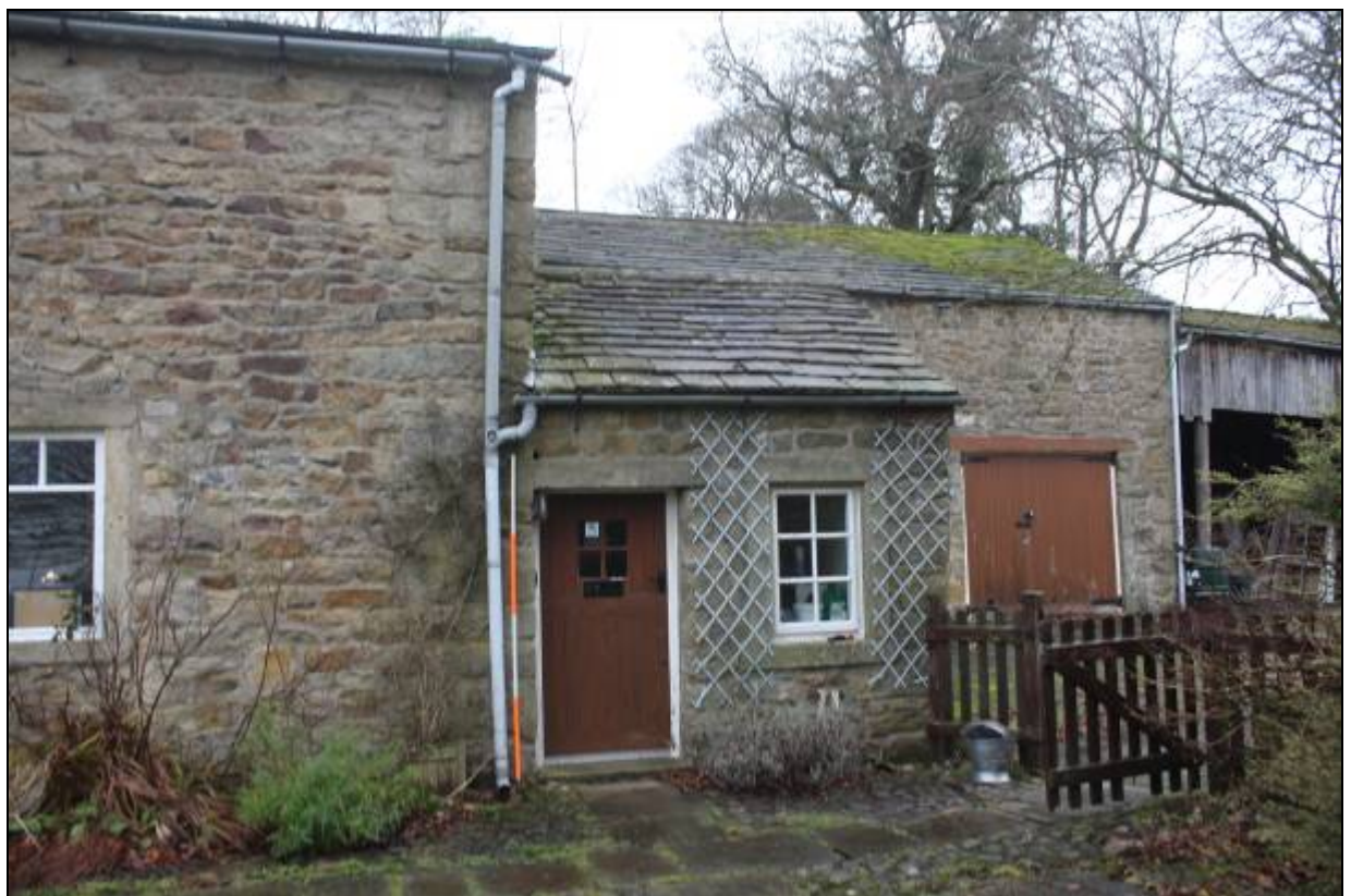
16. The single-storey porch, probably late 19 th century
