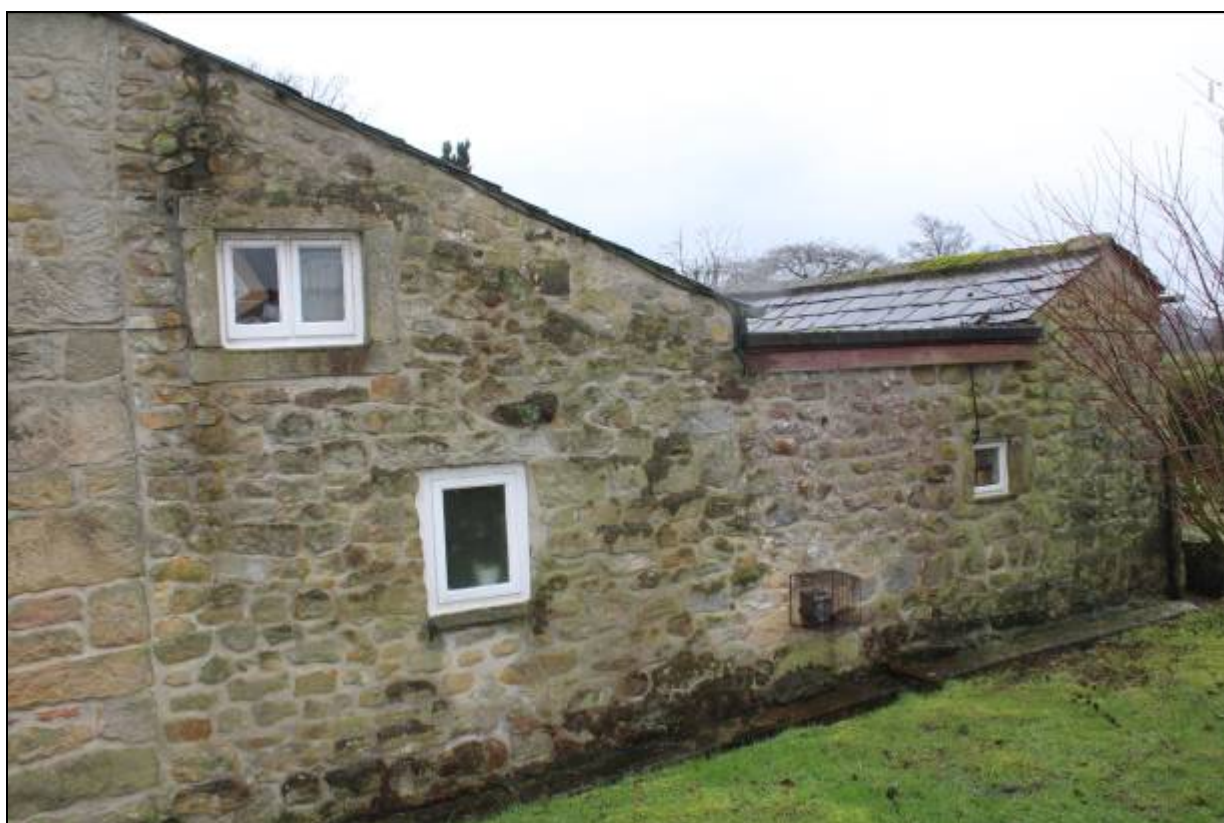
34. Rear of the outbuildings showing 1970s link between cartshed/garage (left) and garden room
