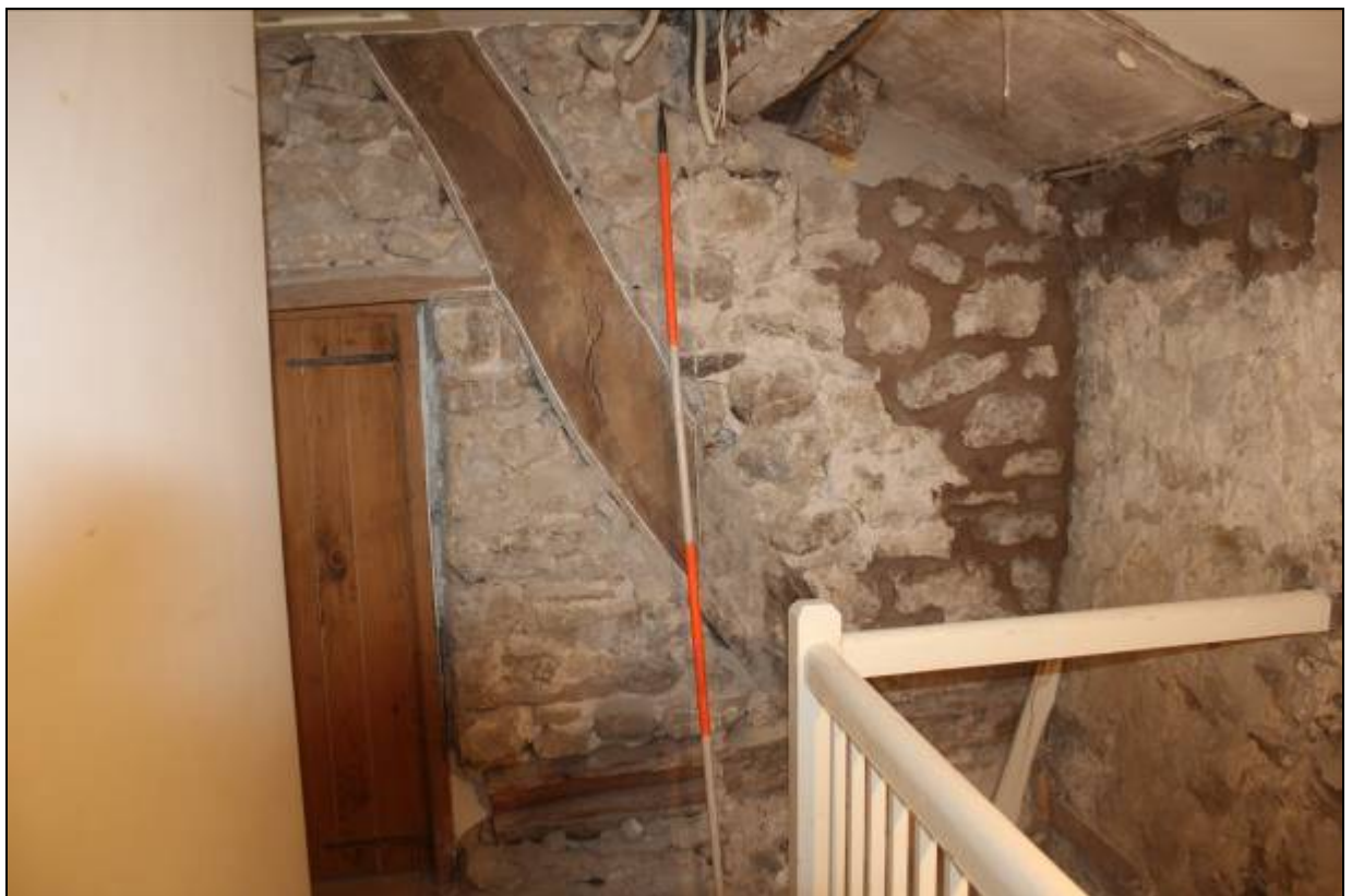
26. North blade following removal of cupboard
