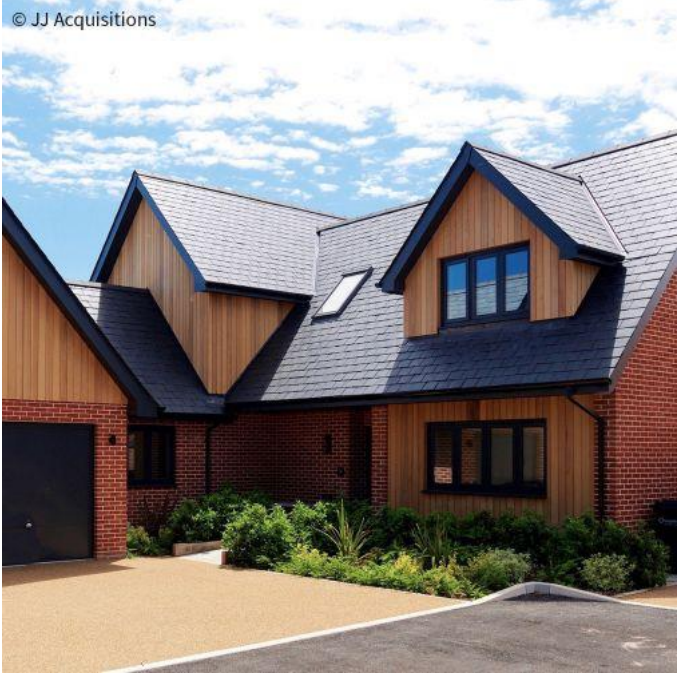
3. Roof Slates: Cupa 4 blue slate.
