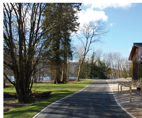
Fallbarrow Park, Windermere: Completed CellWeb TRP® Installation
