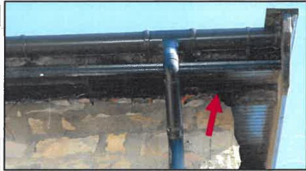
Old signs of bird nesting below soffit (lhs) and gap on south east corner (rhs)
