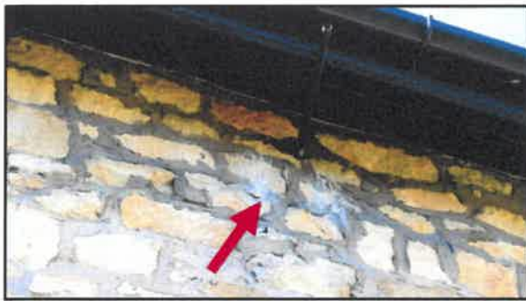
Old signs of bird nesting below soffit (lhs) and gap on south east corner (rhs)
