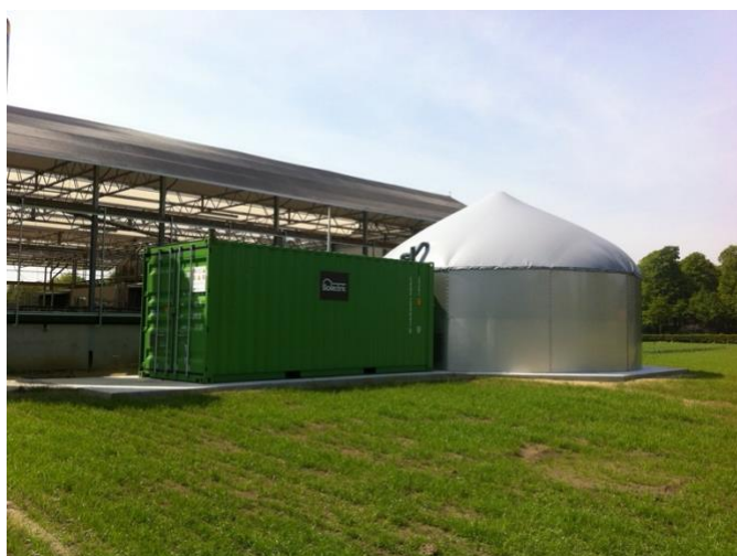
Example Bioelectric Installation
