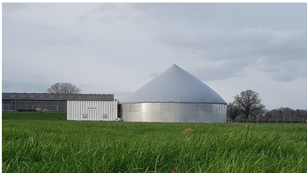
33kw small AD system in Wales
