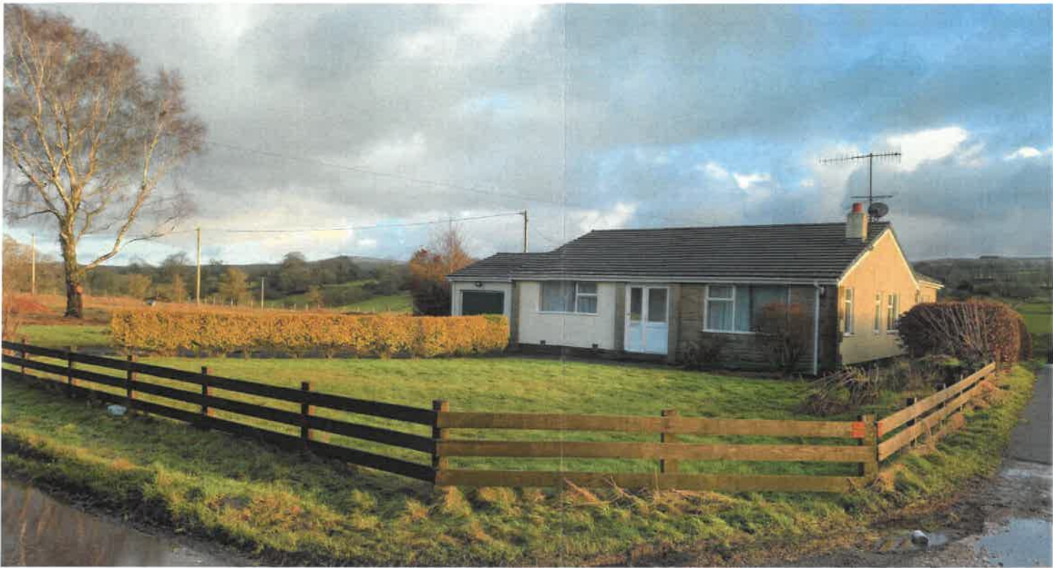
PL02: Photograph of existing bungalow taken from Rimington Lane. NTS
