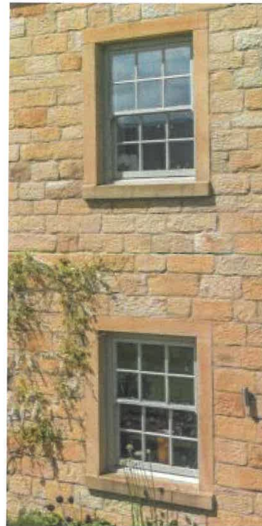
PL13: Example of traditional painted timber sliding sash windows. Boxwood House, Rimington.
