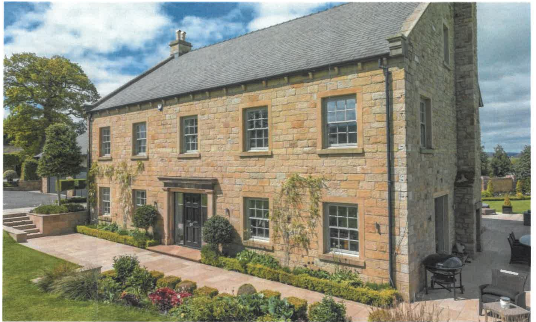
PL07: Precedent image of Georgian style architecture within the village. Boxwood House, Rimington.
