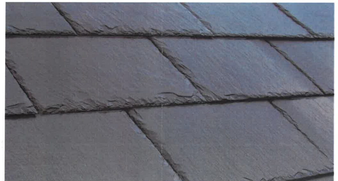
PL14: Example of Burlington natural slate roofing.
