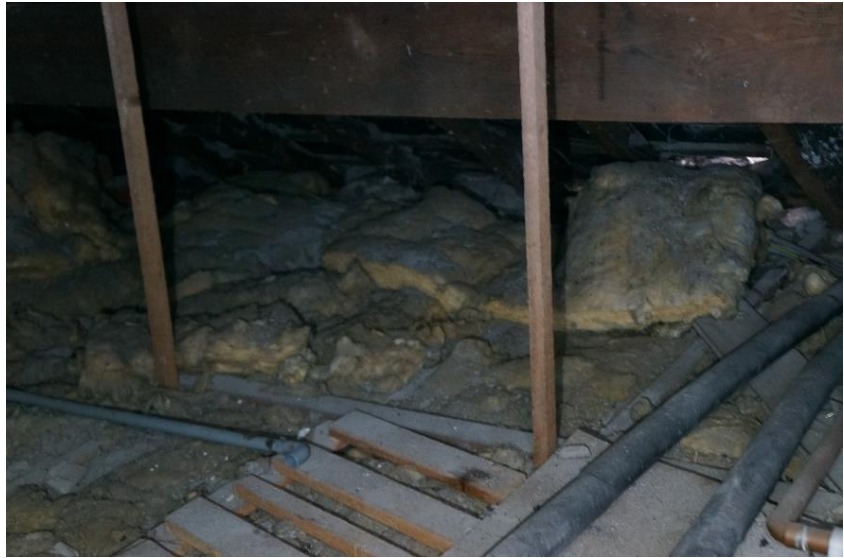
Photo 7: Insulation in the loft space covered in light grey dust from the mortar.
