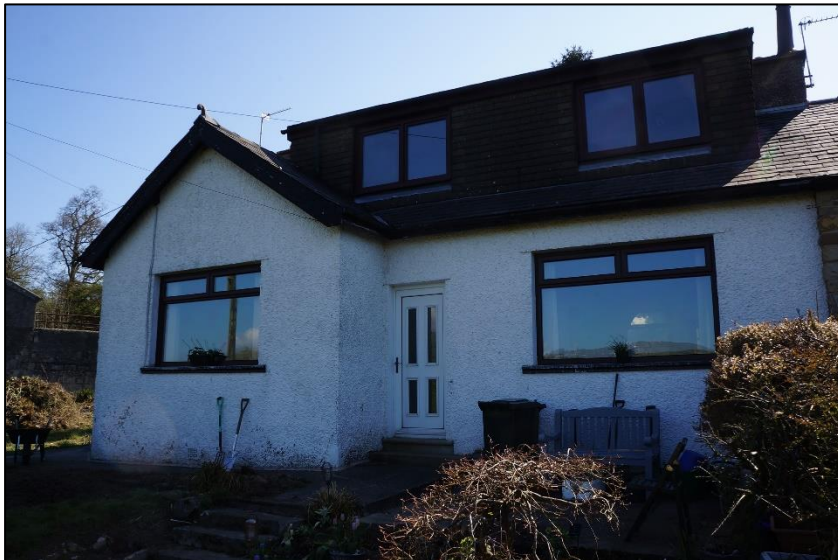
Photo 1: West elevation of house, showing flat-roofed dormer.
