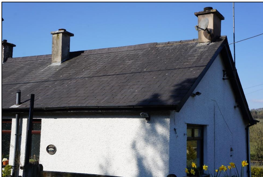
Photo 3: East and north elevations, showing the blue slate dual pitched roof.
