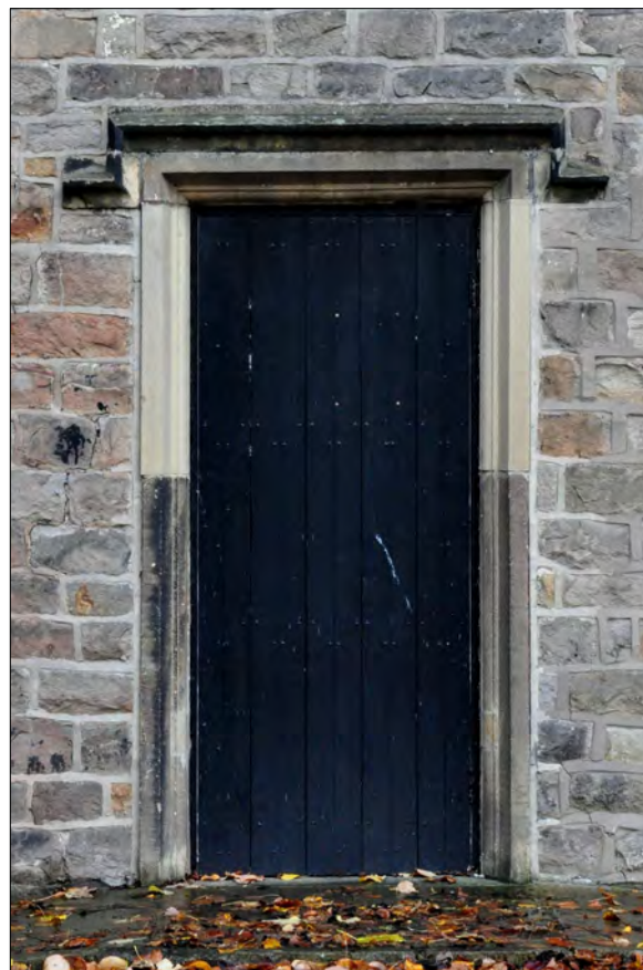
Photo 4: Former window in east elevation, proposed to be re-instated
