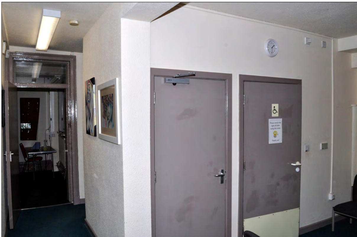
Photo 10: Modern partitions with store, proposed for platform lift
