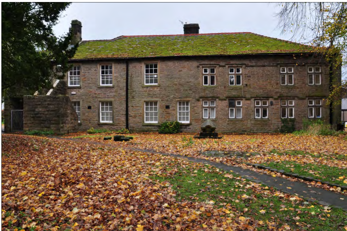
Photo 2: The south side. Original five bays of 1725 school at right
