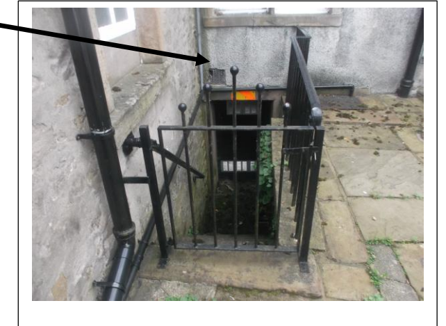
Courtyard cellar steps
