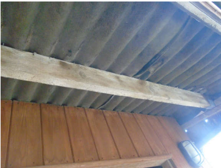
The underside of the roof overhang
