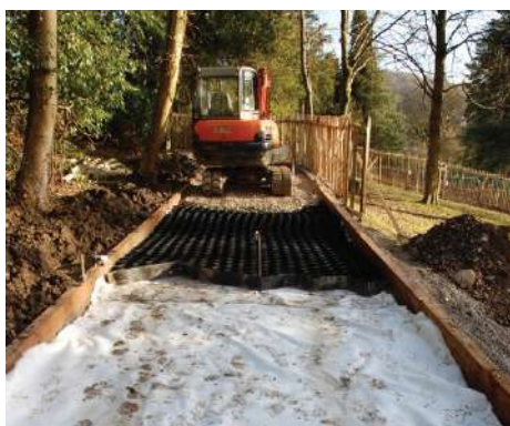
Fallbarrow Park, Windermere: CellWeb TRP® Installation
