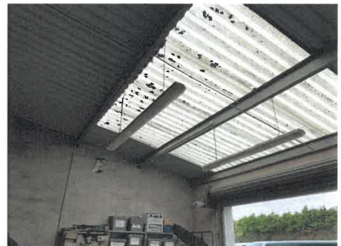
Figure 4: Workshop internal / roof
