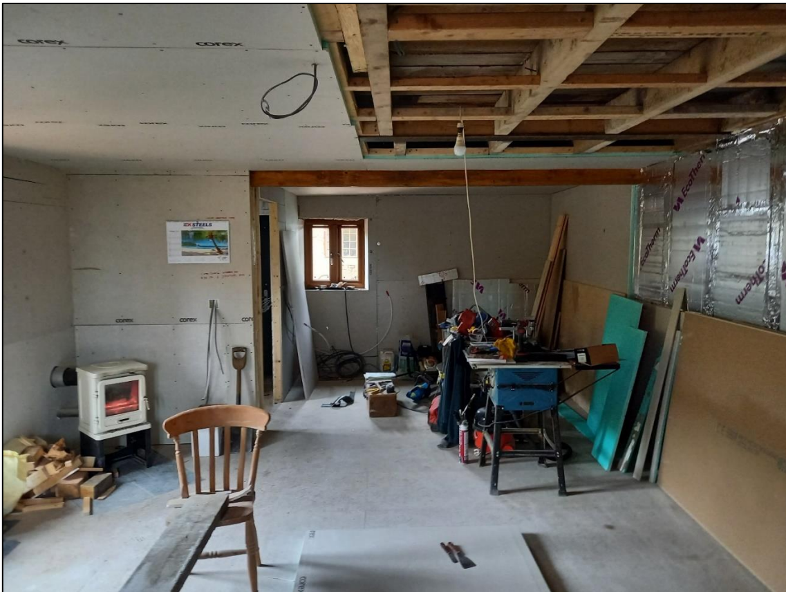
PL08: View South West at ground floor level.
