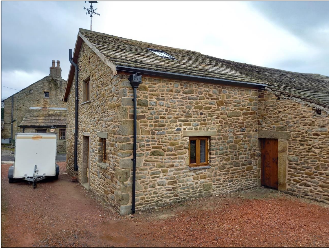
PL03: View of the barn from the north east.
