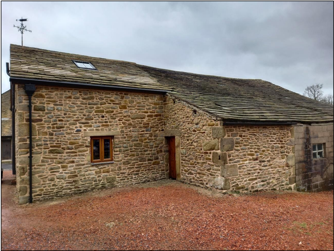
PL05: View of the north west elevation of the barn.
