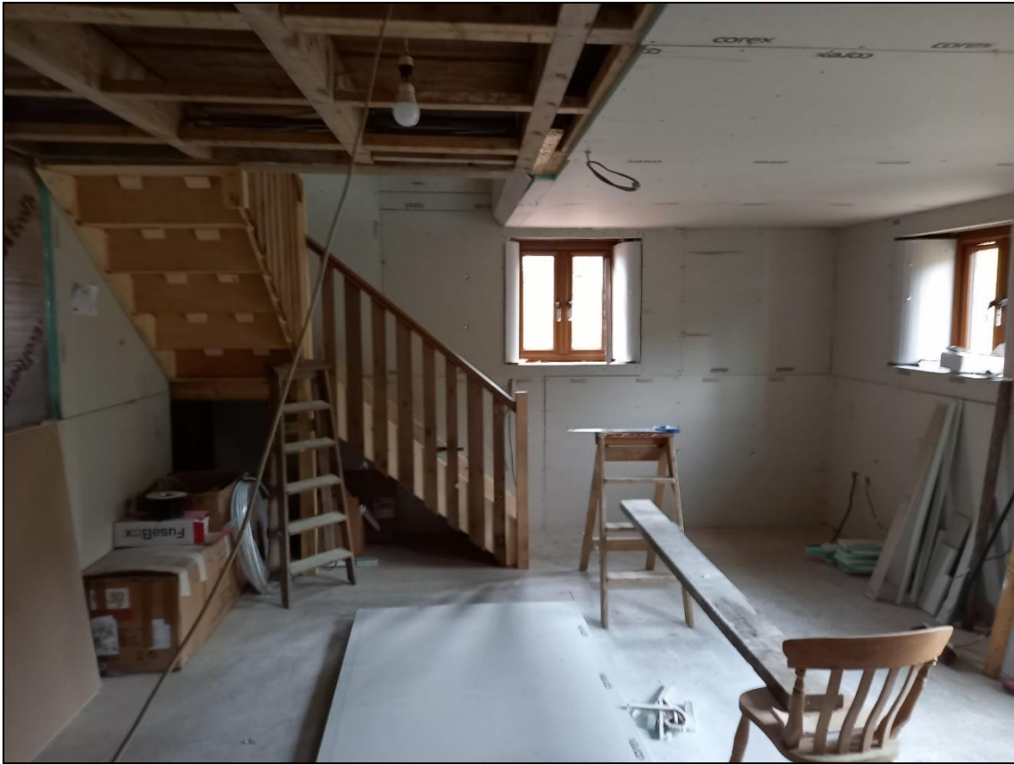
PL09: View North East at ground floor level
