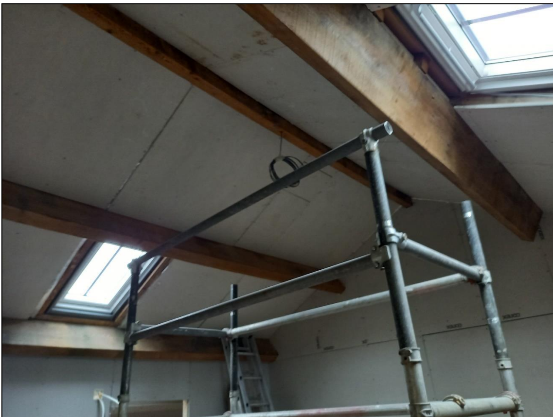
PL09: View South West at first floor
