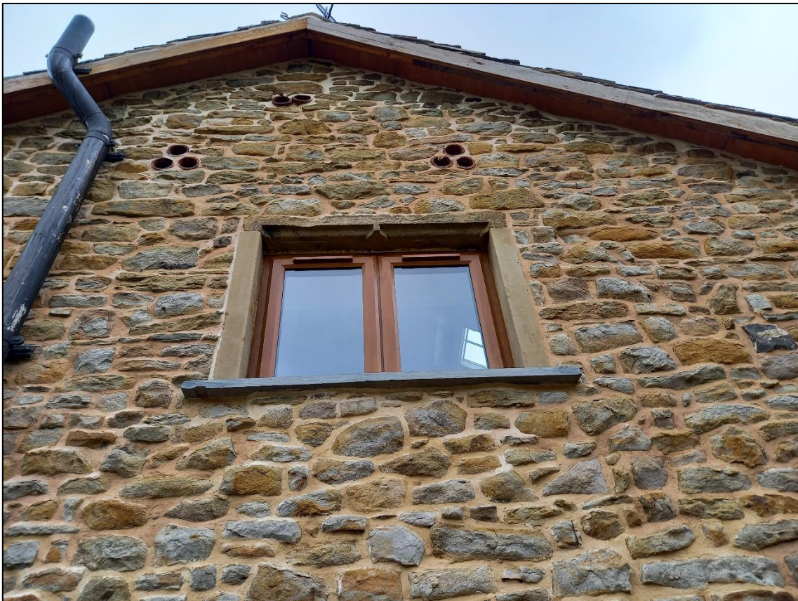
PL04: View of re-used widow head from the late 17 th / early 18 th century.
