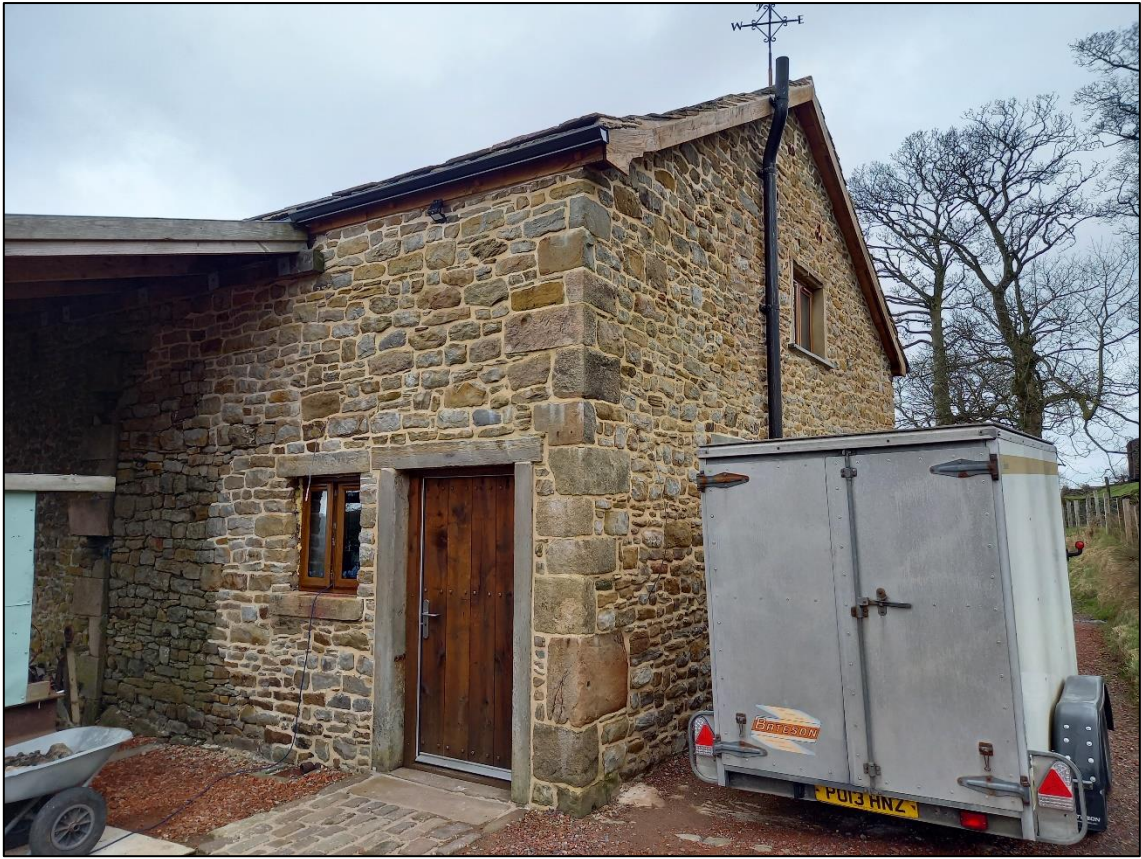
PL01: View of the Barn from the South.
