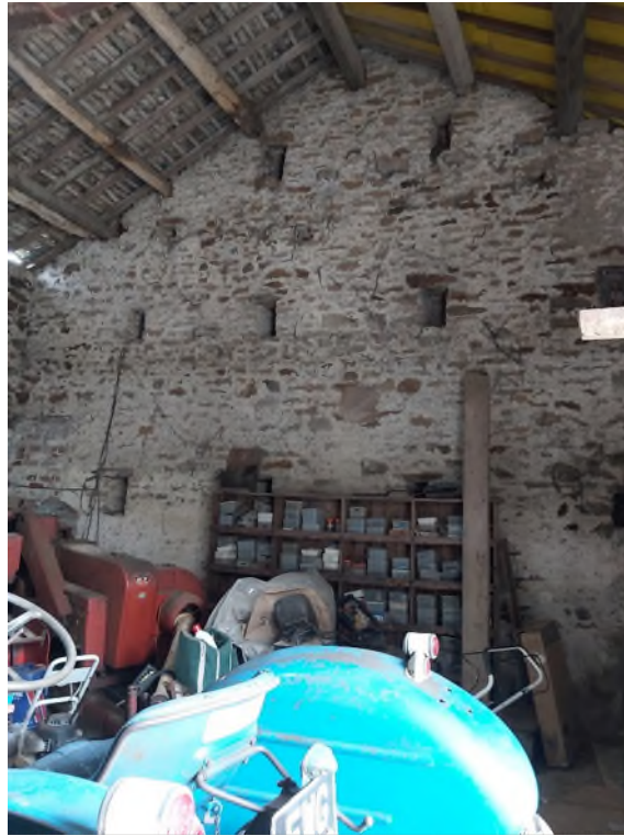
Party Wall Viewed from within main barn building
