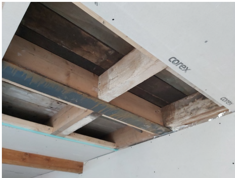
New 203x133 beam supporting existing floor joists
