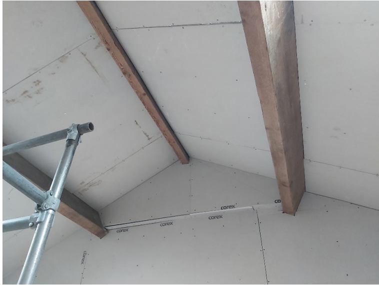
Existing Purlins & Ridge Member
