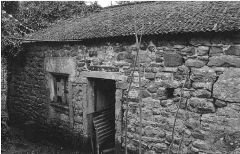
FIGURE 11: VIEW OF OUTBUILDING 2 (PIGSTY)
