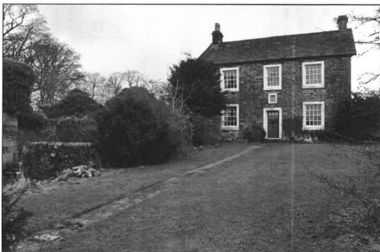
FIGURE 9: SOUTH ELEVATION OF BLACK HOUSE FARMHOUSE. OUTBUILDINGS ARE BEHIND PLANTING & TREES ON THE LEFT-HAND SIDE
