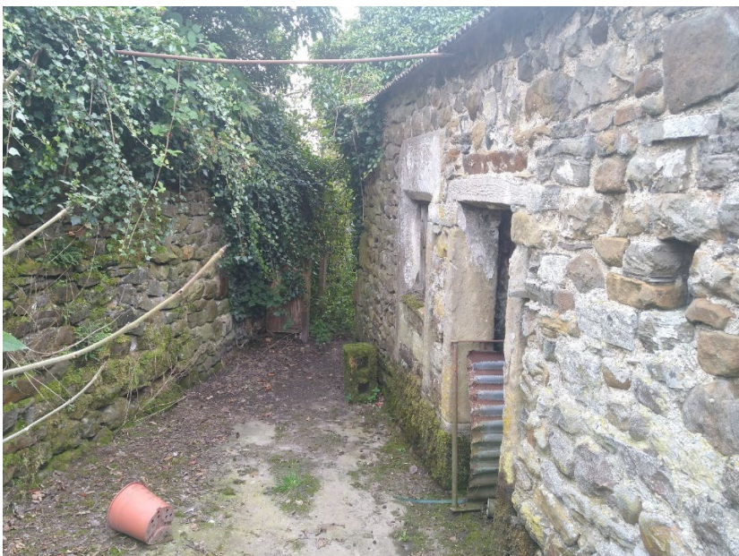
FIGURE 16: REAR OF STONE OUTBUILDING 2 (pigsty)
