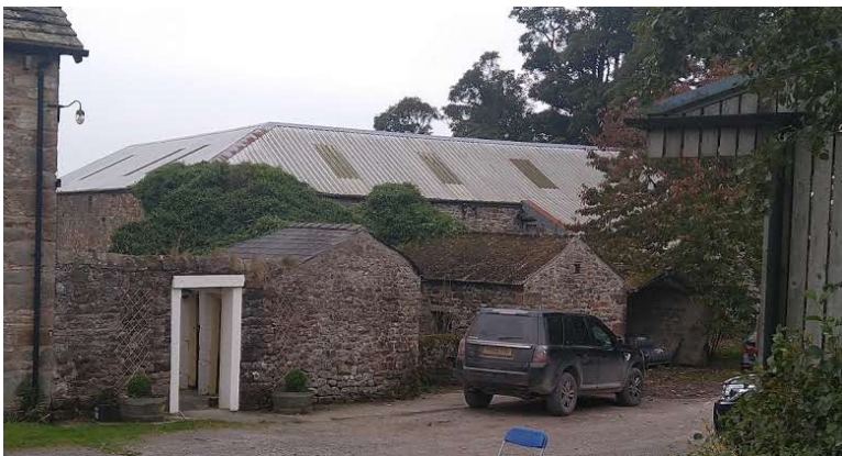
FIGURE 5: SMALL STONE OUTBUILDINGS IN THE FOREGROUND
