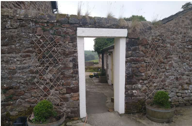
FIGURE 7: DOOR IN STONE BOUNDARY WALL LEADING TO OUTBUILDING & YARD BEHIND
