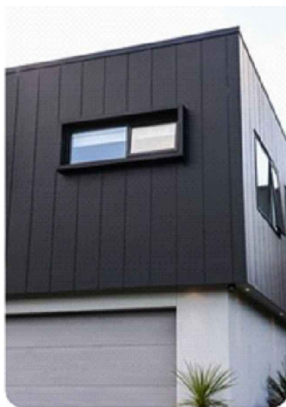
Wall cladding: Catnic - SSR2 Standing Seam Cladding - To Entrance Canopy, steel colour coated (colour tbc).
