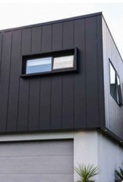
Wall cladding: Catnic - SSR2 Standing Seam Cladding - To Entrance Canopy, steel colour coated (colour tbc).
