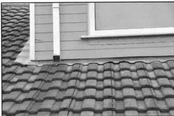
View of roof coverings below dormer (lhs) and internal view of small roof void (rhs) all areas well sealed with no gaps present
